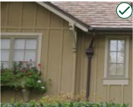
Carmel vertical board and batten siding
