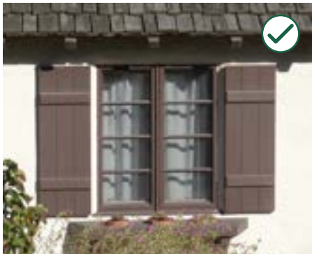
Window with shutters
