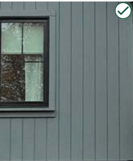
Fiber cement vertical siding
