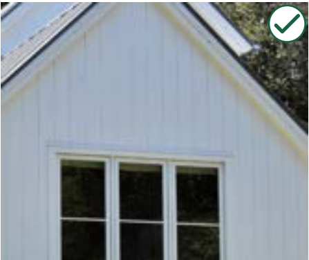
Wood vertical siding
