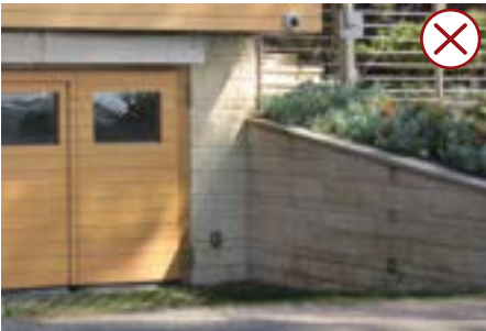
Large exposed retaining wall
