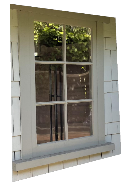
WOOD WINDOWS MATCH EXISTING WITH TRUE-DIVIDED LIGHTS
