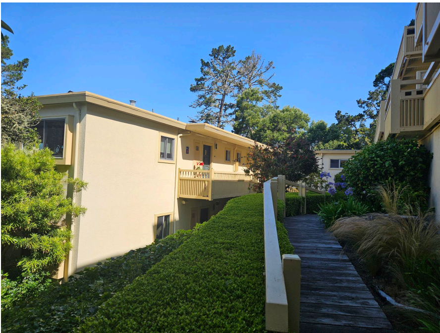
Figure 3: East elevation of Building B.
