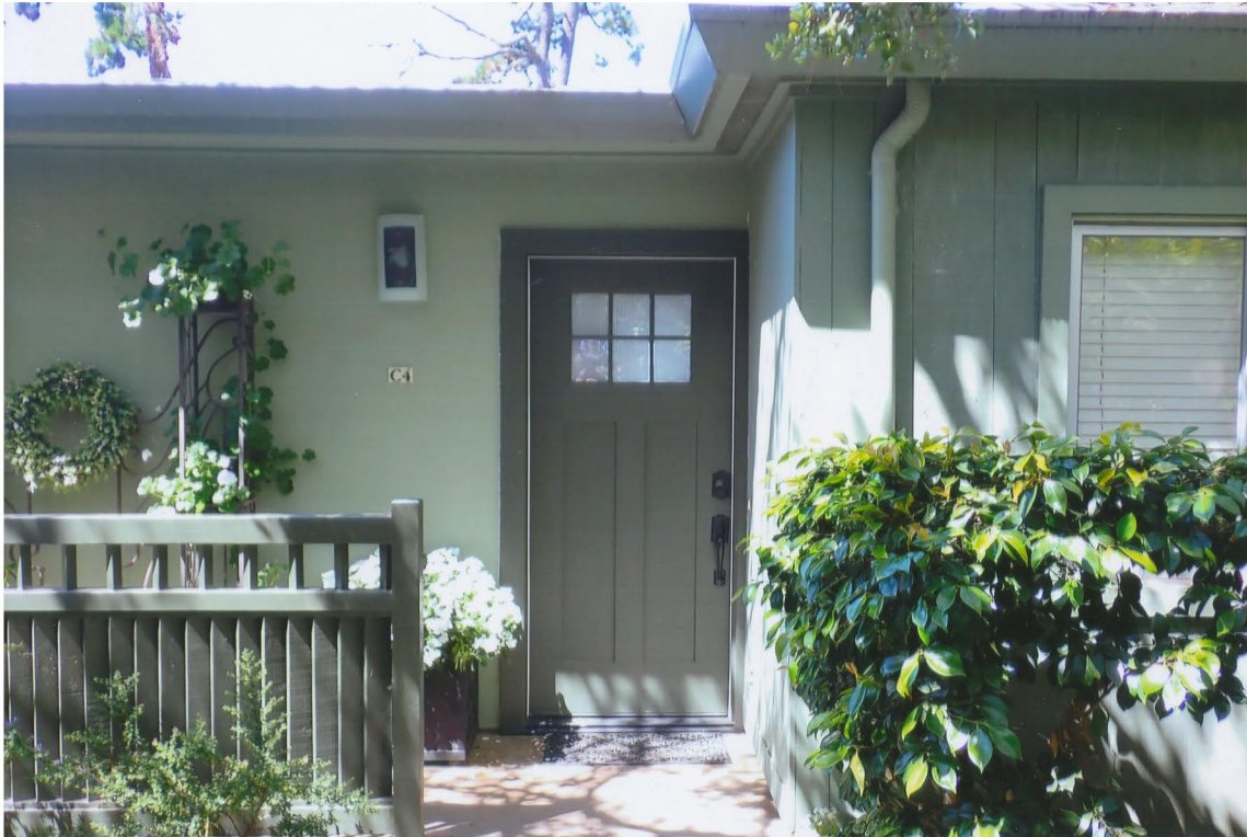
Photo #11. Looking West at Unit 4, Bldg. C, note treatment of Door & lighting fixture, Kent Seavey, Sept., 2025.
