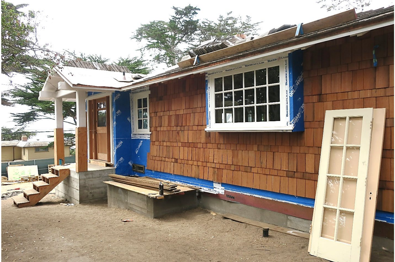
Figure 8: View of new shingles, south elevation.
