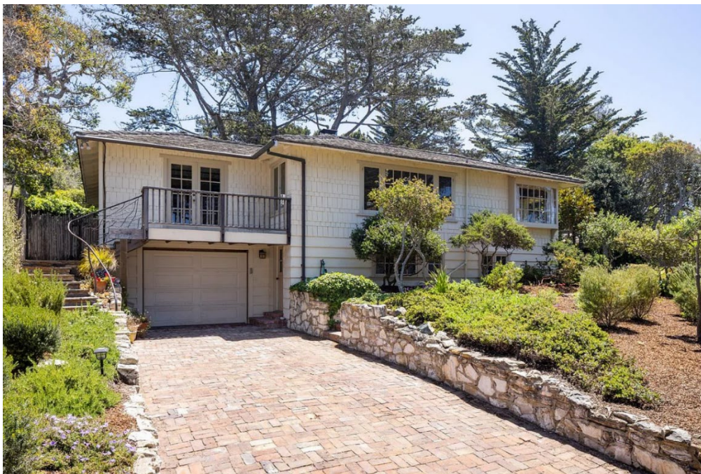
Figure 1: View of original Rockwell House, prior to construction.
