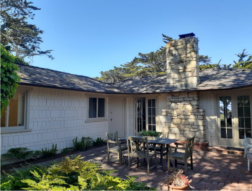
Figure 1: View of back patio, looking SW
