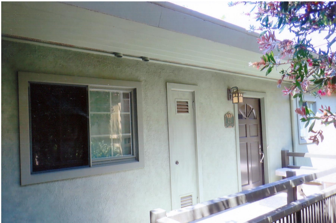
Photo #10. Looking North at entry of Unit 3, Bldg. C, note treatment of door, lighting & fenestration, K. Seavey, Sept, 2025.
