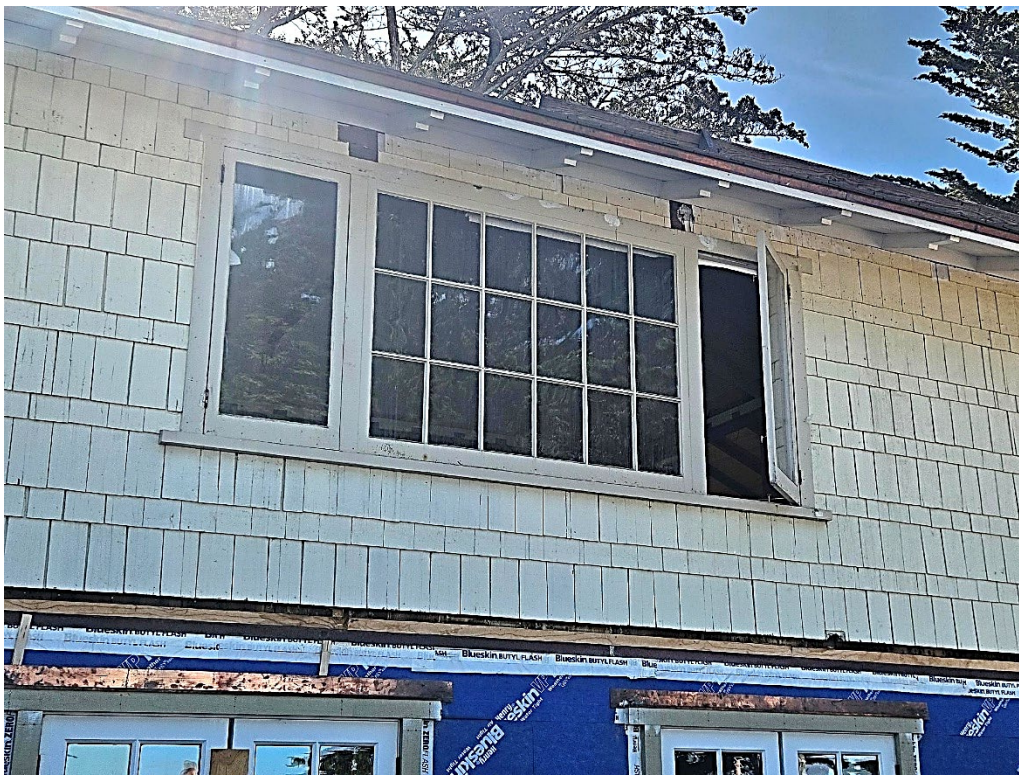
Figure 3: Detail of the one remaining original window on the front elevation.
