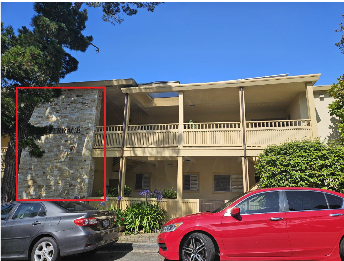
Figure 10: View of altered wall, east elevation Building A.
