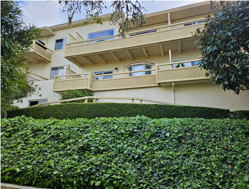
Figure 2: West elevation of Building A.
