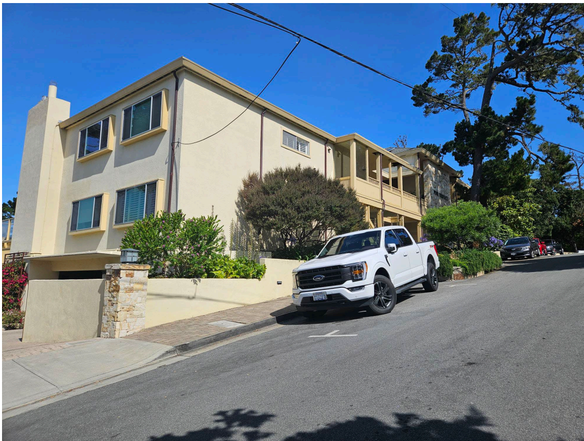
Figure 1: Building A looking northwest with view of “boxed” windows.
