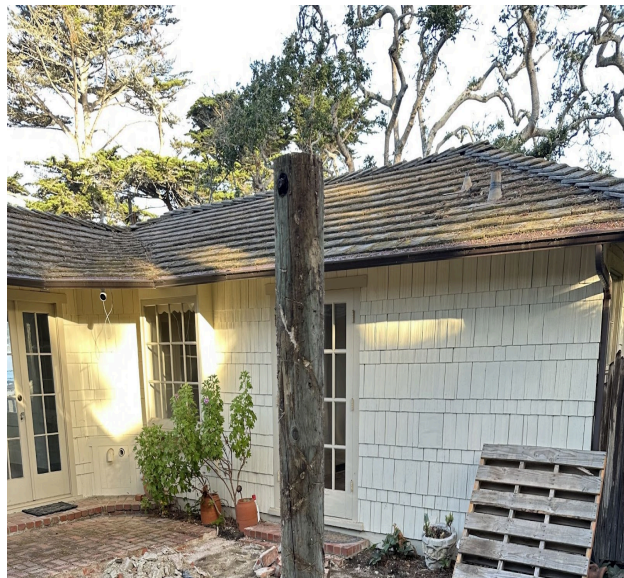
Original Synthetic Roof (Pic#2)
