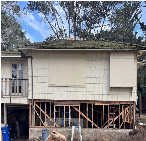
Original Synthetic Roof (Pic #1)
