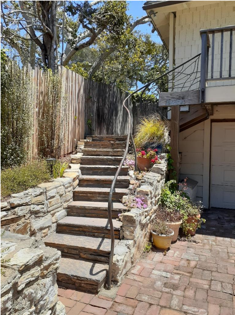
Figure 7: View of rock stairs added in 1960 and decorative railing added in 2002.
