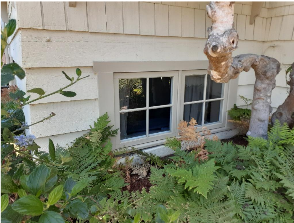
Figure 4: Basement windows on south elevation
