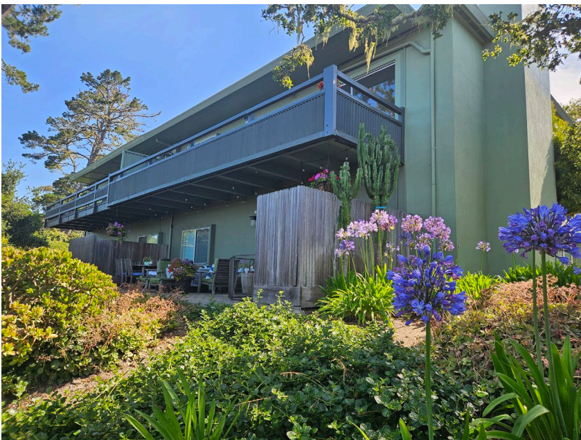
Figure 5: Rear elevation of Building C.
