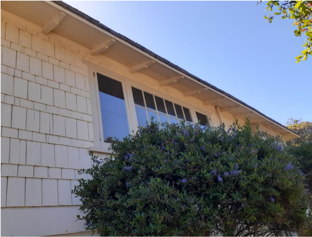
Figure 5: View of extended lintels and sills and decorative notched rafters
