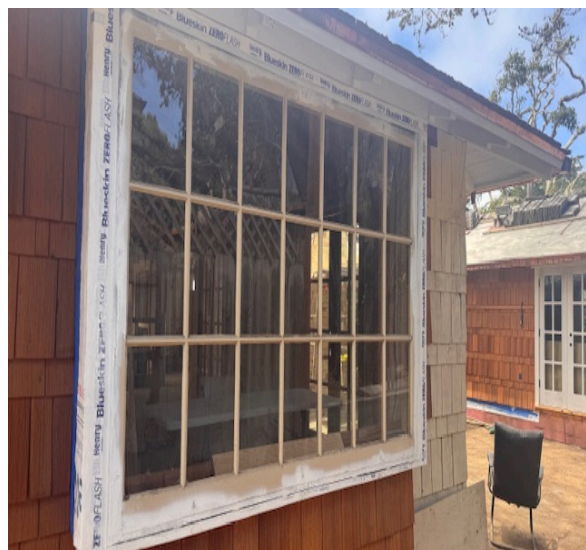
Existing Window Nook
