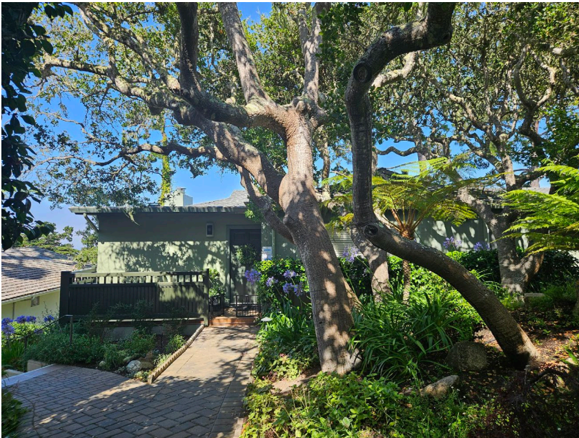
Figure 4: Front elevation of Building C.
