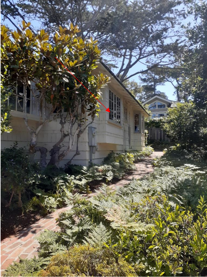
Figure 3: Arrow indicates location of new entrance.
