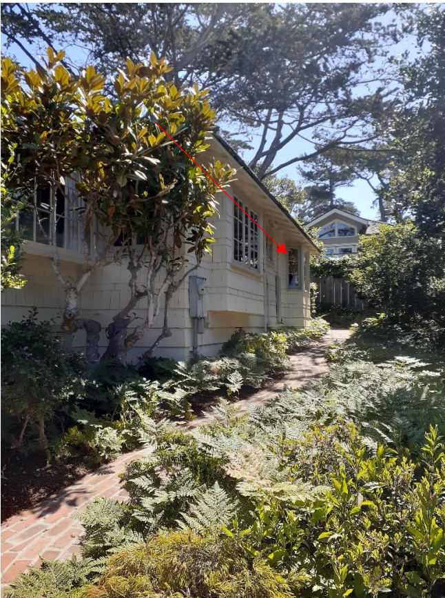
Figure 2: View NE of south elevation with added bay window, indicated with red arrow
