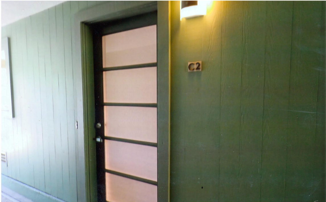
Photo #9. Looking SW at entry of Unit 2, Bldg. C, note flush wood veneer over stucco wall, Kent Seavey, Sept., 2025.
