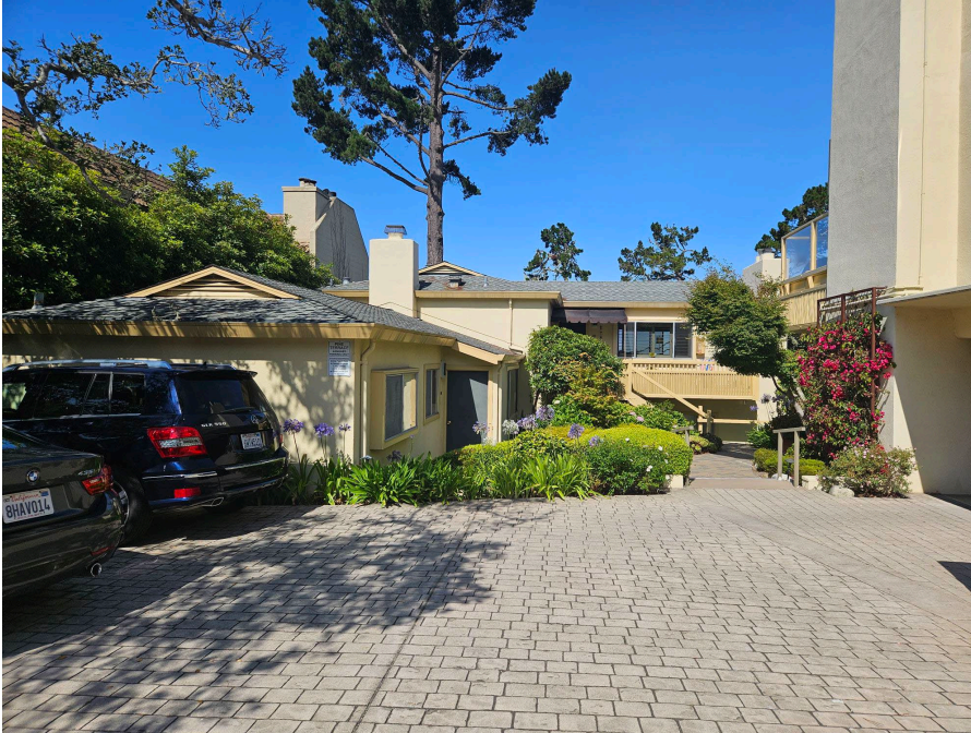
Figure 6: View of Building D from Mission St.
