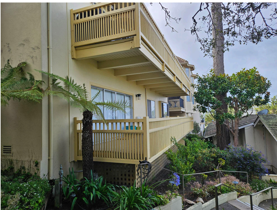
Figure 7: View of Building D balconies, south elevation.
