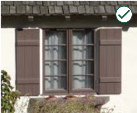
Window with shutters
