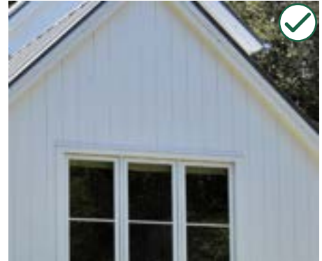
Wood vertical siding
