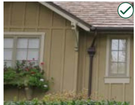
Carmel vertical board and batten siding
