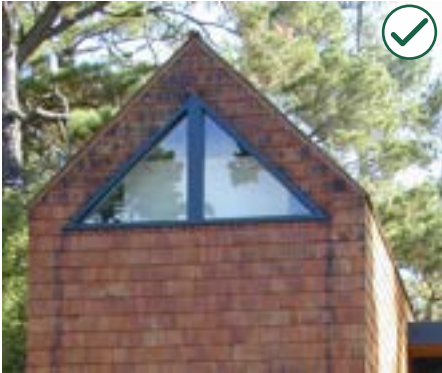
Wood shingle siding
