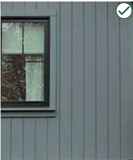
Fiber cement vertical siding
