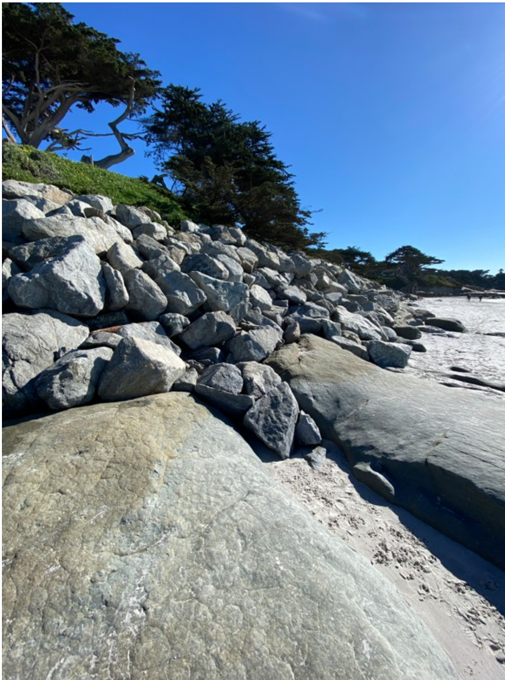
Photograph 53: Profile View of Revetment R3 on January 30, 2023
