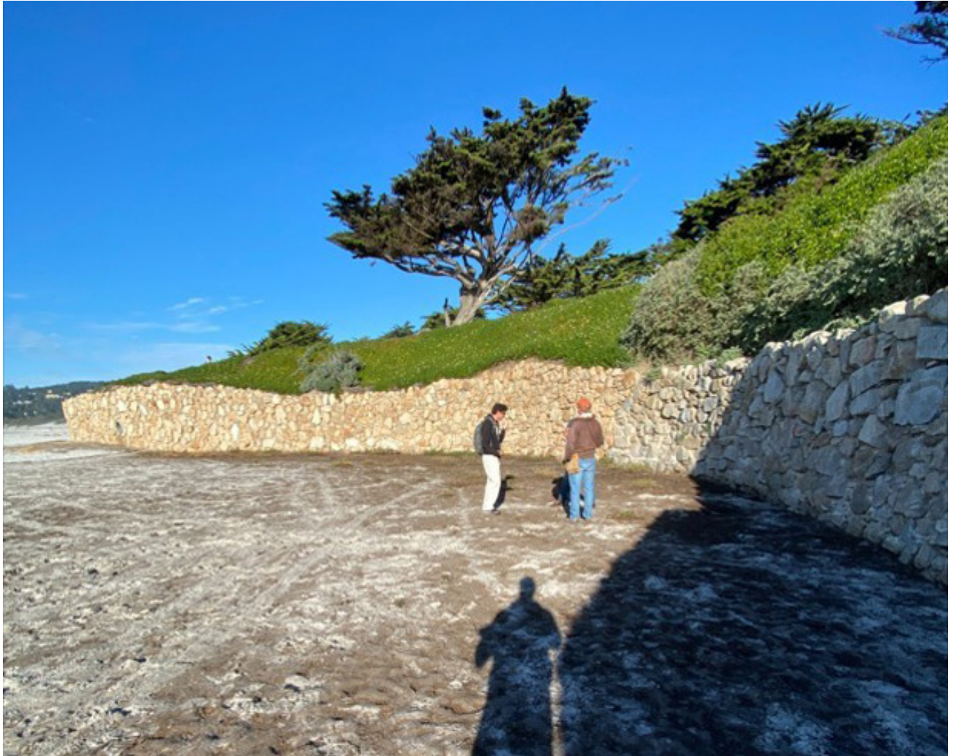
Photograph 25: Looking North at Seawall S3 on December 22, 2022
