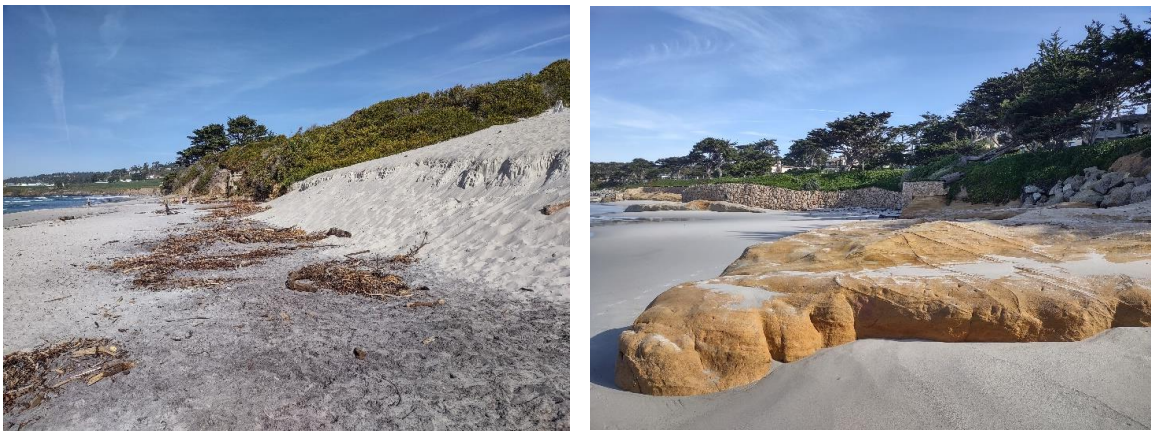
Figure 22. In response to winter storms (seen here in 2023), it is common for the steep sand dunes around Del Mar Avenue to scarp on the seaward edge (left), and for scouring to expose the underlying base of sandstone outcroppings (right) and footings of the coastal armoring in the southern areas of the beach.
