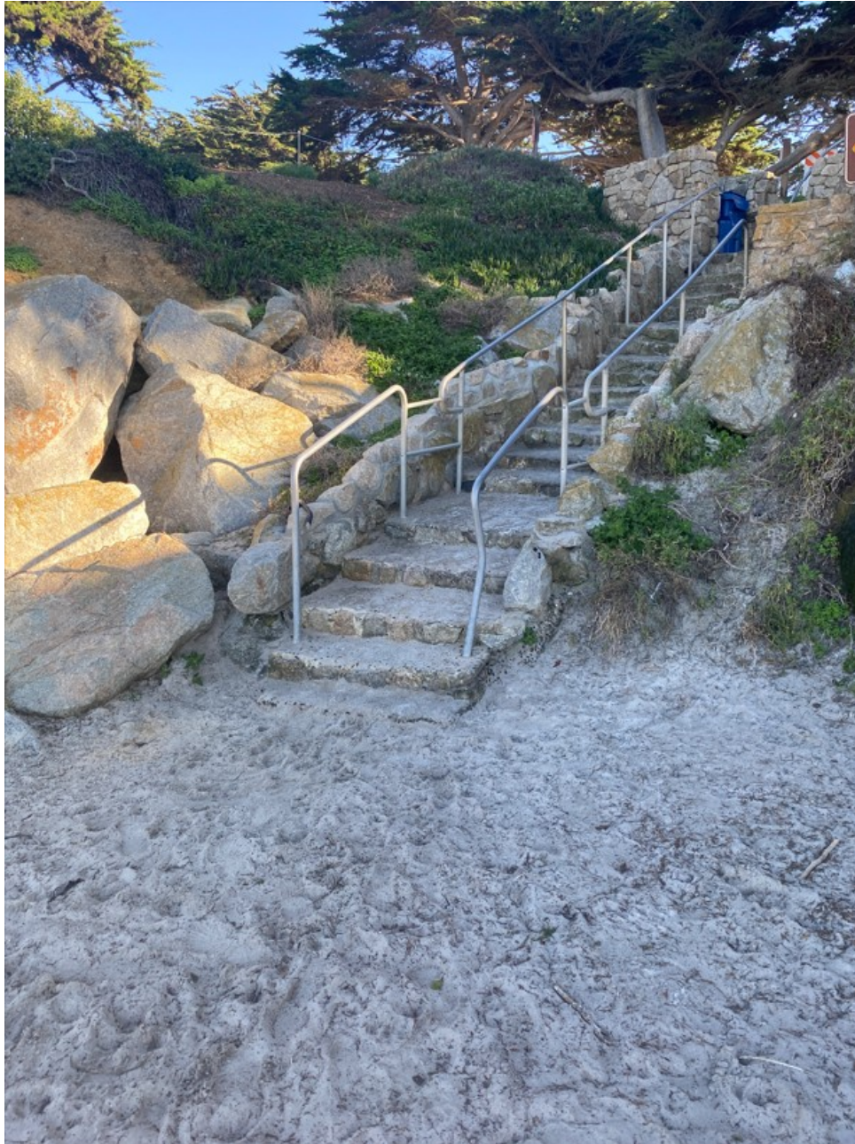
Photograph 14: Public Access Stairway ST2 on December 22, 2022
