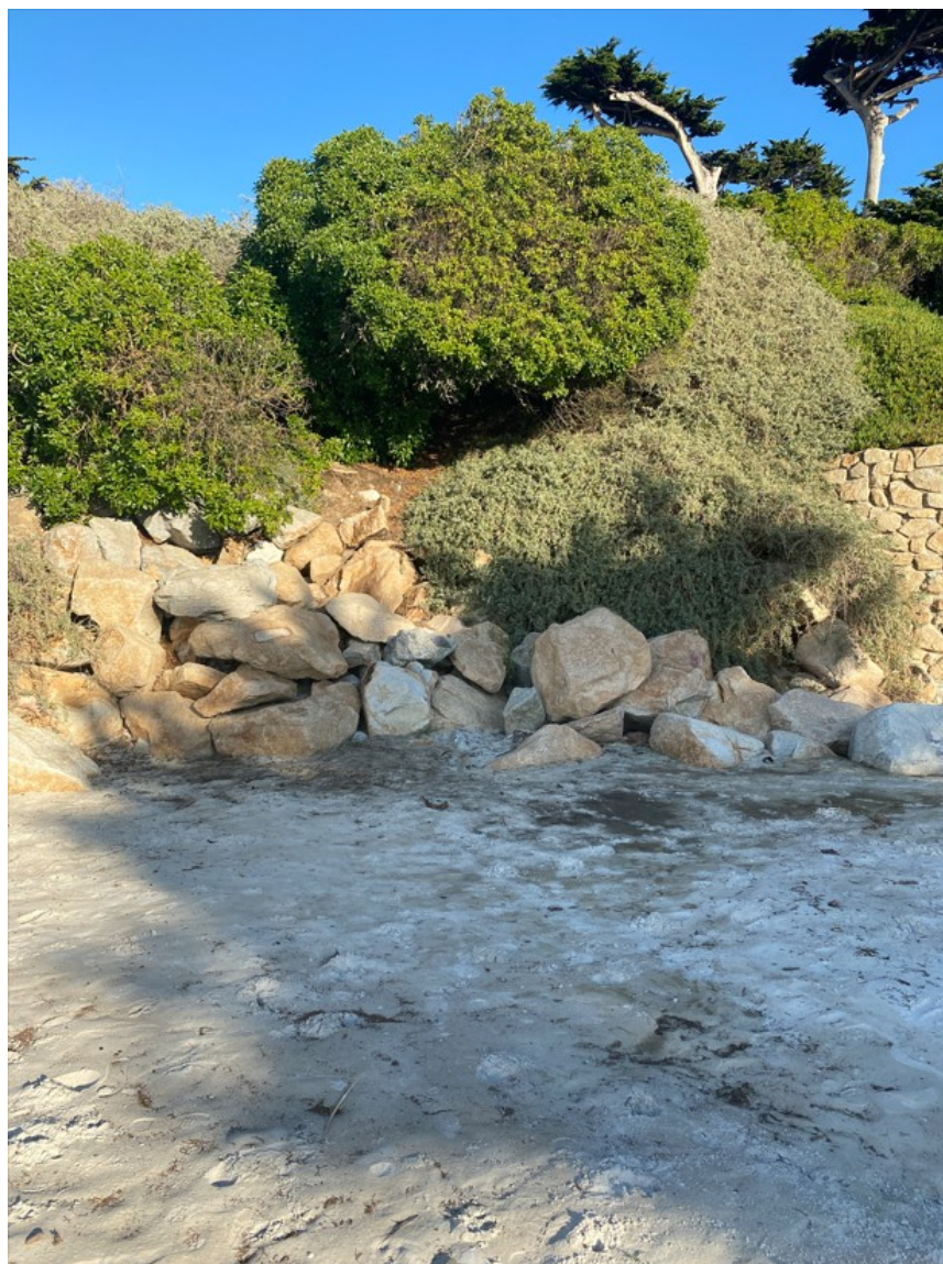
Photograph 33: Showing South End of Revetment R2 on December 22, 2022
