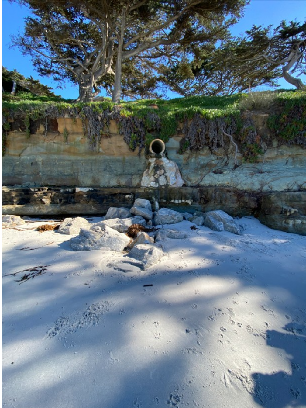
Photograph 44: Storm Drain Outfall with Minor Armoring Between ST4 and R3 on January 30, 2023
