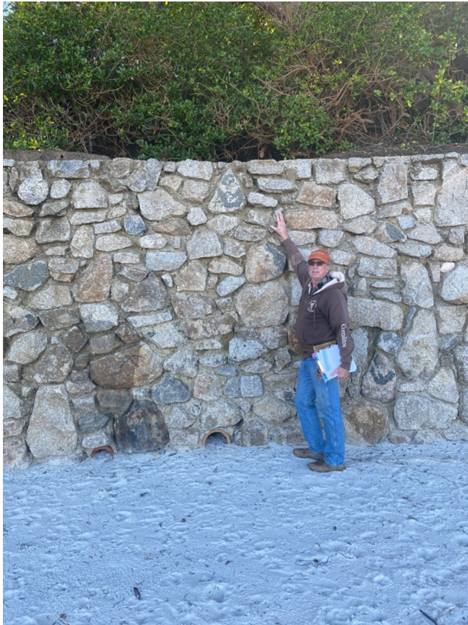
Photograph 9: Seawall S2 on December 22, 2022
