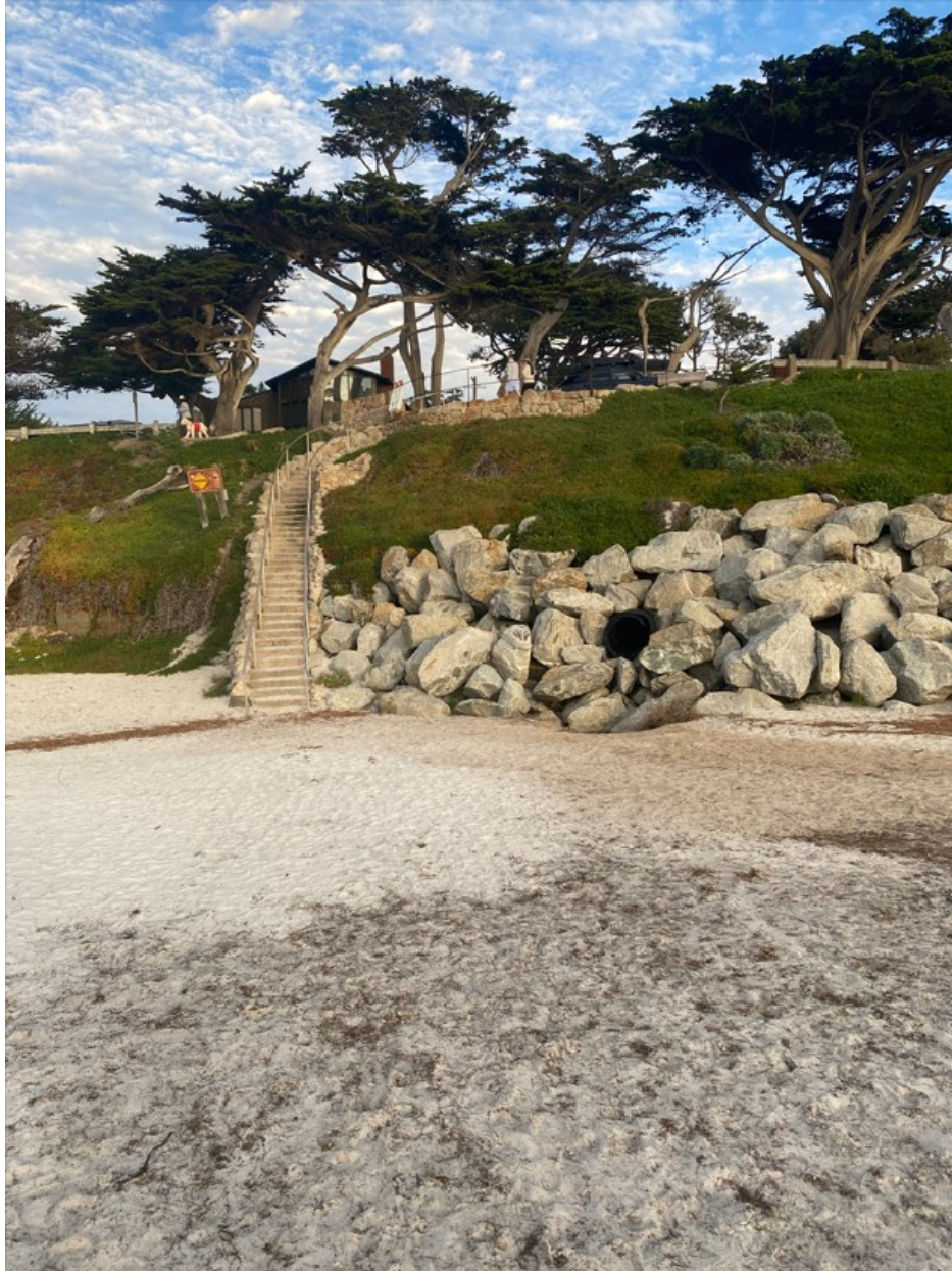
Photograph 58: Showing Stairway ST5 and North End of Revetment R6 on December 22, 2023
