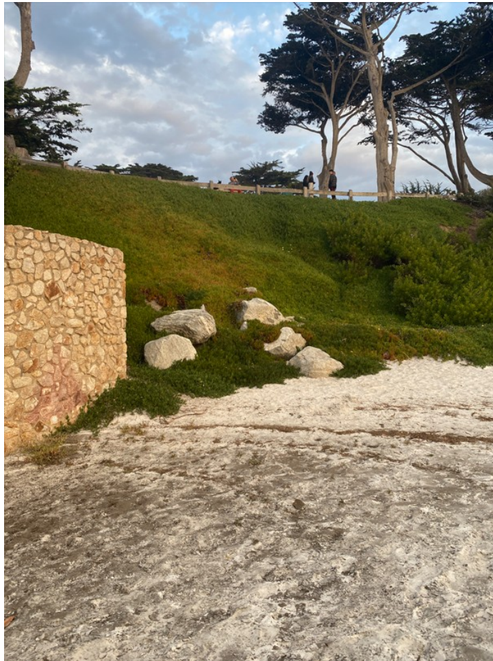
Photograph 63: Showing Few Boulders Exposed at the North End of Revetment R4 On December 22, 2022
