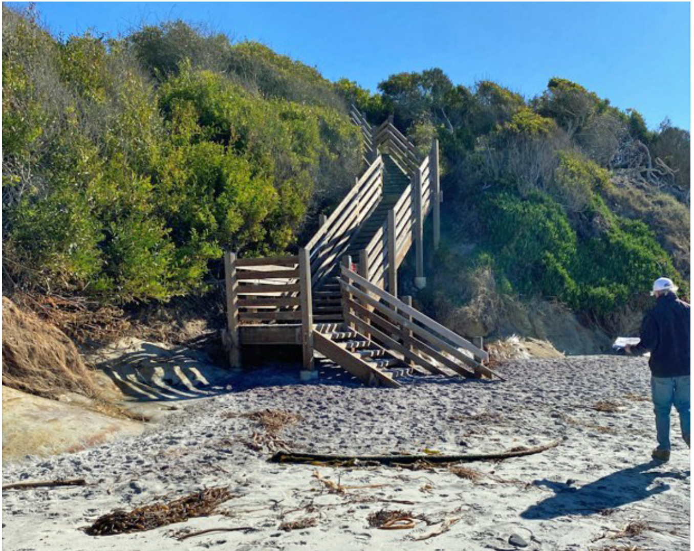
Photograph 96: Stairway ST11 on January 30, 2023
