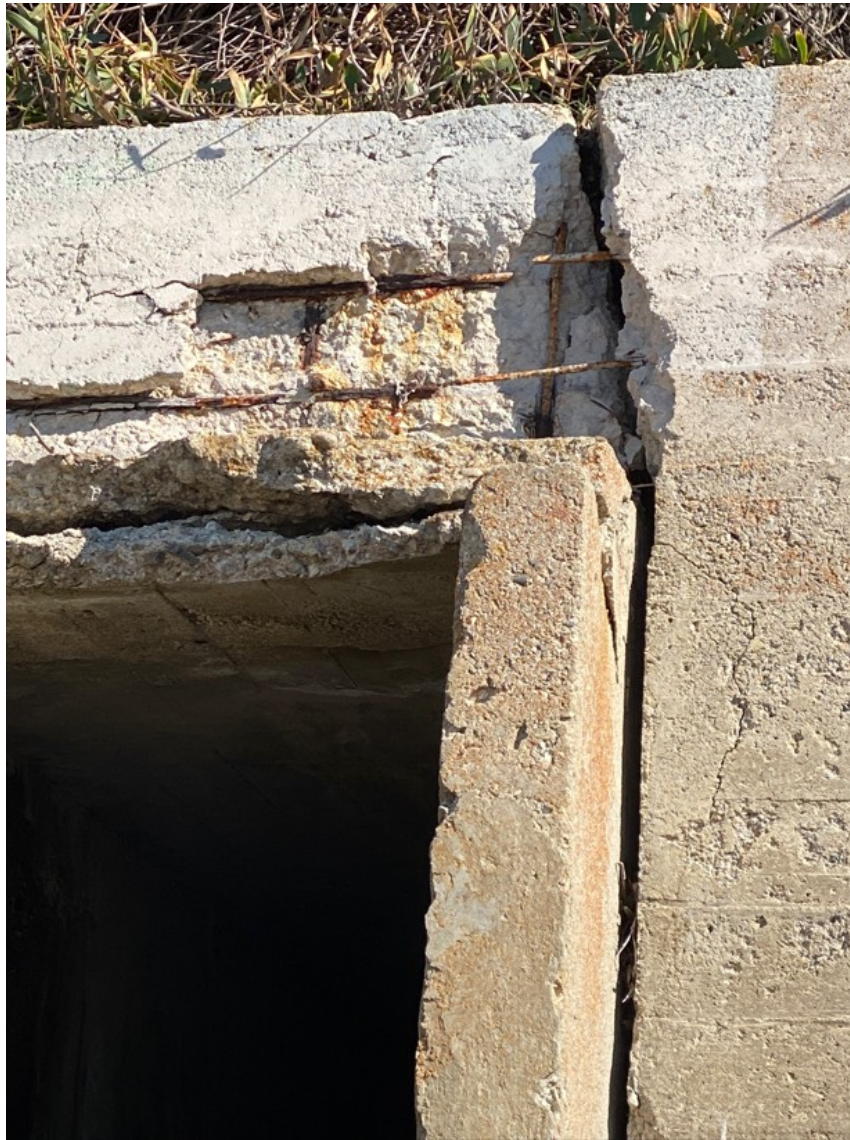
Photograph 95: Seawall S10 on January 30, 2023
