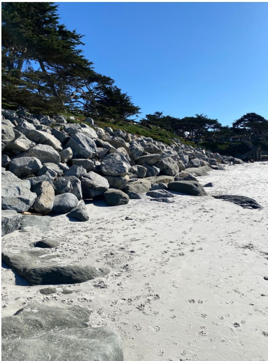
Photograph 51: Showing the Middle Portion of Revetment R3 on January 30, 2023
