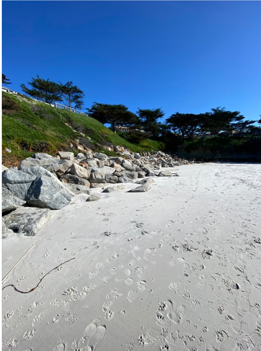
Photograph 49: Showing Revetment R3 Looking South on January 30, 2023
