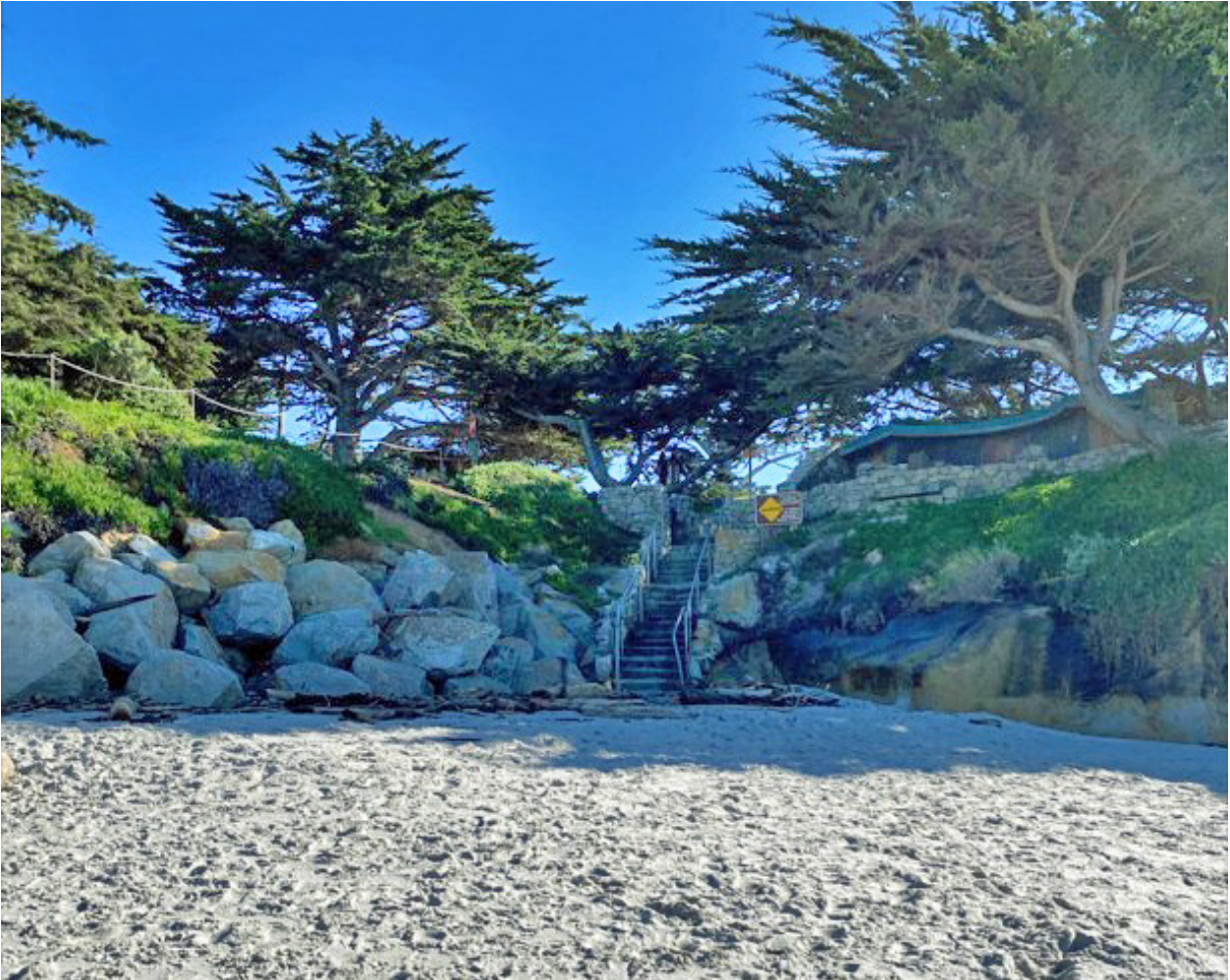
Photograph 15: Showing Revetment R1 and Stairway ST2 on January 30, 2023
