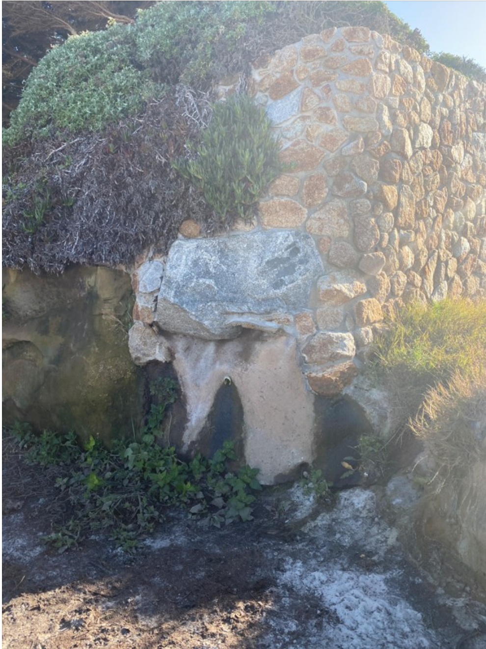
Photograph 13: North End of Seawall S2 on December 22, 2022
