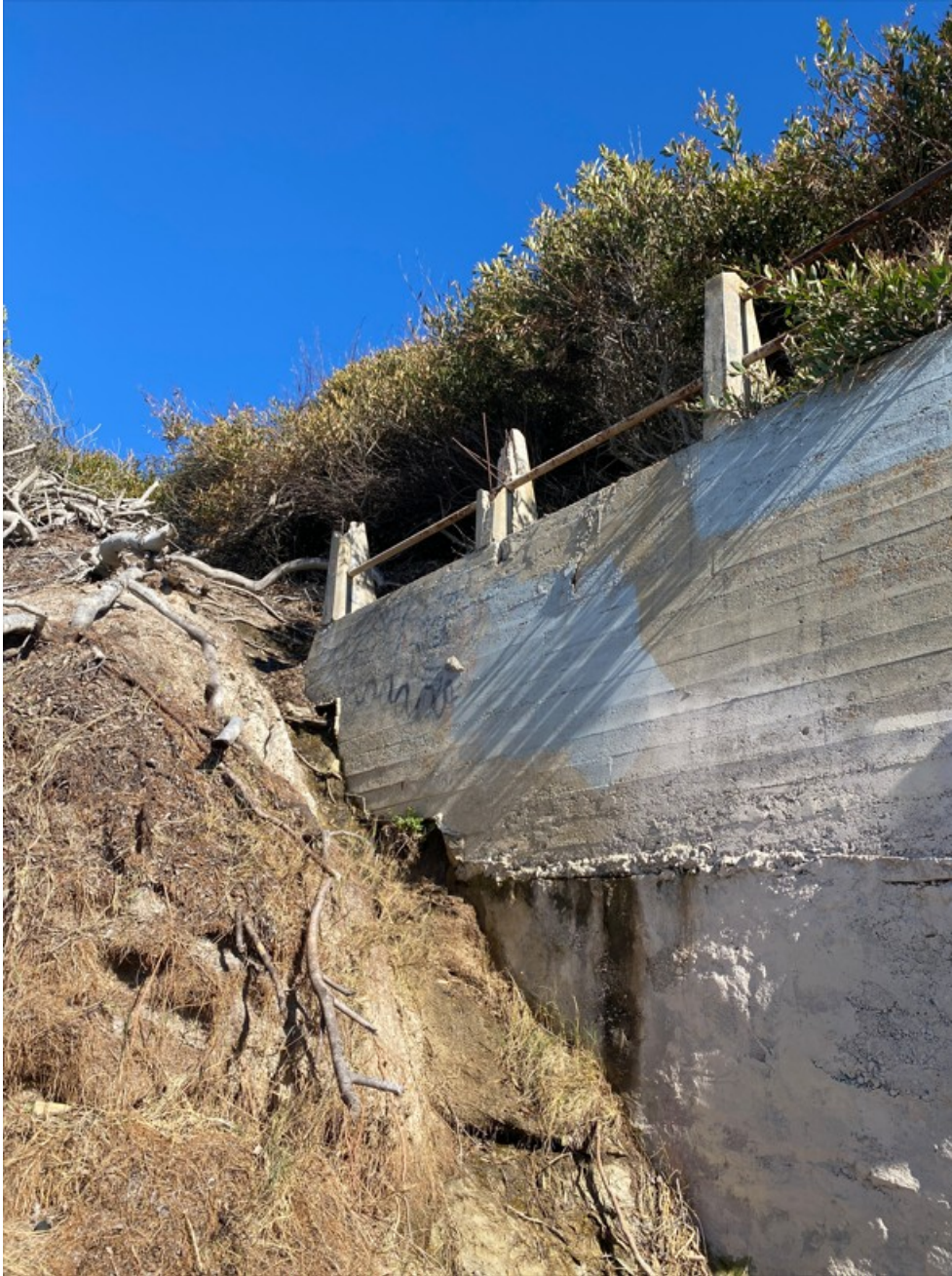
Photograph 94: Seawall S10 on January 30, 2023
