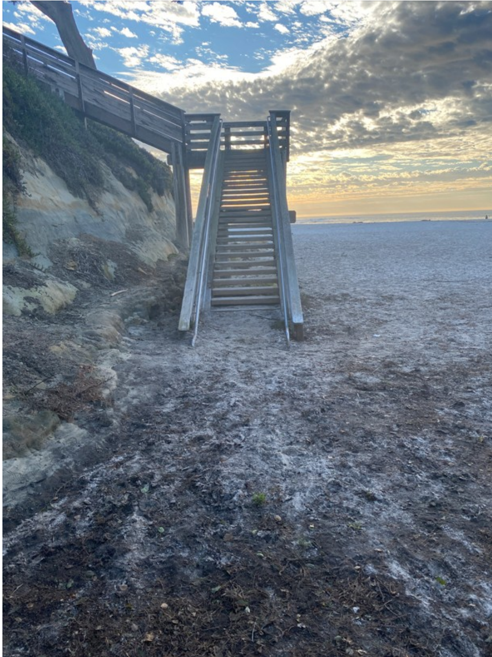
Photograph 40: Showing Base of Stairway ST4 naturally buried in beach sand on December 22, 2022
