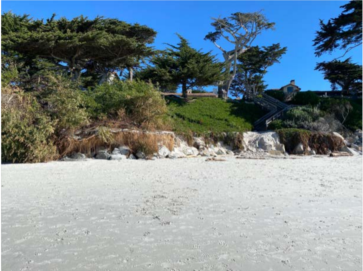
Photograph 80: Showing South End of Central Portion of Revetment R5 on January 30, 2023
