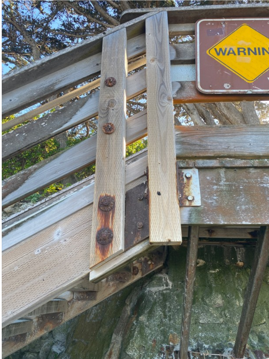
Photograph 5: Public Access Stairway ST1 on December 22, 2022
