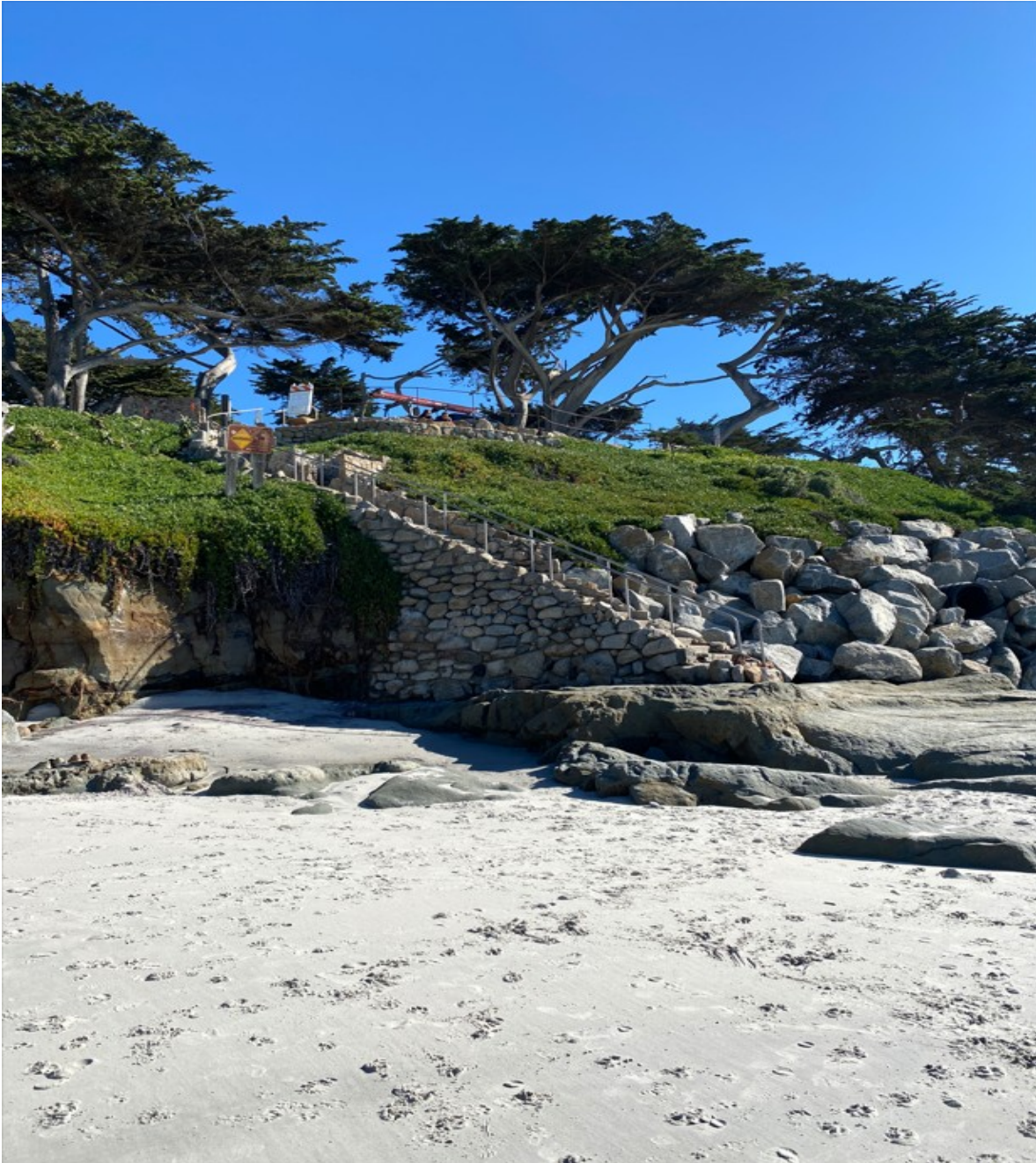
Photograph 56: Showing Stairway ST5 on January 30, 2023
