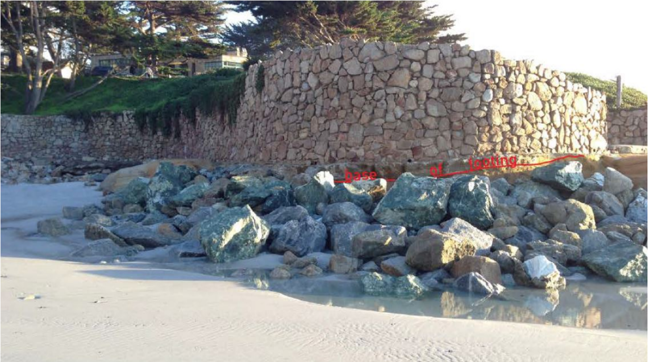
Photograph 29: Seawall S3 Just North of ST4 in February 2016 (Easton Geology)
