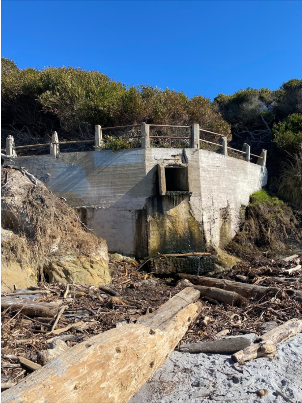
Photograph 92: Seawall S10 on January 30, 2023
