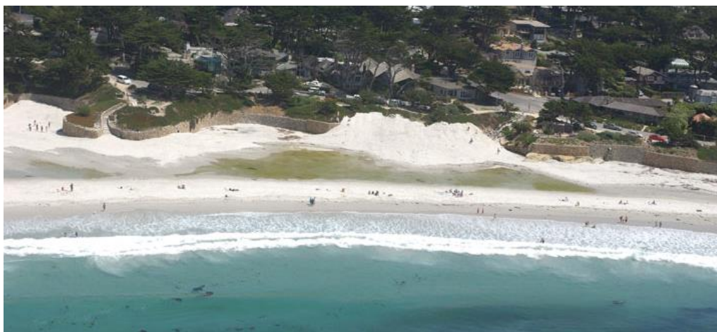
Figure 17. Beach management with sand bulldozed over the riprap revetments near 13th Avenue Source: Coastal Records Project (August 2003).
