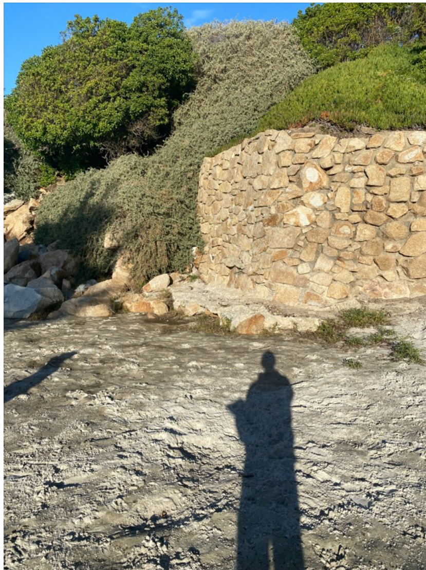
Photograph 32: North End of Seawall S3 on December 22, 2022
