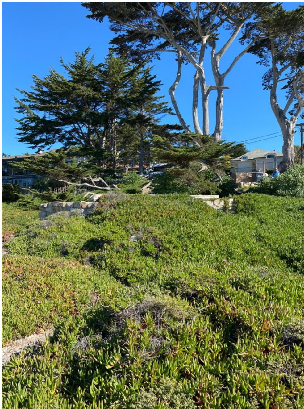
Photograph 88: Seawall S8 on January 30, 2023
