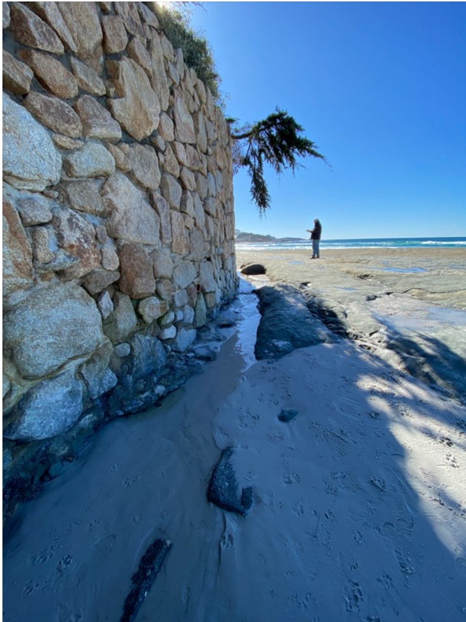
Photograph 70: Seawall S7 Foundation on January 30, 2023
