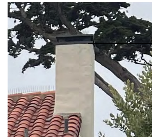
EXISTING CHIMNEY CAP ON MAIN RESIDENCE
