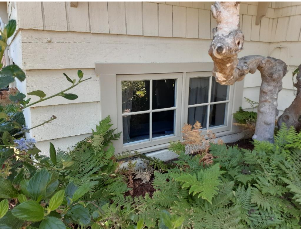
Figure 4: Basement windows on south elevation
