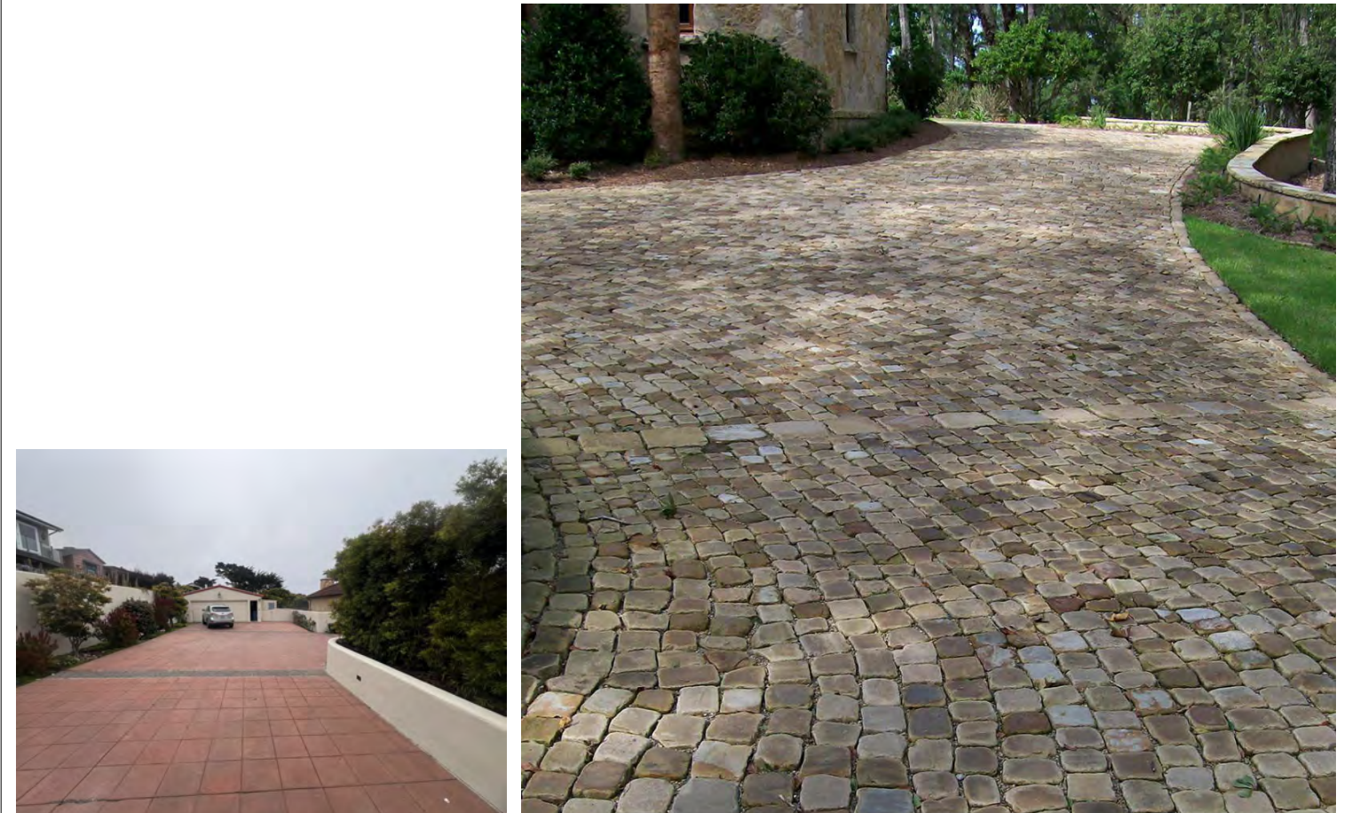
EXISTING STAMPED CONCRETE
