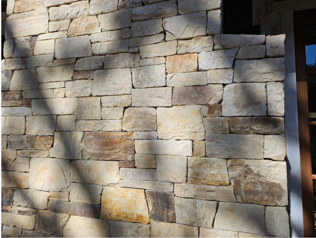
Figure 6: Detail of new chimney.
