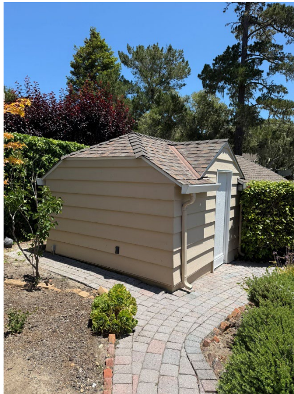
Back and south side of garage
