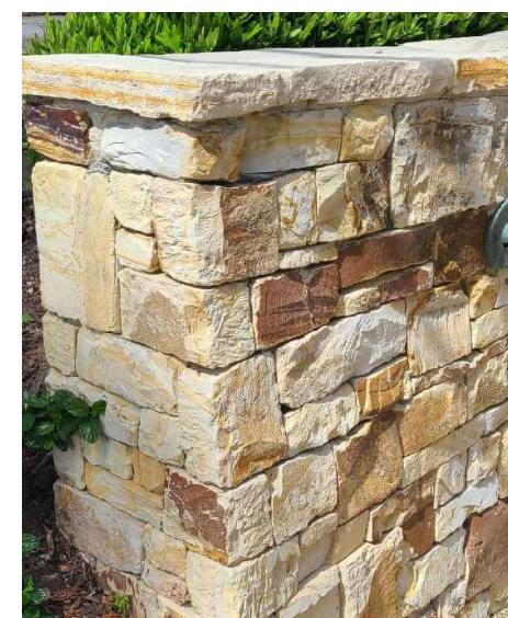
NEW STONE AT ENTRY COLUMN / GARAGE
