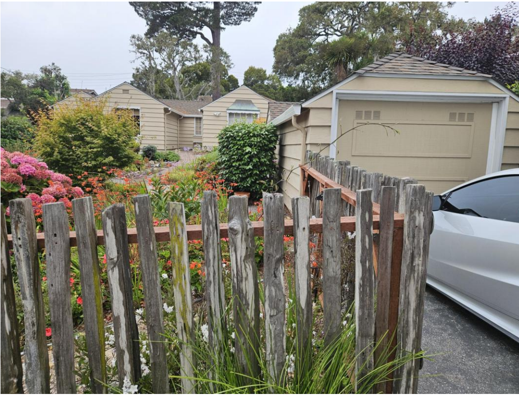
Figure 5: View of Unit House and garage from Torres Street.
