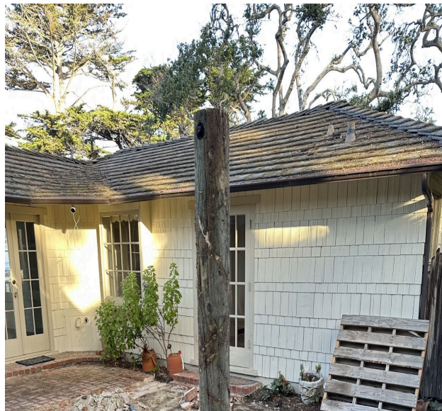
Original Synthetic Roof (Pic#2)
