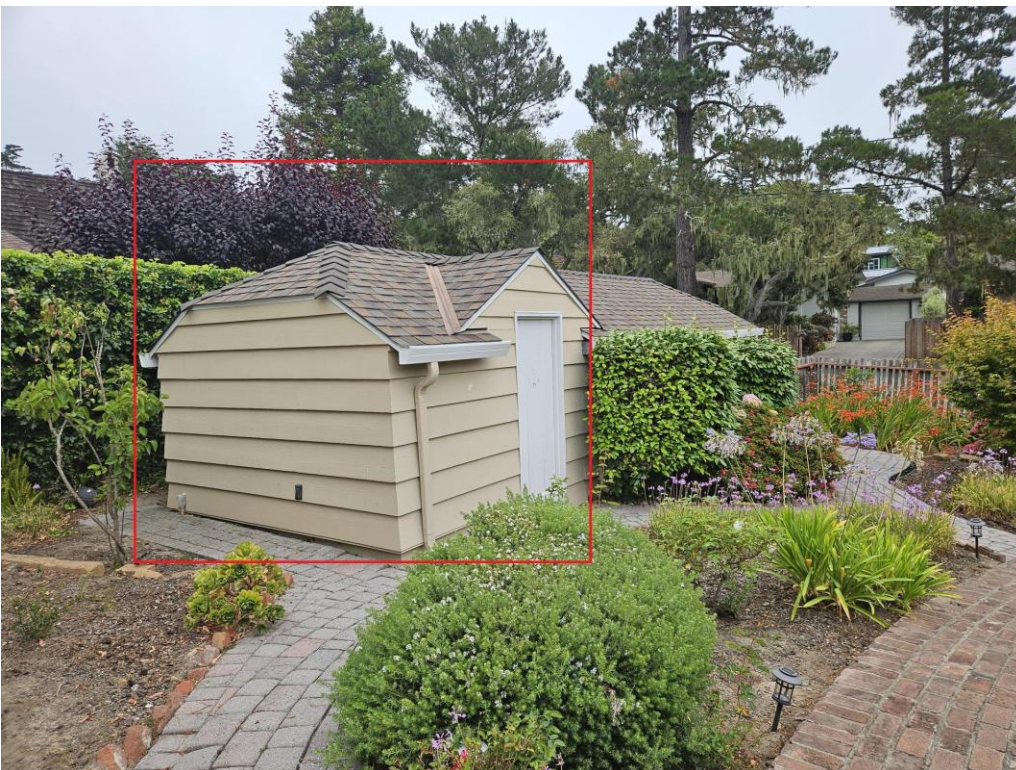
Figure 6: View of garage addition, indicated in red.
