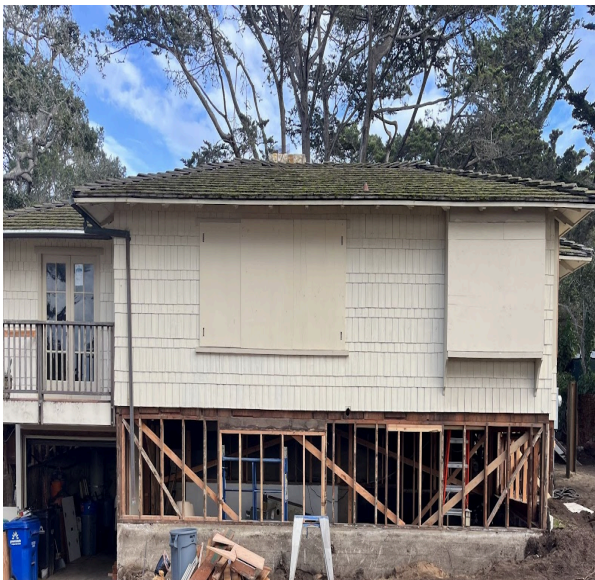
Original Synthetic Roof (Pic #1)
