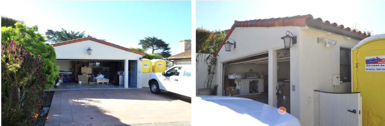
Figures 3 and 4. Left image shows the garage's north elevation and the widened opening. Right image details the north and west elevations. The shed roofed west elevation addition is hidden behind the yellow portable lavatories. 2
