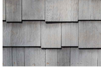
NEW WOOD SHINGLES AT NEW ADDITION
