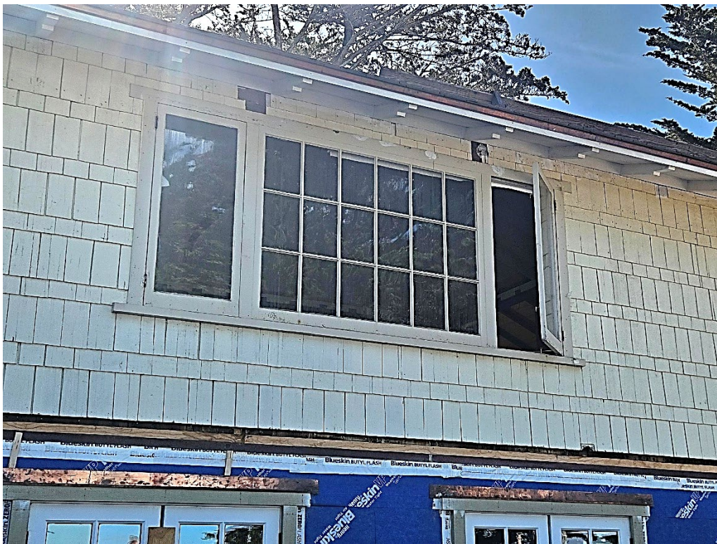
Figure 3: Detail of the one remaining original window on the front elevation.
