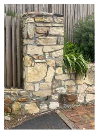
EXISTING CARMEL STONE AT RETAINING WALL DRIVEWAY
