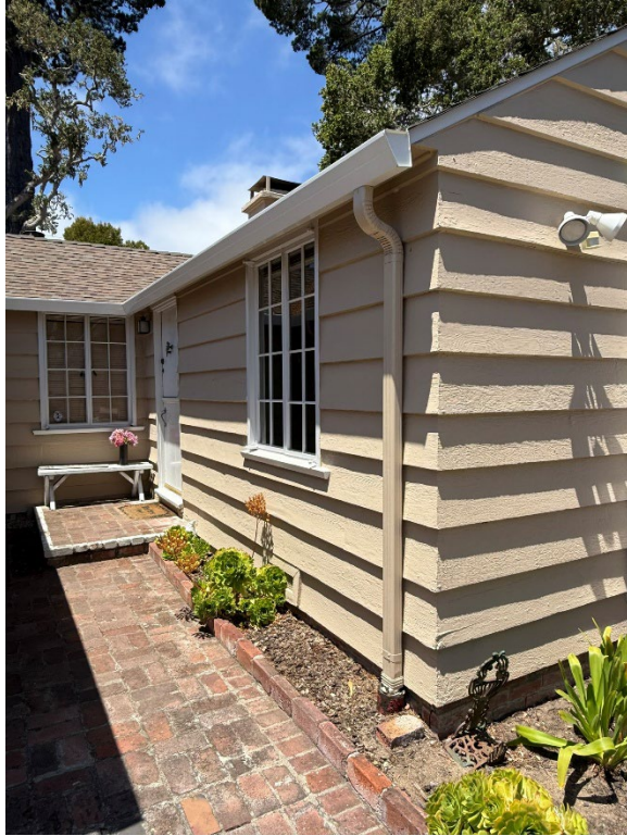
View toward front door (at right)
