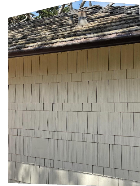
EXISTING WOOD SHINGLES / ROOF SHAKES
