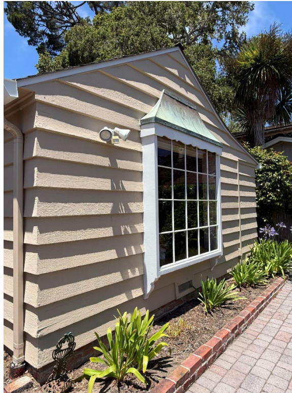
Bay window detail
