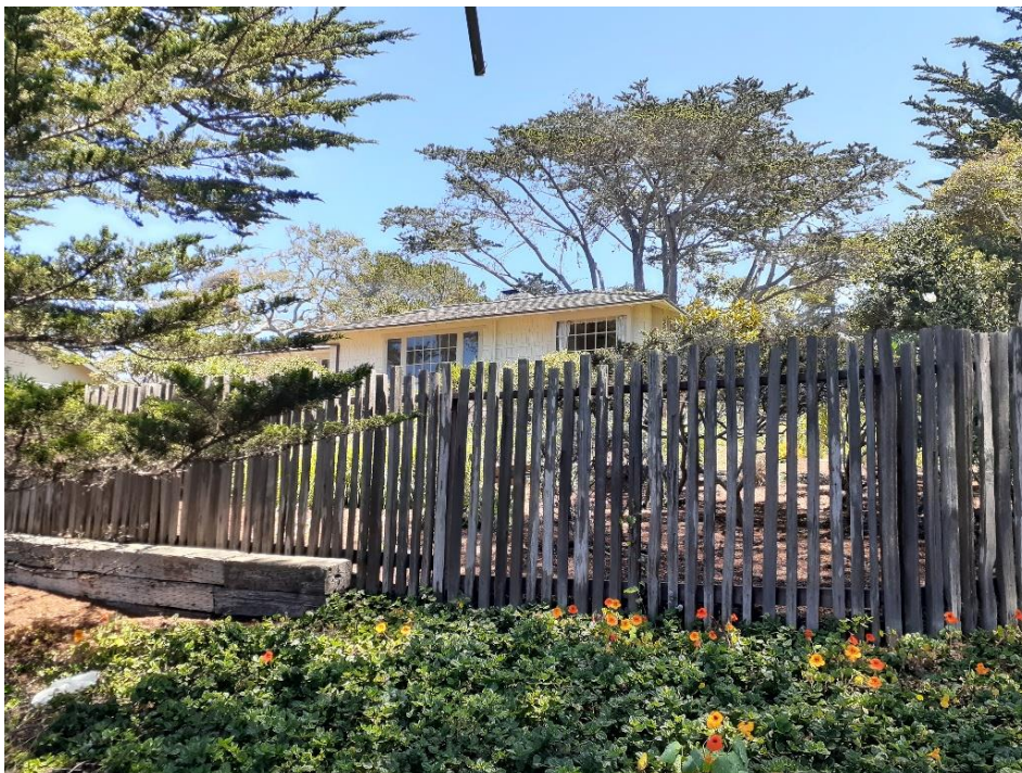
Figure 5: The existing grape stake fence will be retained.
