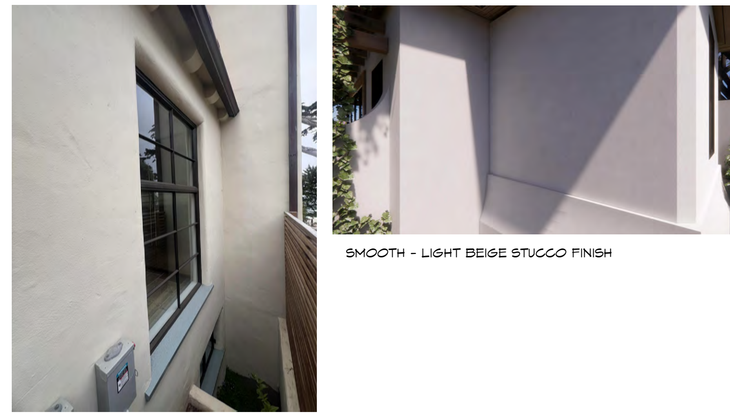
EXISTING STUCCO FINISH
