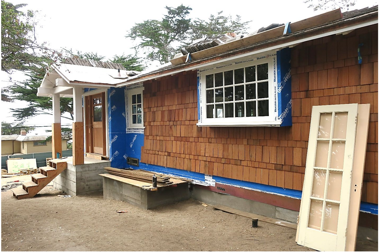
Figure 8: View of new shingles, south elevation.
