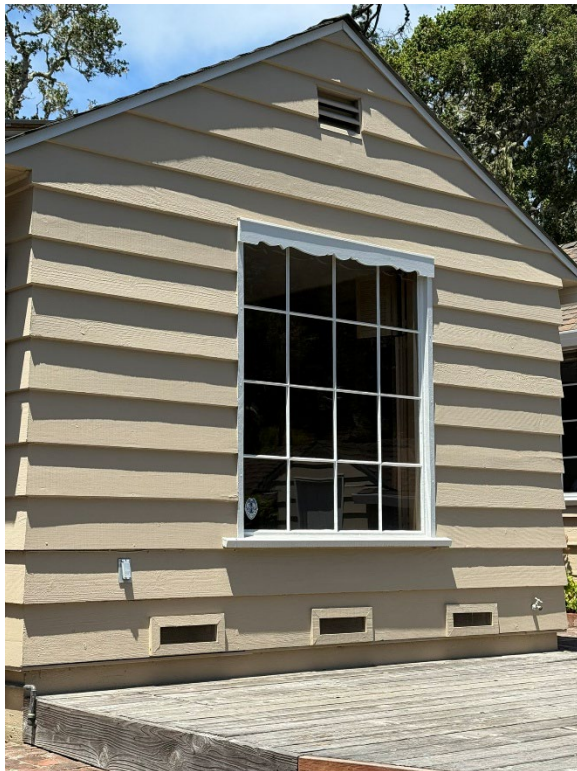
Central wing, facing garden
