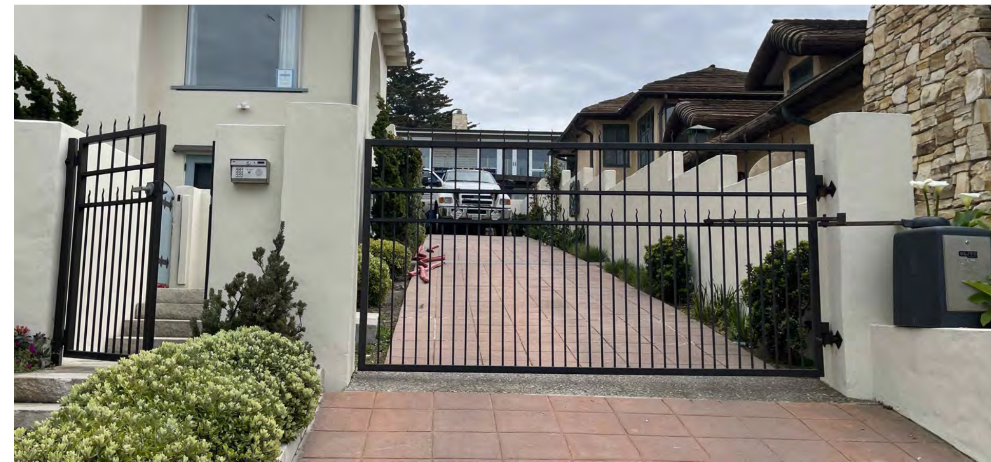
EXISTING DRIVE AND PEDESTRIAN GATE TO BE REPLACED
