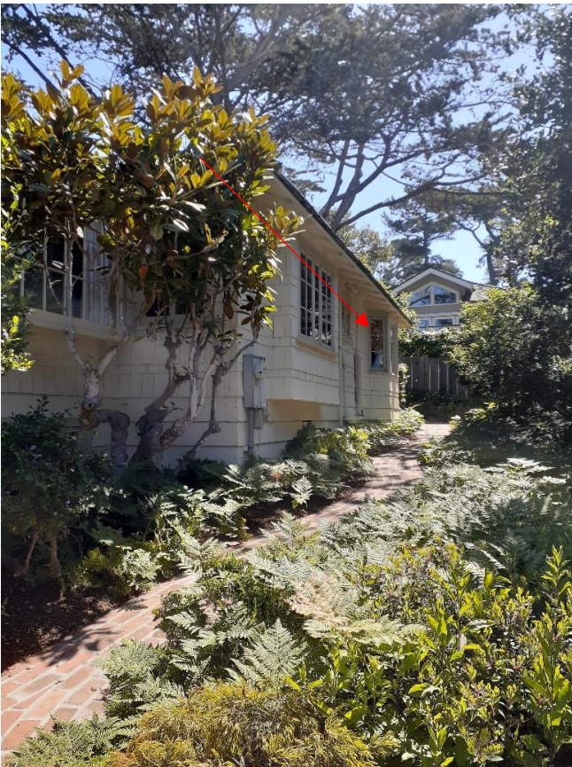
Figure 2: View NE of south elevation with added bay window, indicated with red arrow
