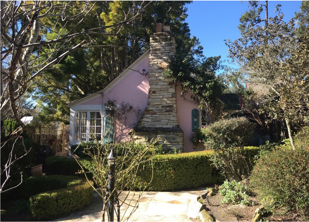
Figure 3: Façade, view looking west from front walkway.
