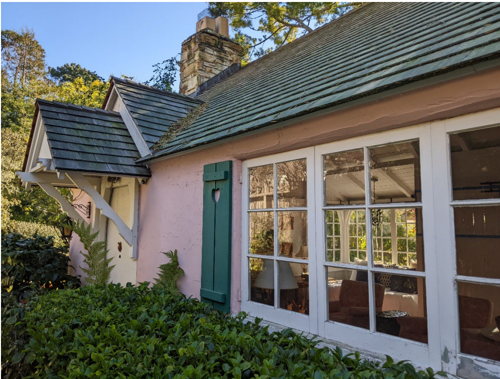
Figure 7: Entry door and bank of three windows to remain in place.
