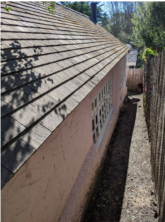
Figure 8: Rear (west) elevation, partially below-grade.
