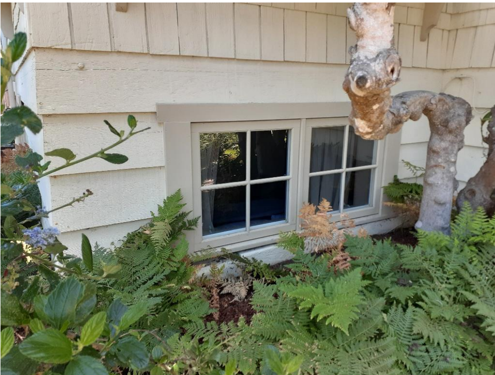
Figure 4: Basement windows on south elevation
