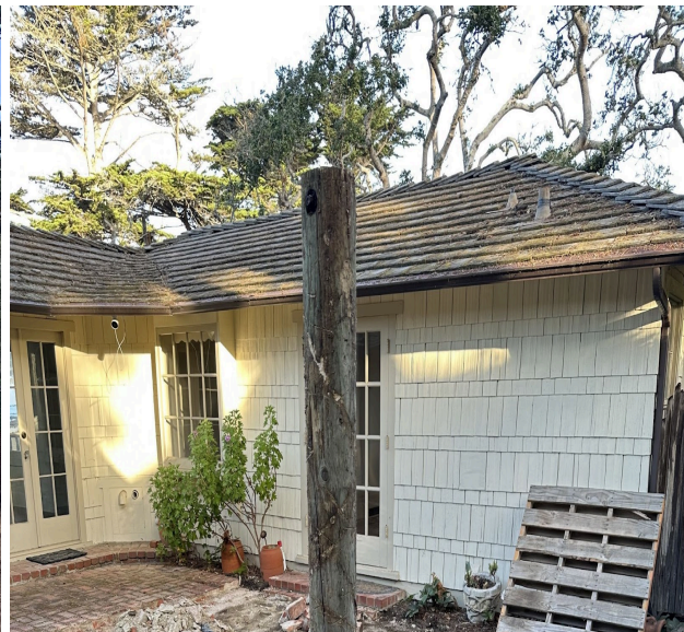
Original Synthetic Roof (Pic#2)
