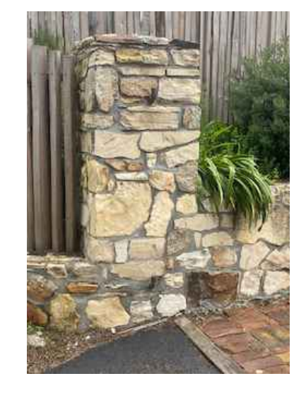
EXISTING CARMEL STONE AT RETAINING WALL DRIVEWAY
