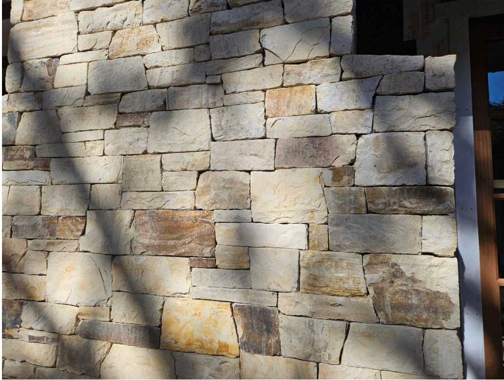
Figure 6: Detail of new chimney.
