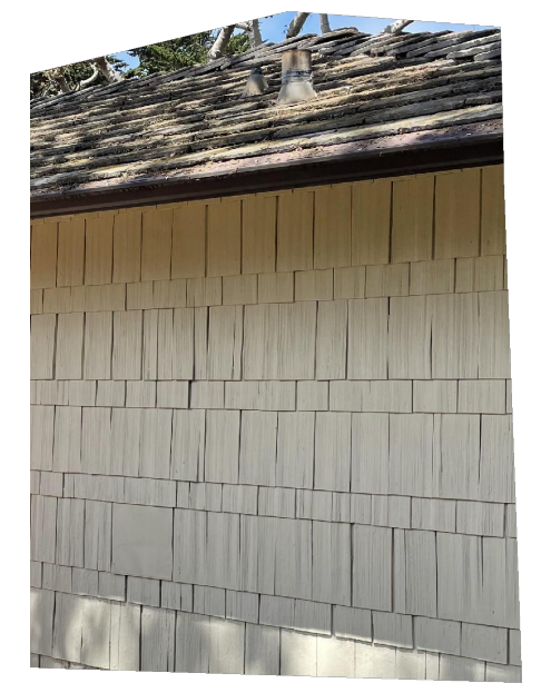
EXISTING WOOD SHINGLES / ROOF SHAKES
