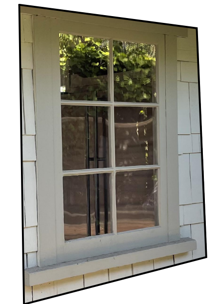
WOOD WINDOWS MATCH EXISTING WITH TRUE-DIVIDED LIGHTS
