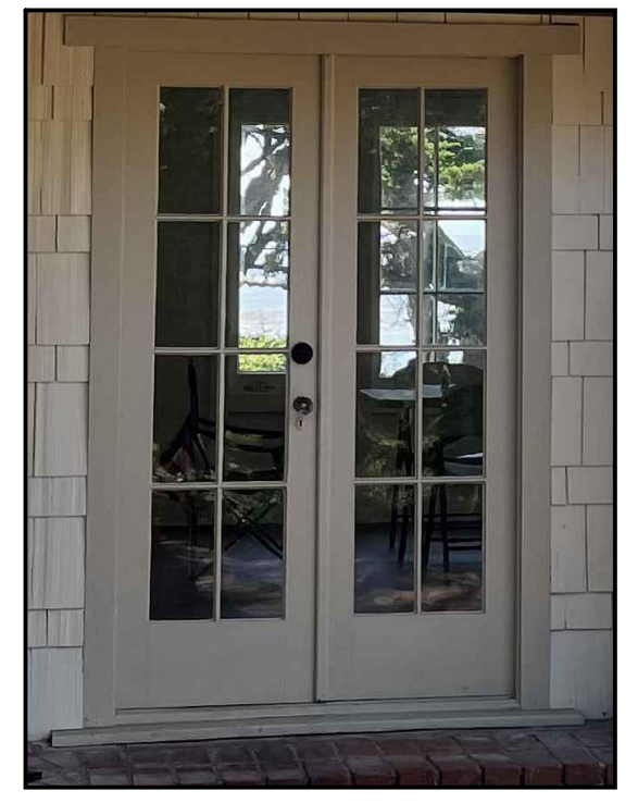
WOOD DOORS MATCH EXISTING WITH TRUE-DIVIDED LIGHTS
