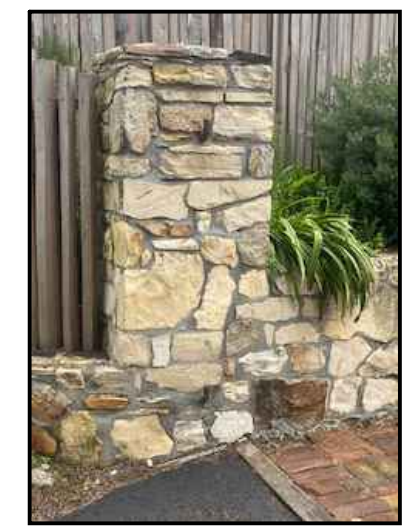
STONE EXISTING CARMEL STONE AT RETAINING WALL DRIVEWAY
