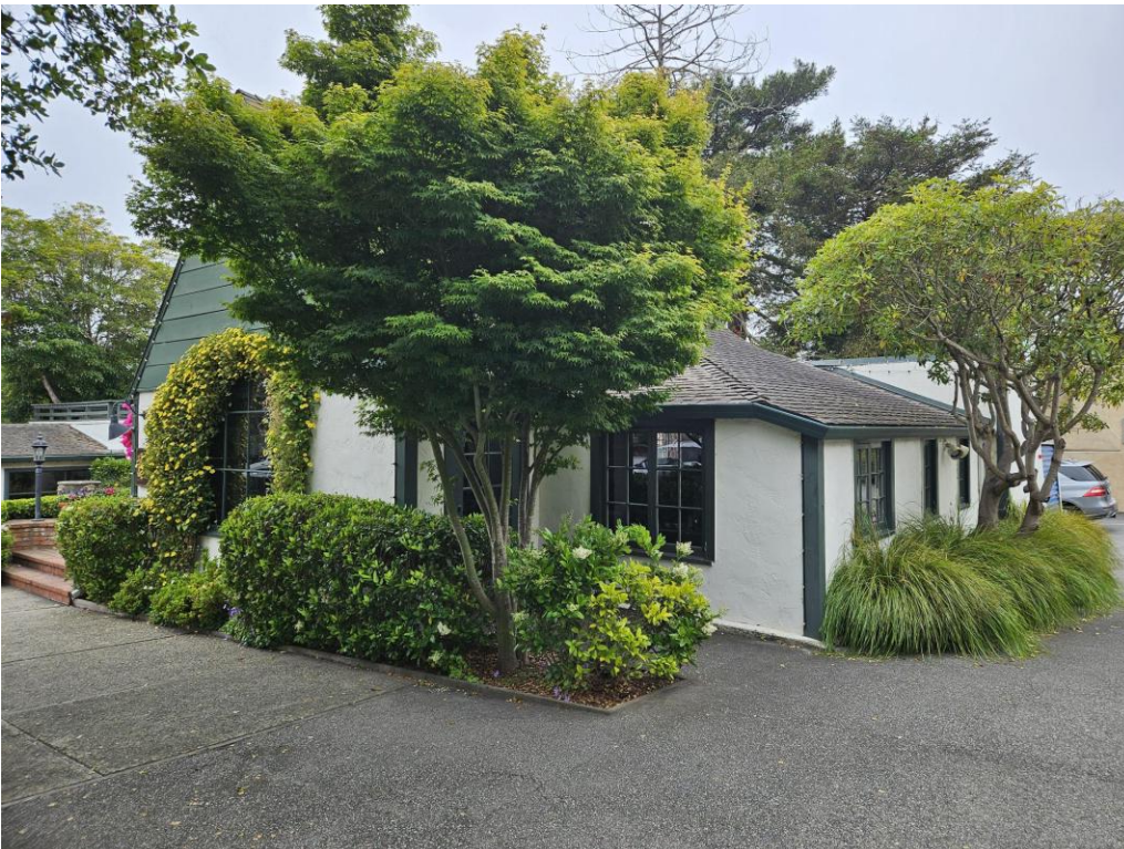
Figure 12: East and north elevations of the house, looking southwest.
