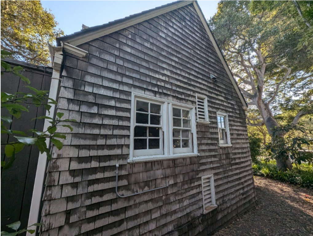
North elevation, view looking southwest.
