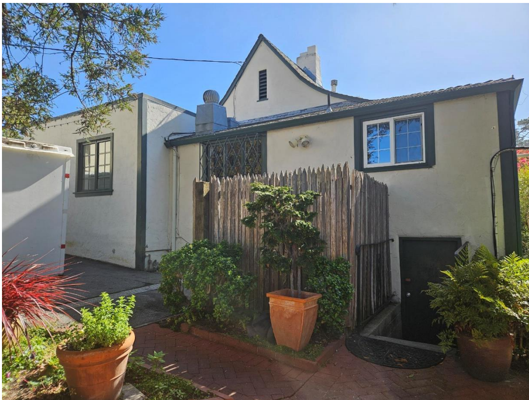
Figure 4: View of rear elevation, 1926 building.
