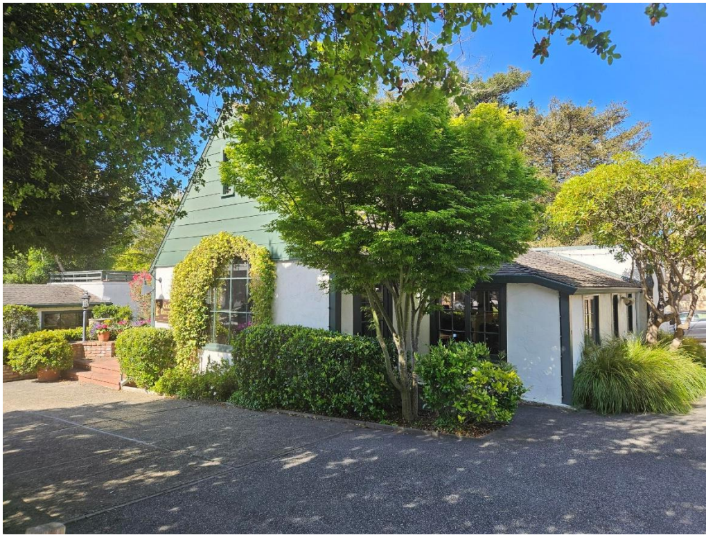
Figure 1: View of front elevation, 1926 building (former James & Irene Kitchen house).
