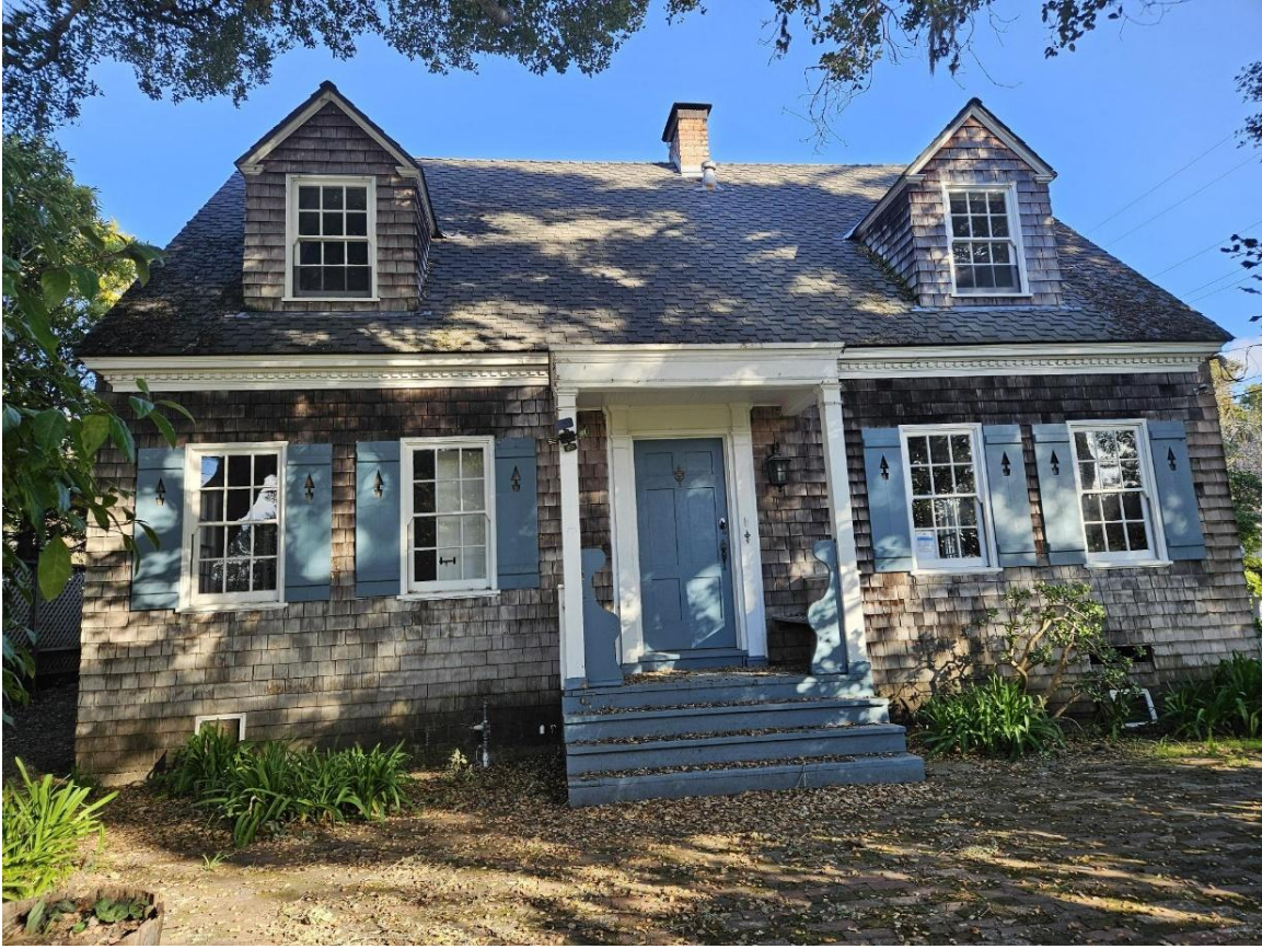
Figure 1: View of front elevation looking east from Camino Real.
