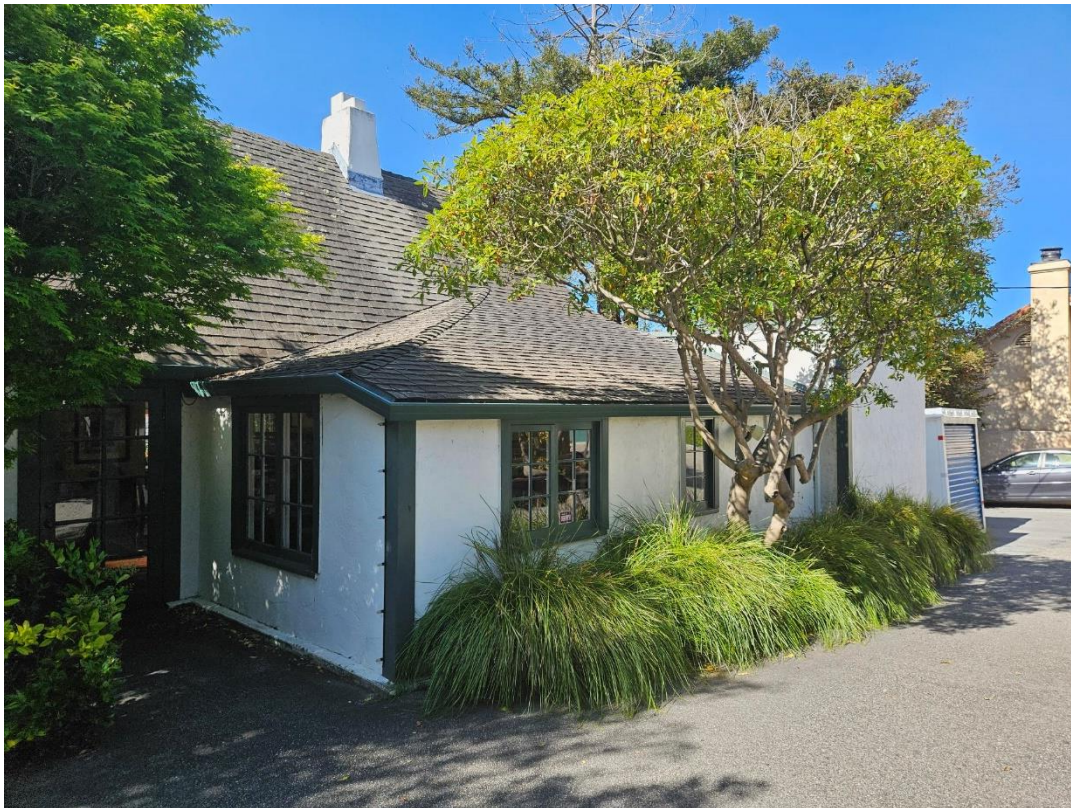
Figure 2: View of north elevation, 1926 building.
