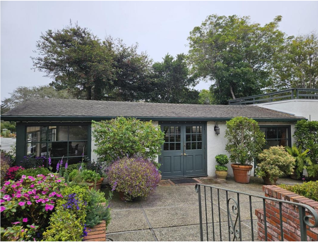
Figure 6: View of plumbing shop north elevation, 2025.
