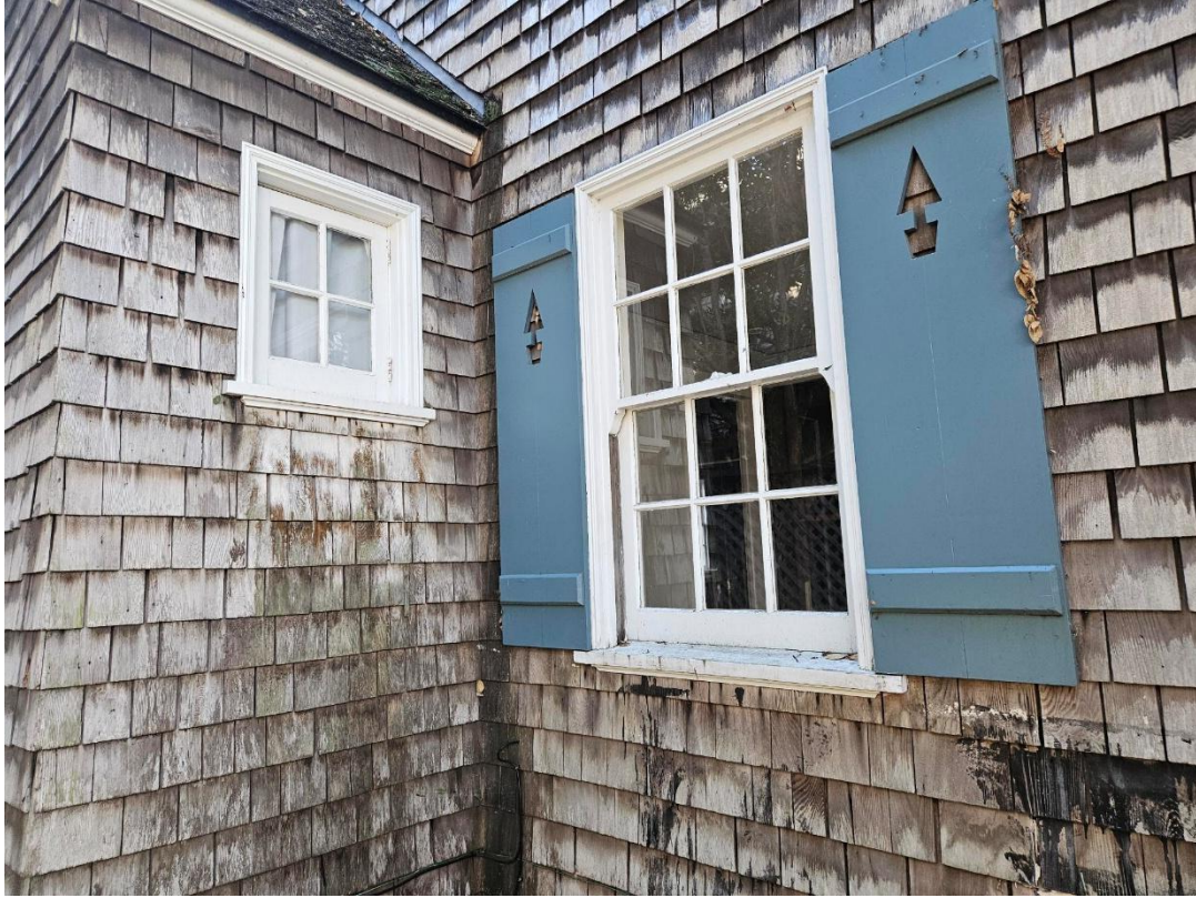
Figure 3: Detail of shingles proposed for removal.
