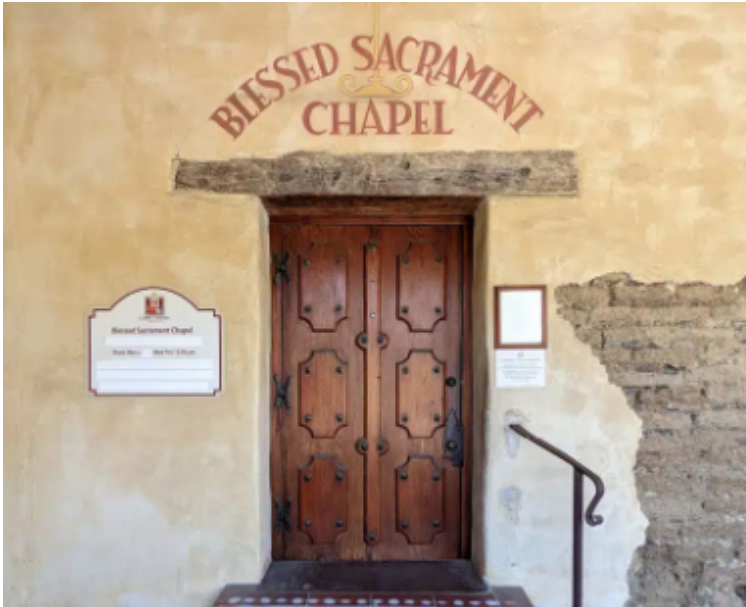
Figure 6: Blessed Sacrament Chapel door, to be moved forward towards the exterior loggia wall (no change to opening size).
