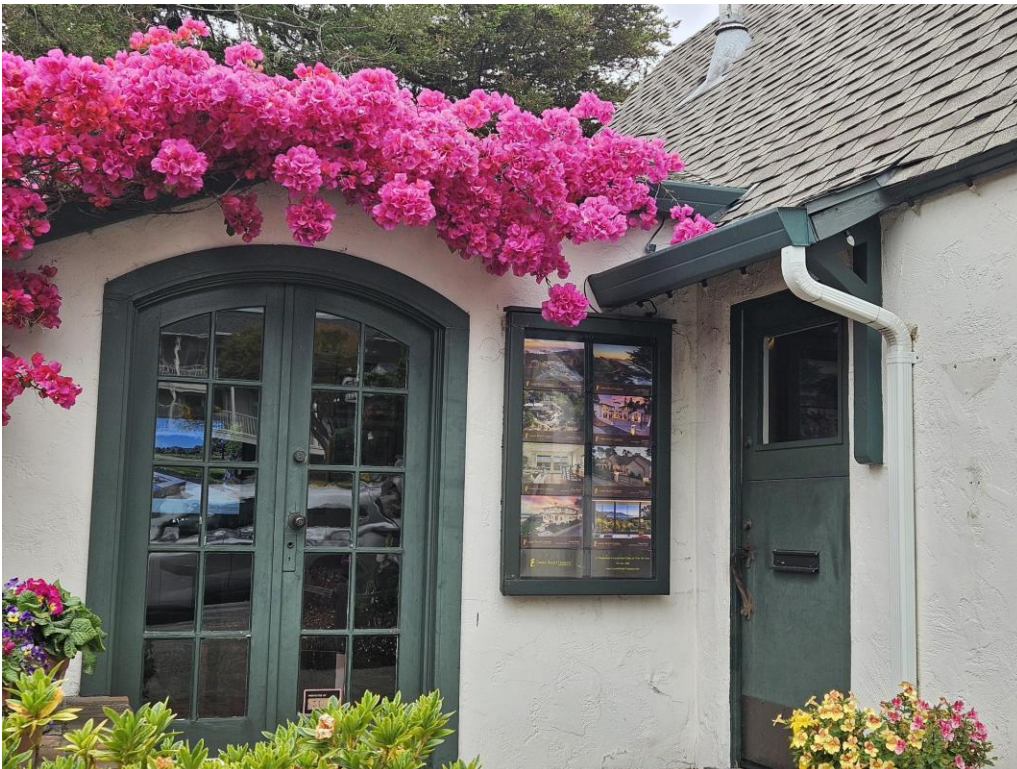
Figure 16: Detail view of the front entrance.
