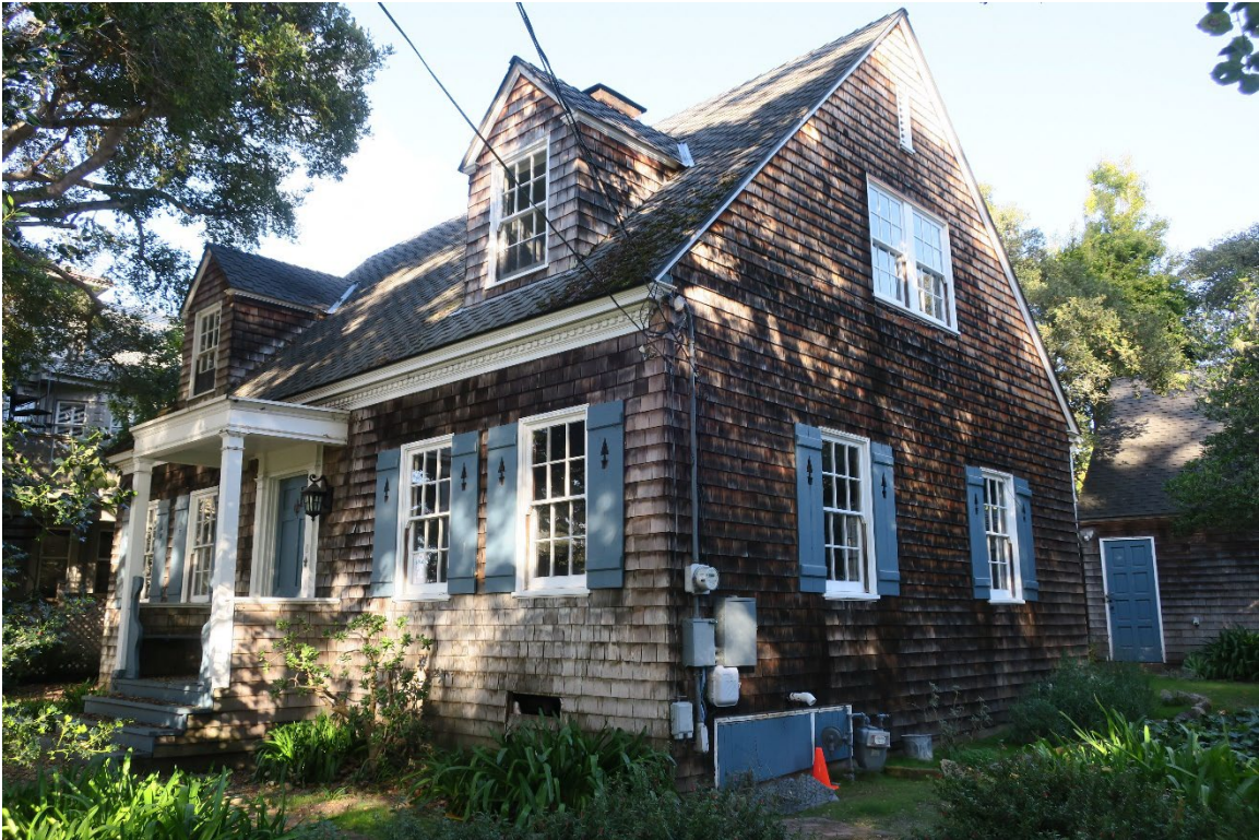
Façade and south elevation, view looking northeast.
