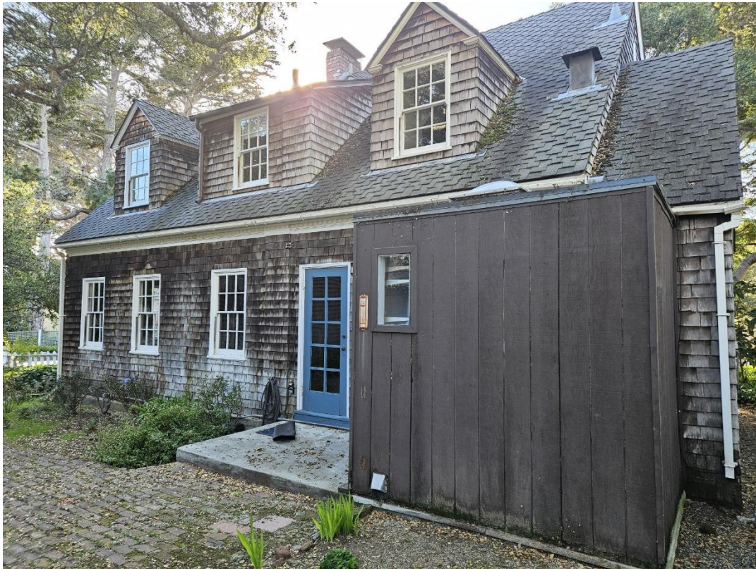
Figure 2: View of the rear elevation looking southwest.
