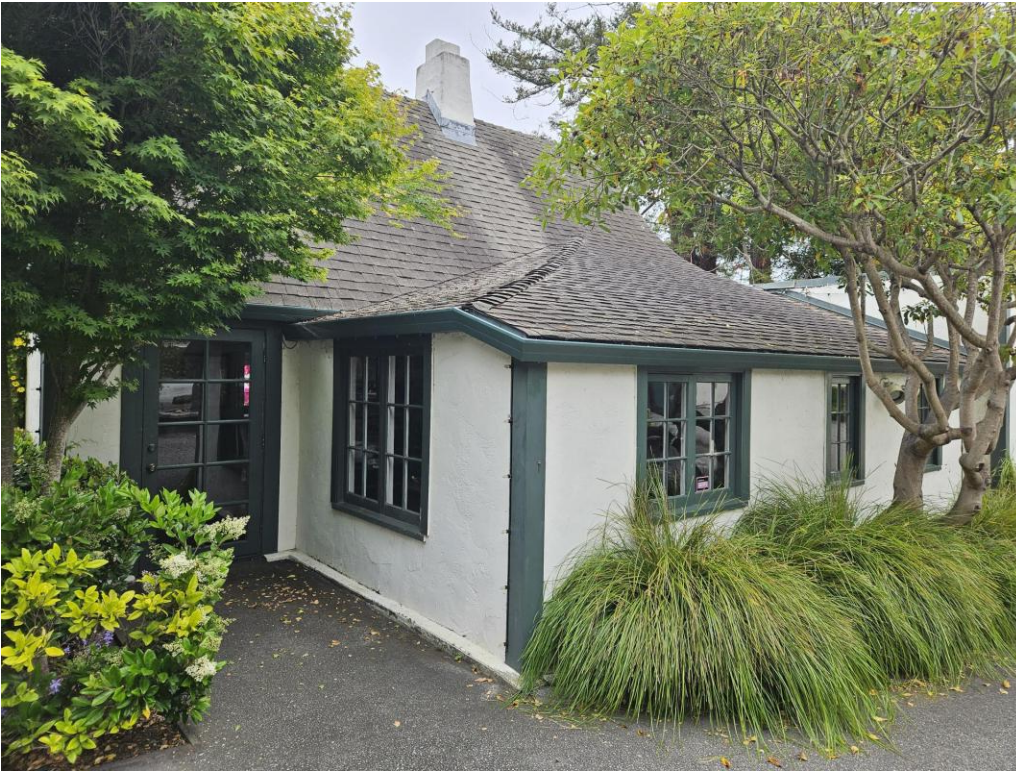
Figure 13: Detail of the east elevation.
