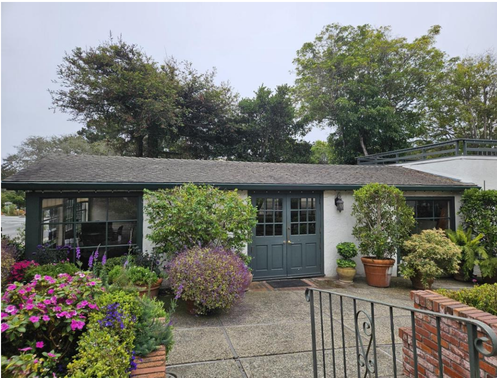
Figure 6: View of plumbing shop north elevation, 2025.
