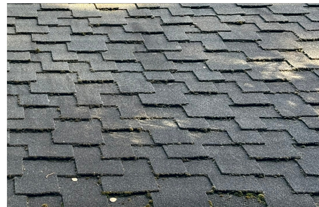
EXISTING ROOFING - COMPOSITION
