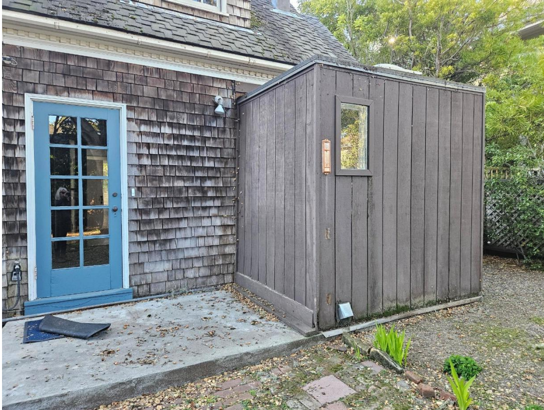
Figure 2: View of rear door to be replaced.
