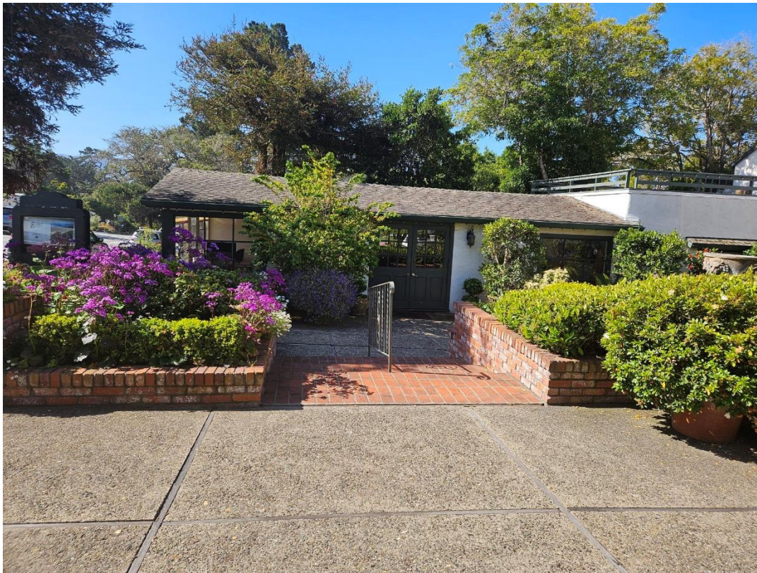
Figure 7: View of north elevation, 1935 plumbing shop.
