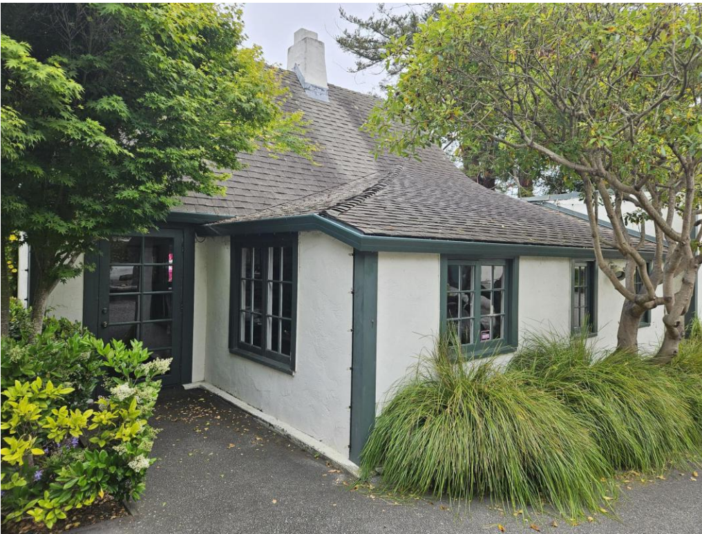
Figure 13: Detail of the east elevation.
