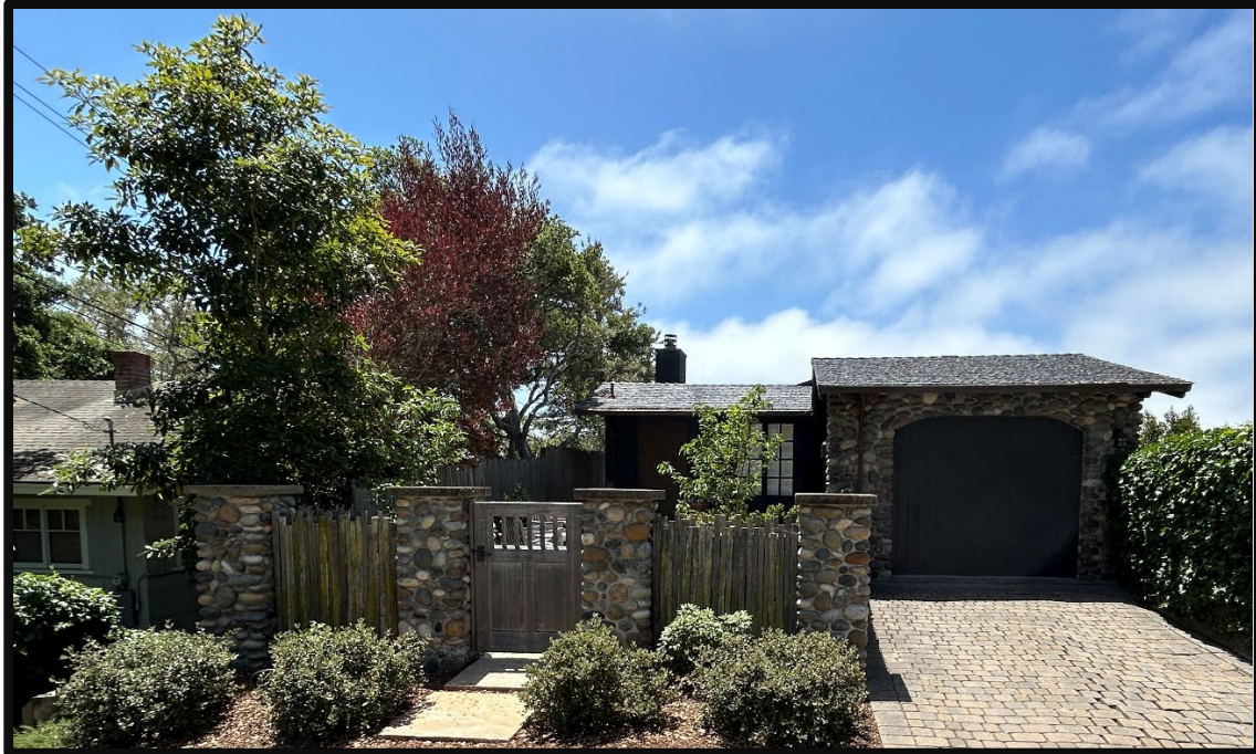
6.2.2. Do not stop wall materials at corners, instead wrap them around the entire building. (See Application of Stone Veneer in the Above Image)
