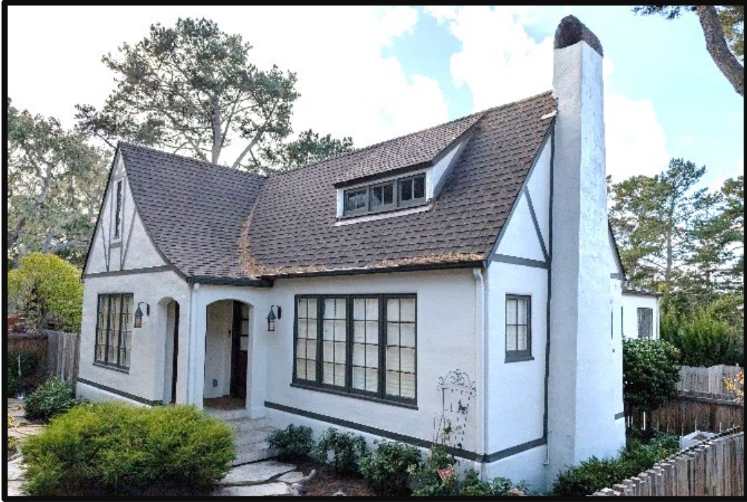
6.3.2. Integrate the primary entrance with the overall design of the house. (See Entry in the Above Image)
