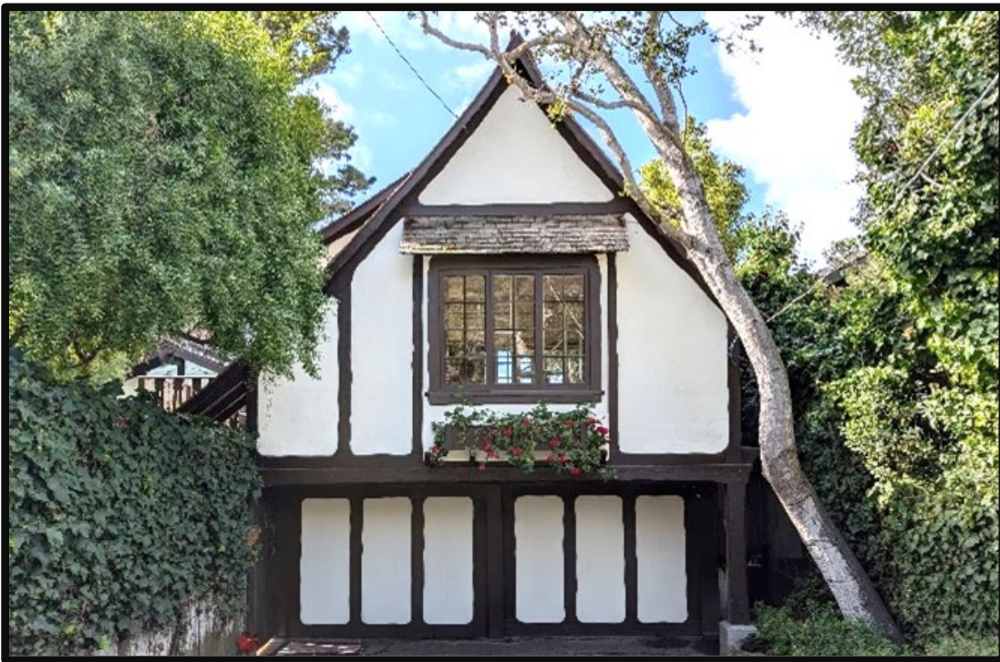
6.3.3. Rather than installing a standard overhead product, craft a garage door either to provide visual interest, to recede completely into the materials and colors of the building wall, or orient it so as not to face the street. (See Garage in the Above Image)
