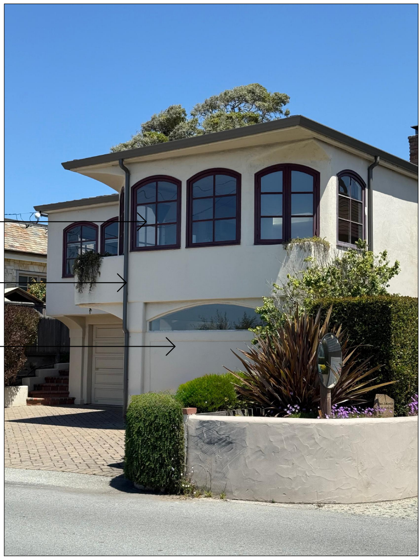
VIEW @ SOUTHWEST CORNER
