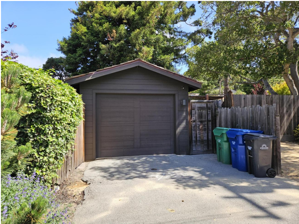
Figure 1: Garage looking north from 13 th Avenue.
