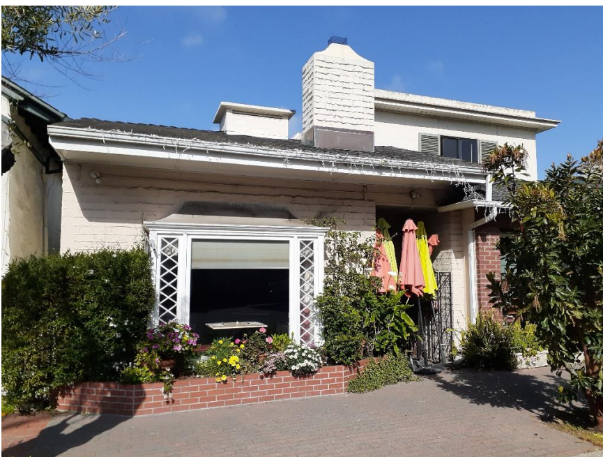
Figure 3: View of 1941 building (Building #3) looking west
