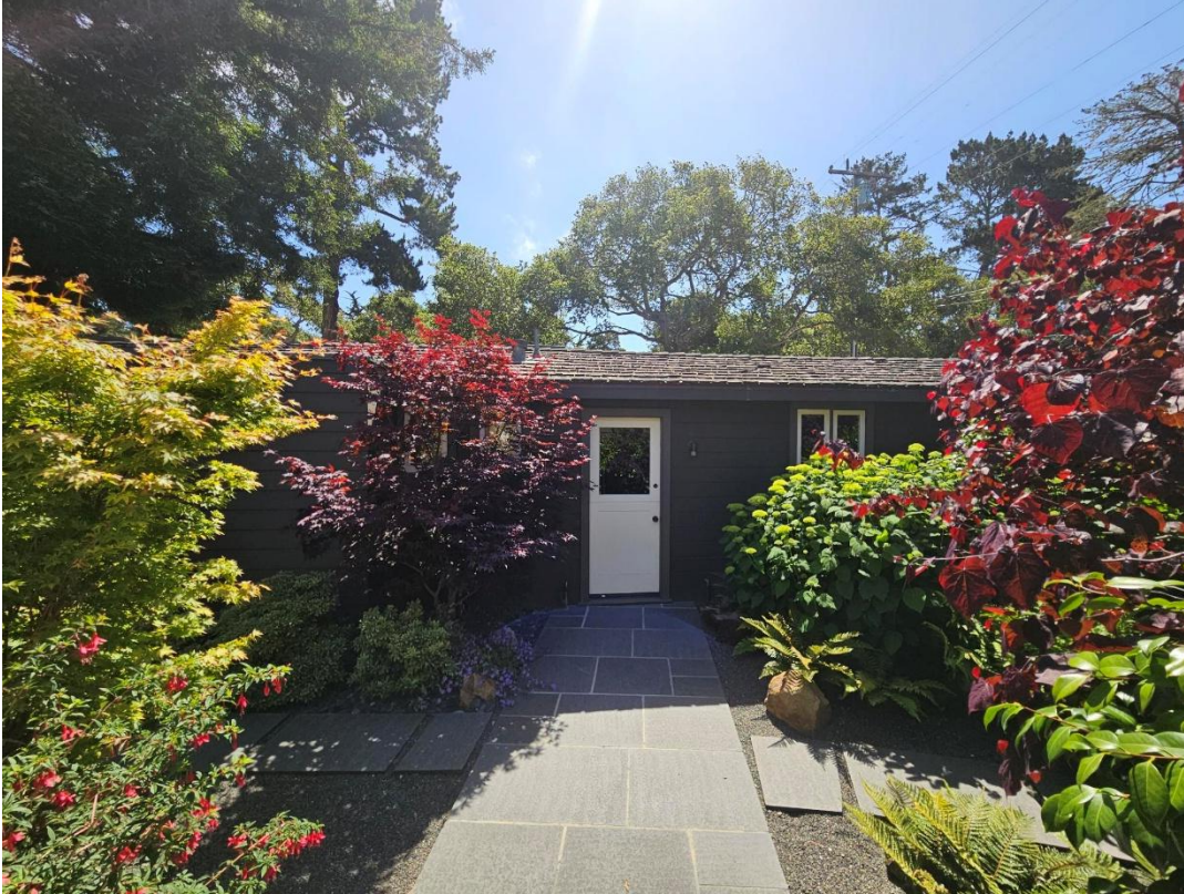
Figure 2: View of 1957 garage, looking east.
