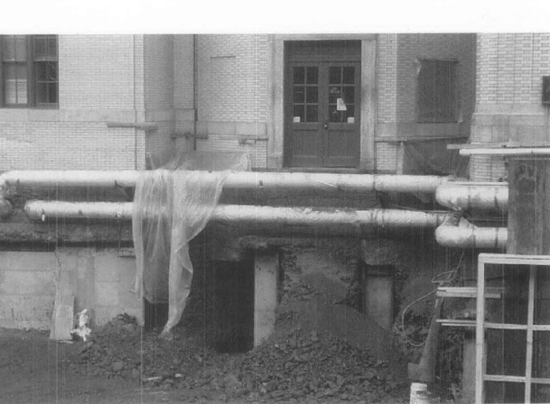
Figure 3. Concrete pier underpinning to an existing building may be necessary when adjacent construction occurs. In this example, piles are hand dug beneath the foundation of the historic building to provide support for new concrete. After the concrete is poured into the holes, the top of the pier and the bottom of the original foundation is packed with a quicksetting grout. The historic building owner should retain an independent engineer to ensure that the underpinning plan adequately protects the historic structure. Photo: Professor Arpad Horvath, Department of Civil and Environmental Engineering, University of California, Berkeley.
