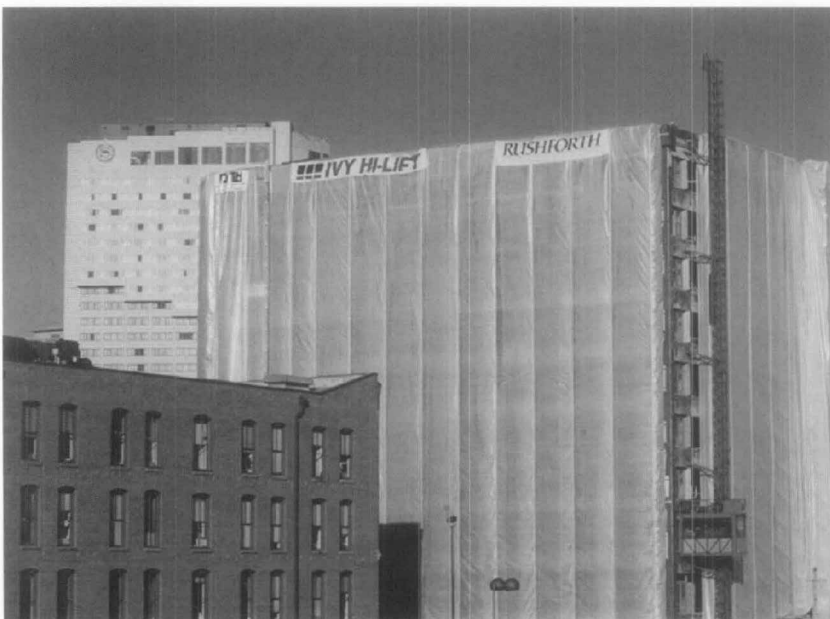
Figure 5. The historic building on the left is partially protected from debris and dust generated by the renovation of the structure to the right. Such temporary enclosure systems consist of a polyethylene or other fabric shell stretched between an aluminum frame. Photo: Walton Technology, Inc.
