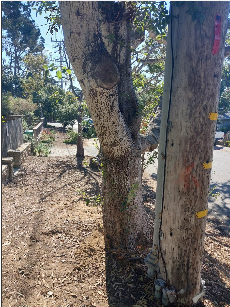
Photo 4: A telephone pole growing within 1-foot of the base of the tree.
