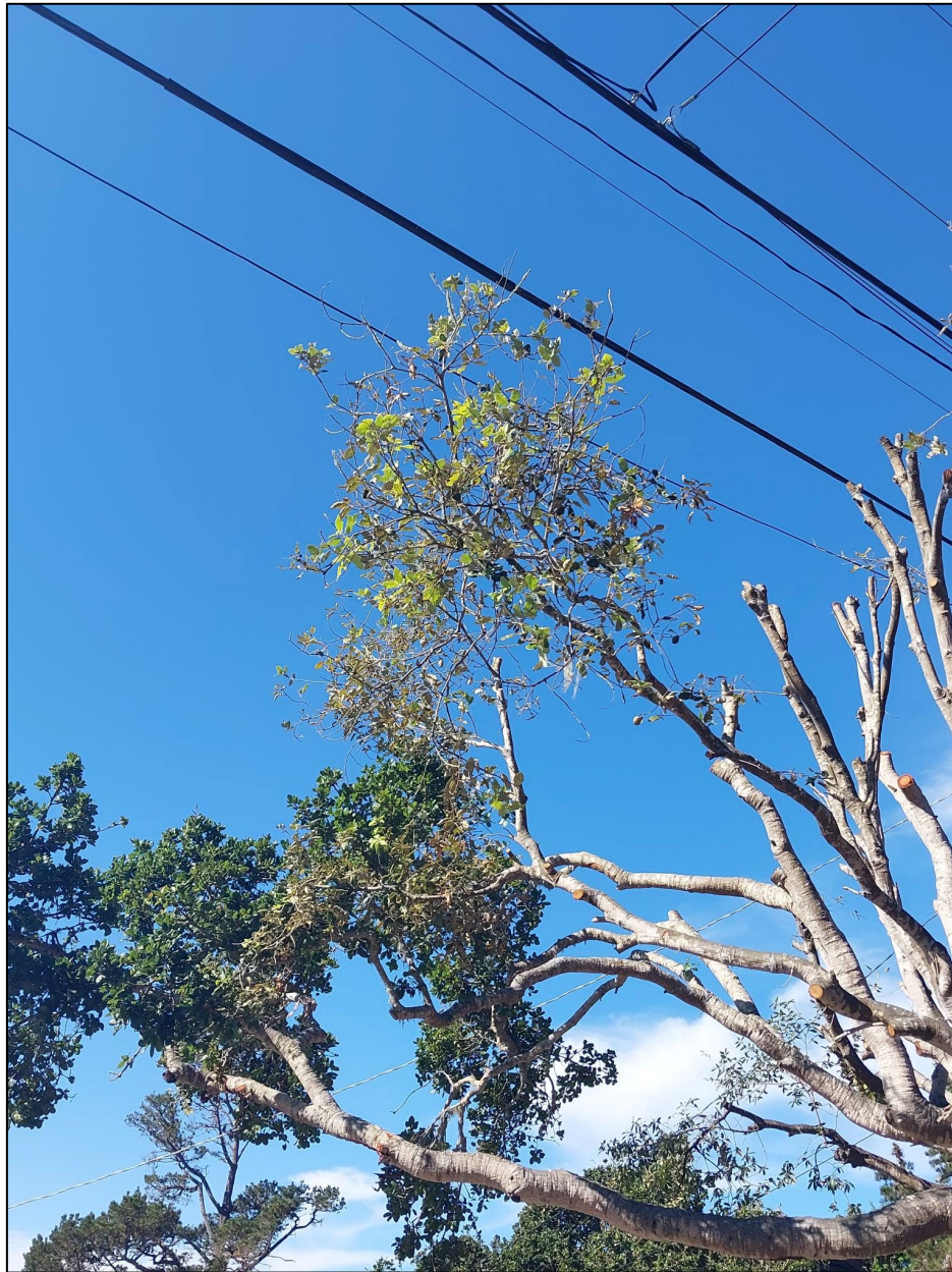
Photo 11: Foliage remaining in the canopy is sparse with twig dieback present.
