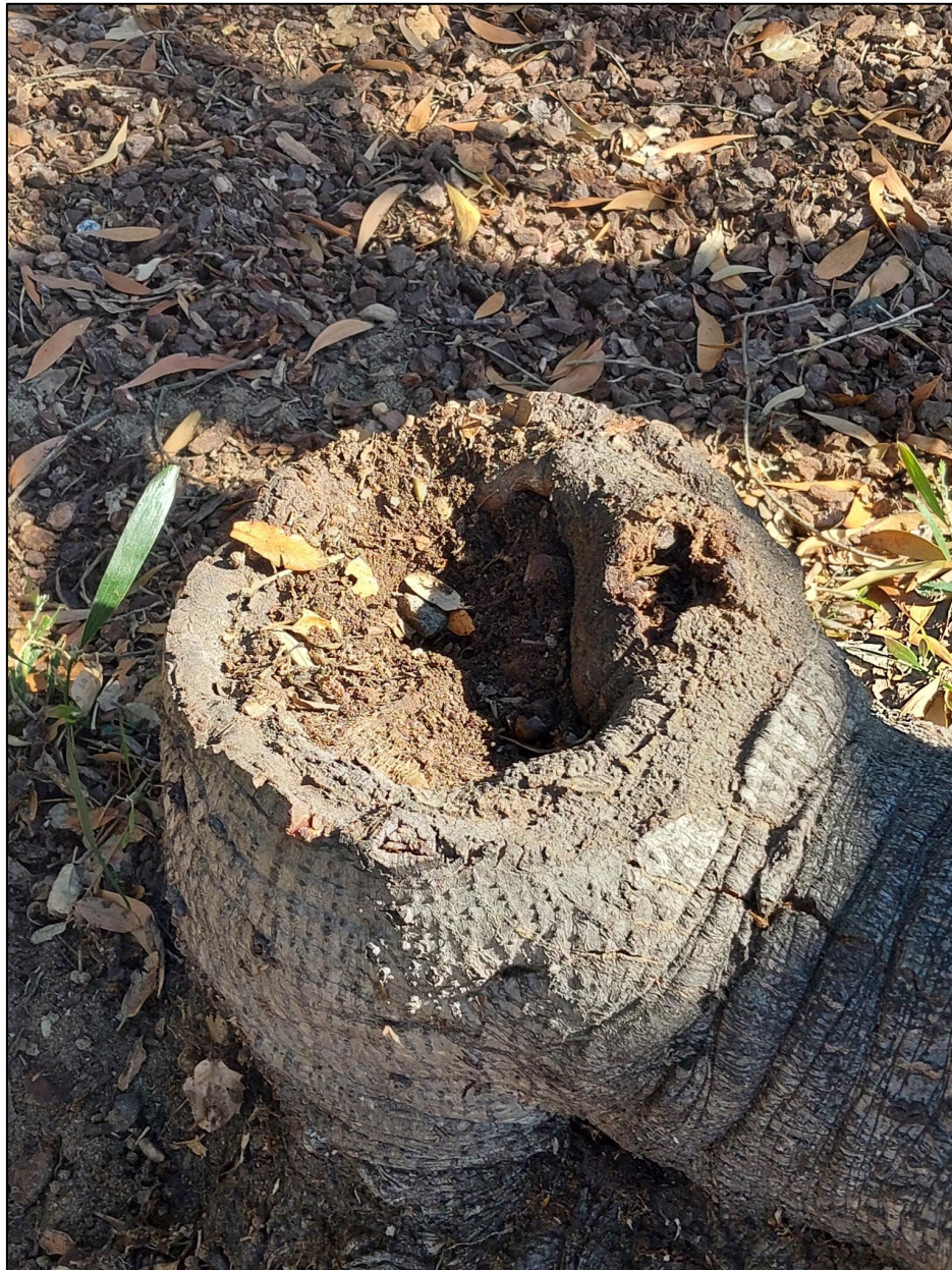
Photo 8: Decay present in the codominant attachment where a previous leader was removed.
