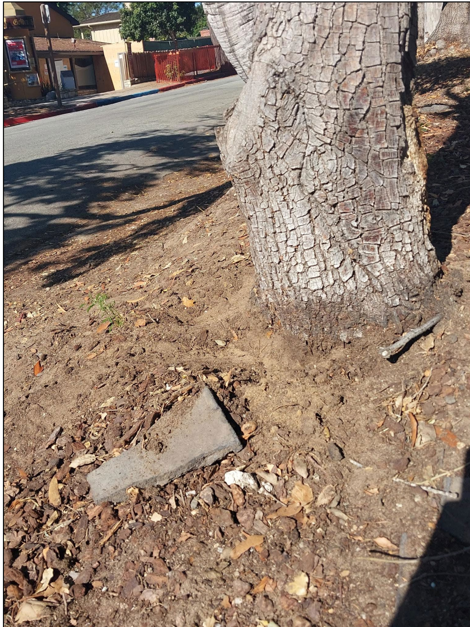
Photo 12: I exposed the tree's root collar by pushing back soil around the tree base, revealing the buried area.
