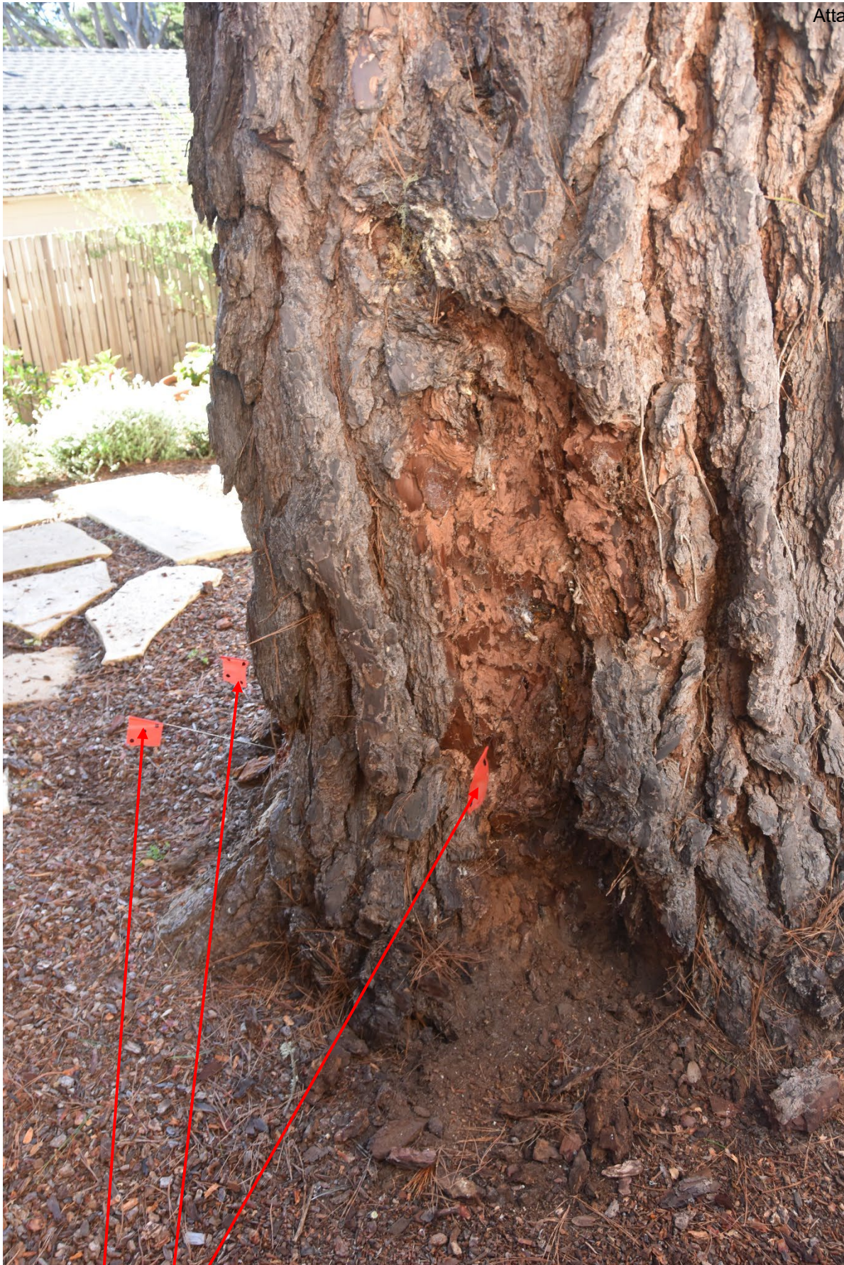
Drill holes #3, #4, and #2
