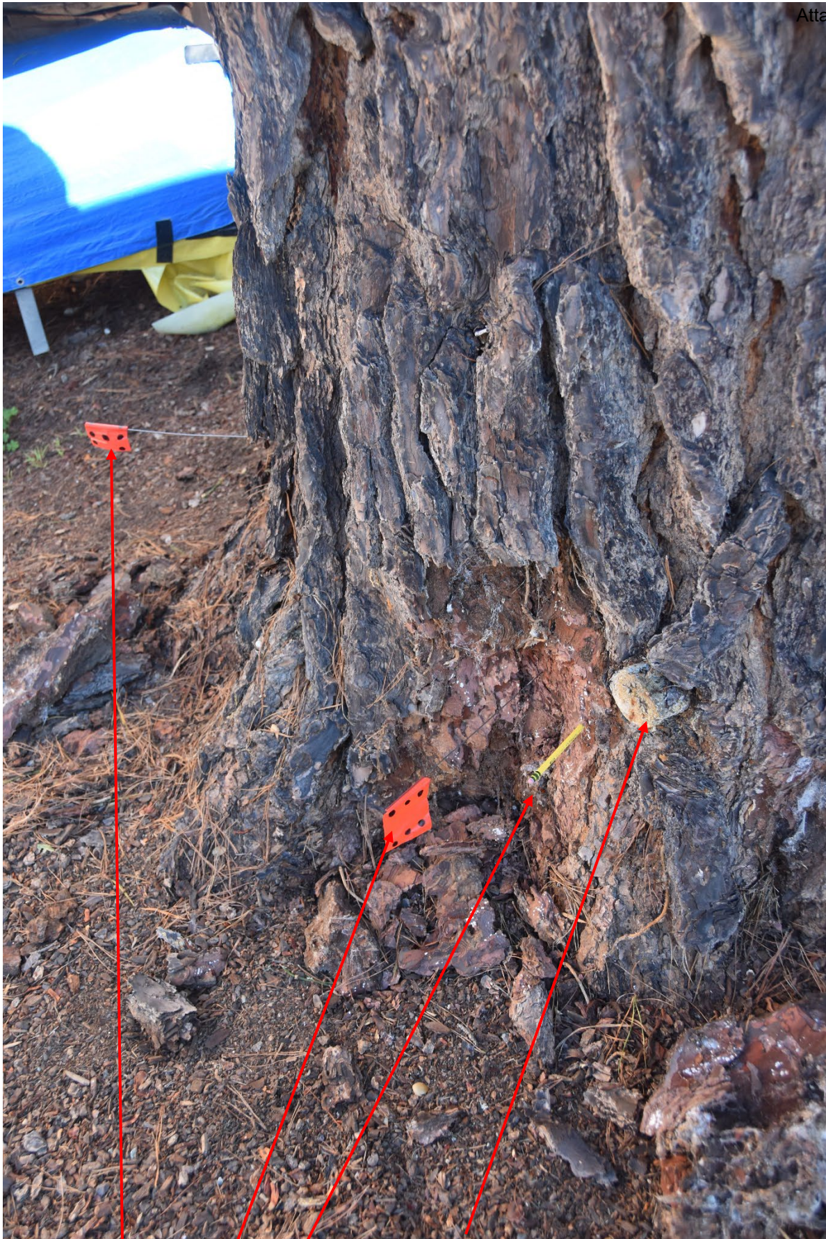
Drill holes #7, and holes #6 and #6.1 adjacent to old stub.
