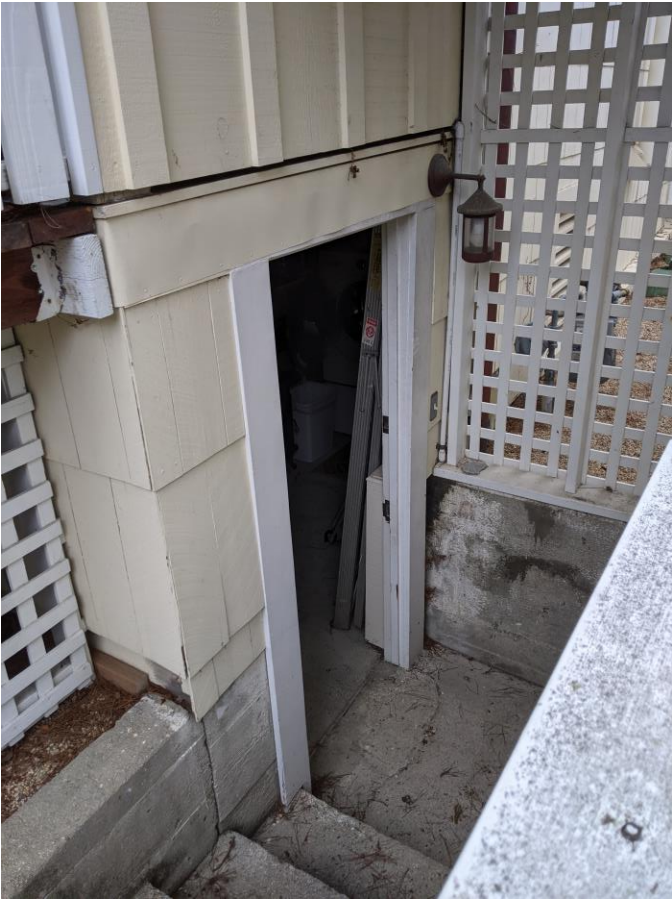
Basement door located at southeast corner of the home.
