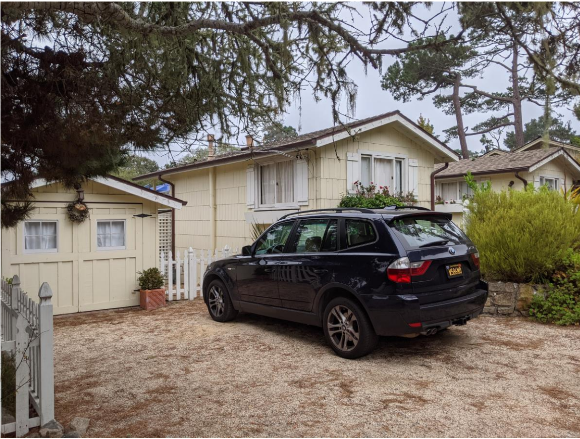
East elevation and north façade.
