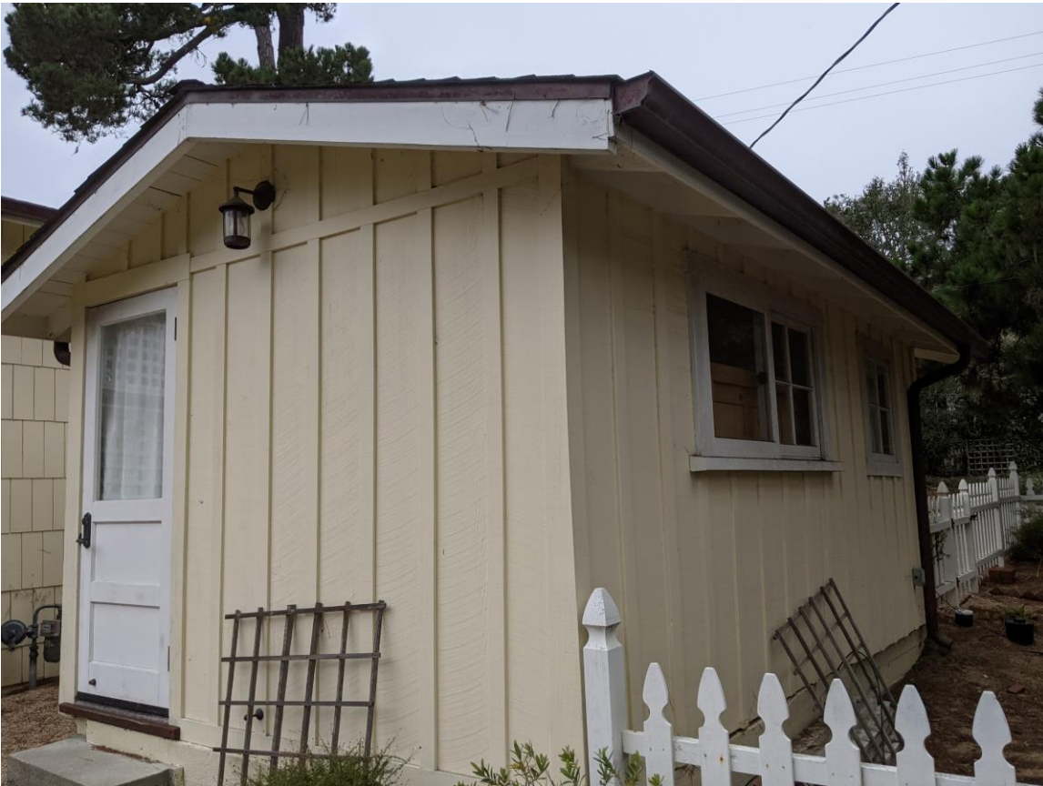
Board and batten gabled garage (south and east elevations).
