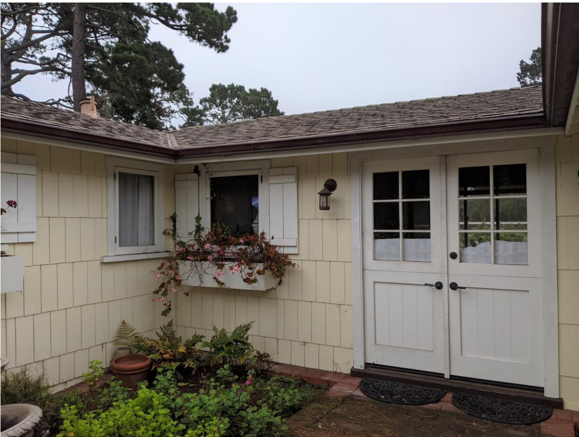
Primary entrance at façade. Two casement windows pictured east of the double Dutch doors.
