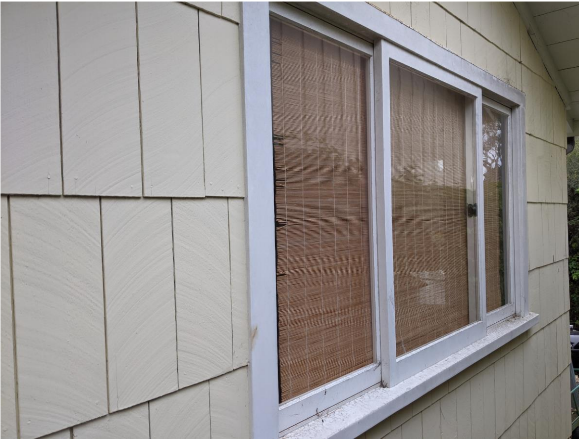
Tripartite style sliding window at west elevation.
