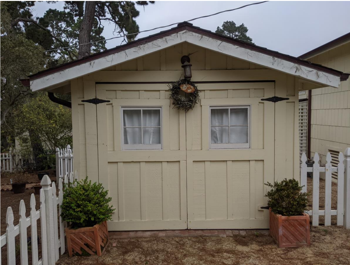
North façade of garage.
