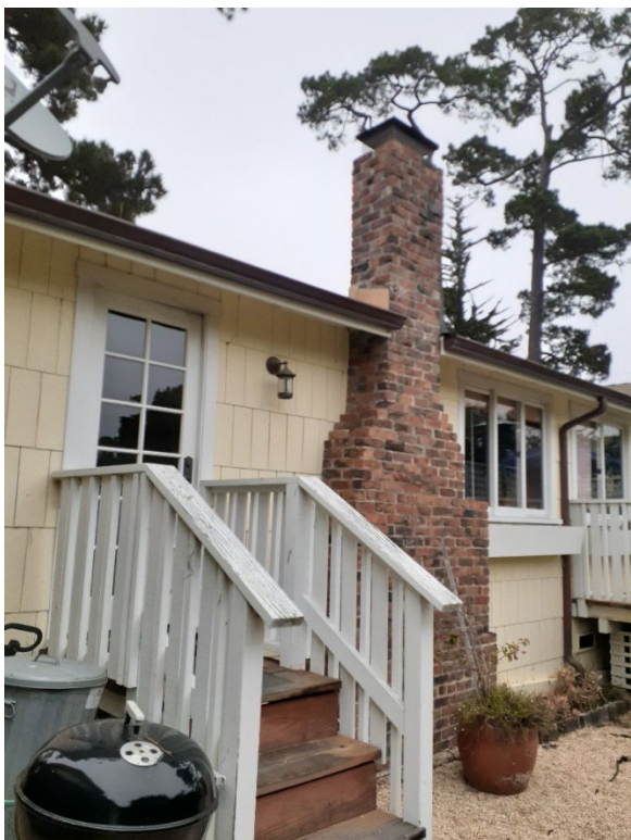
Figure 6: View of chimney, rear elevation
