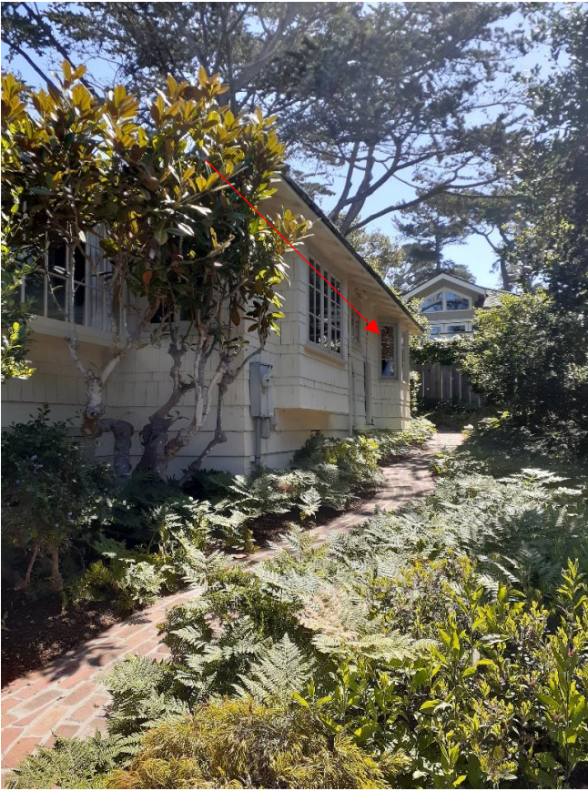
Figure 2: View of south elevation with added bay window
