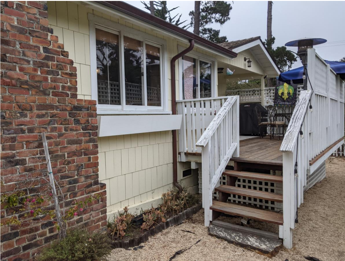
Tripartite sliding window and non-historic deck at rear (south) elevation.
