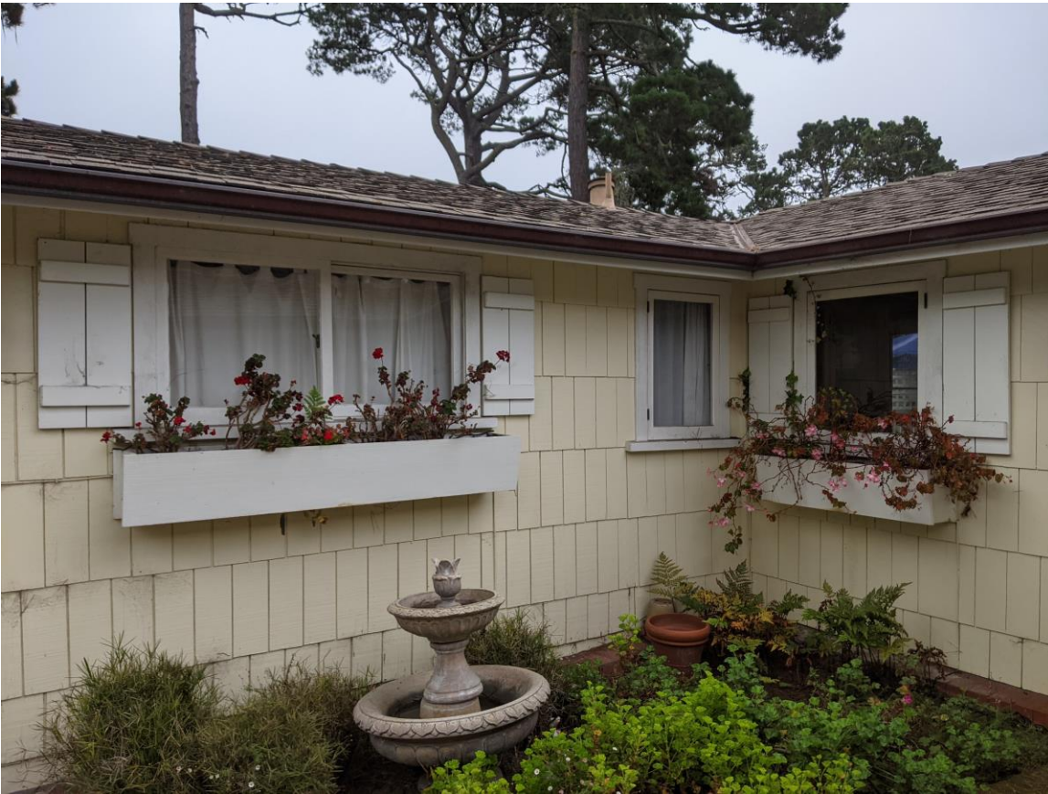
Two-lite sliding window. Non-original shutters and window boxes.
