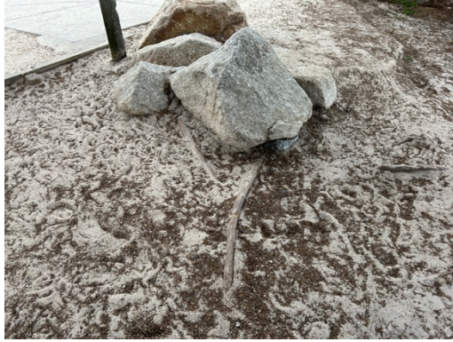
Exposed Roots, Erosion Near Hardscaping
