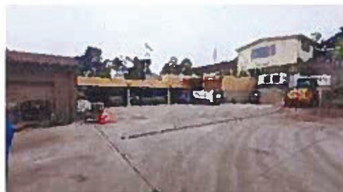
Figure 8 – Existing site paving
