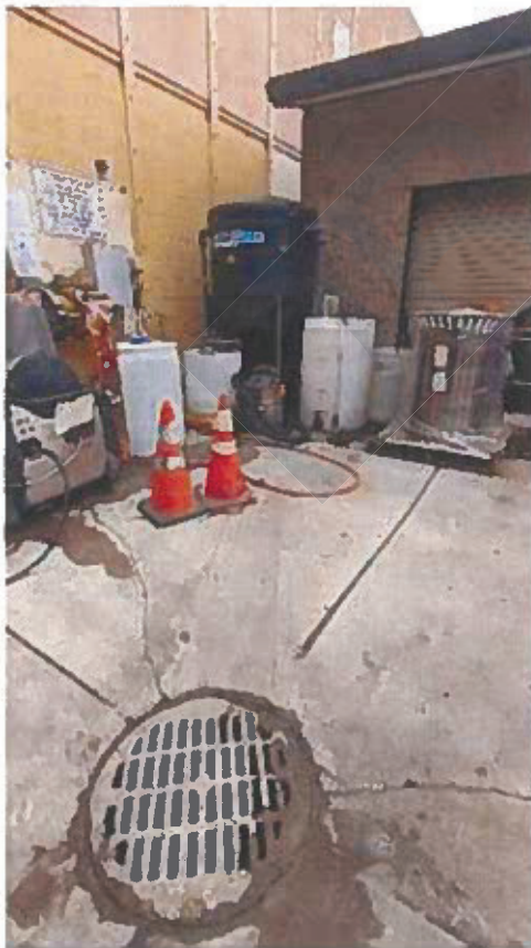
Figure 12 – Existing storm drain
