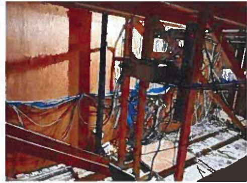
Figure 52 - Existing attic IDF with unsafe floor
