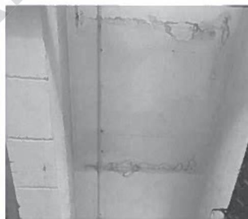
Figure 14 – Moisture stains through cracks in existing concrete slab
