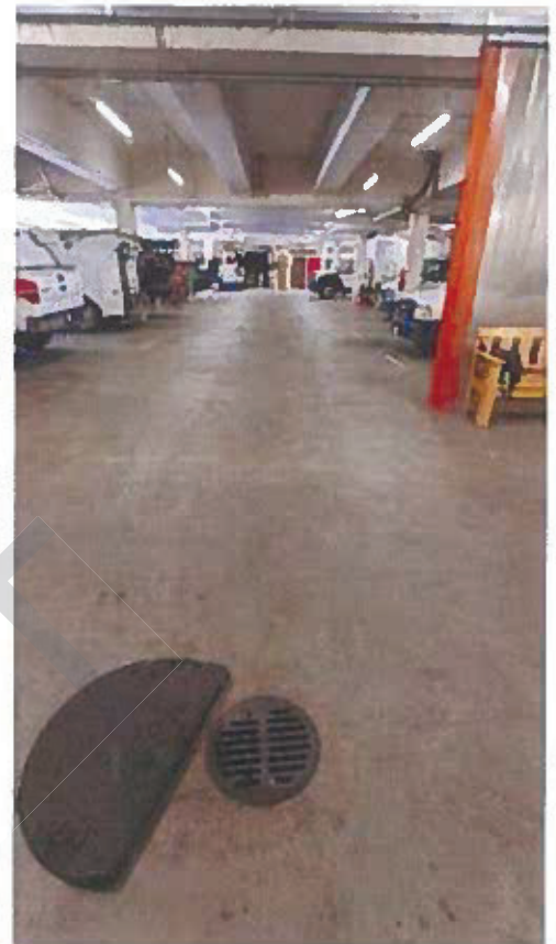
Figure 11 – Existing garage floor drains
