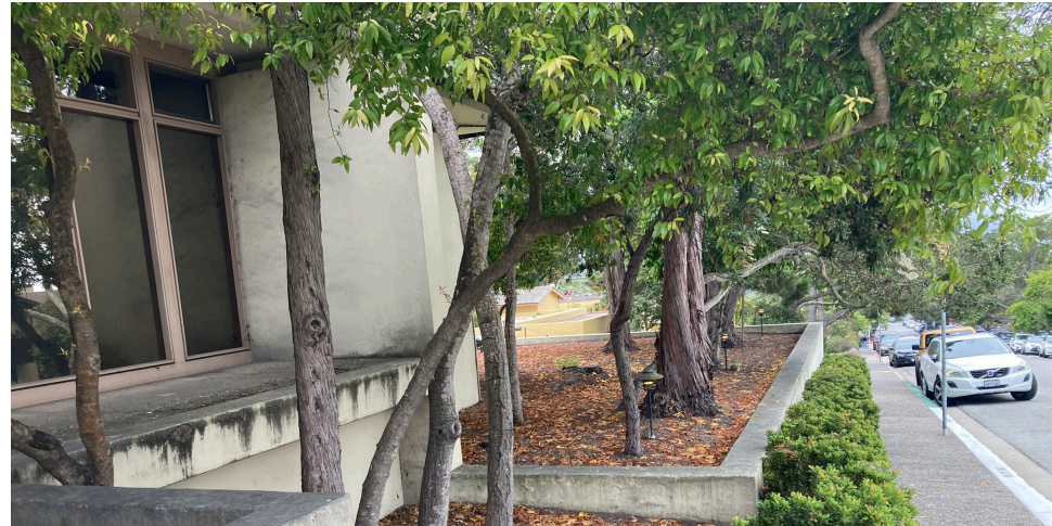
Unimpeded access to Police Building Windows from Junipero Street
