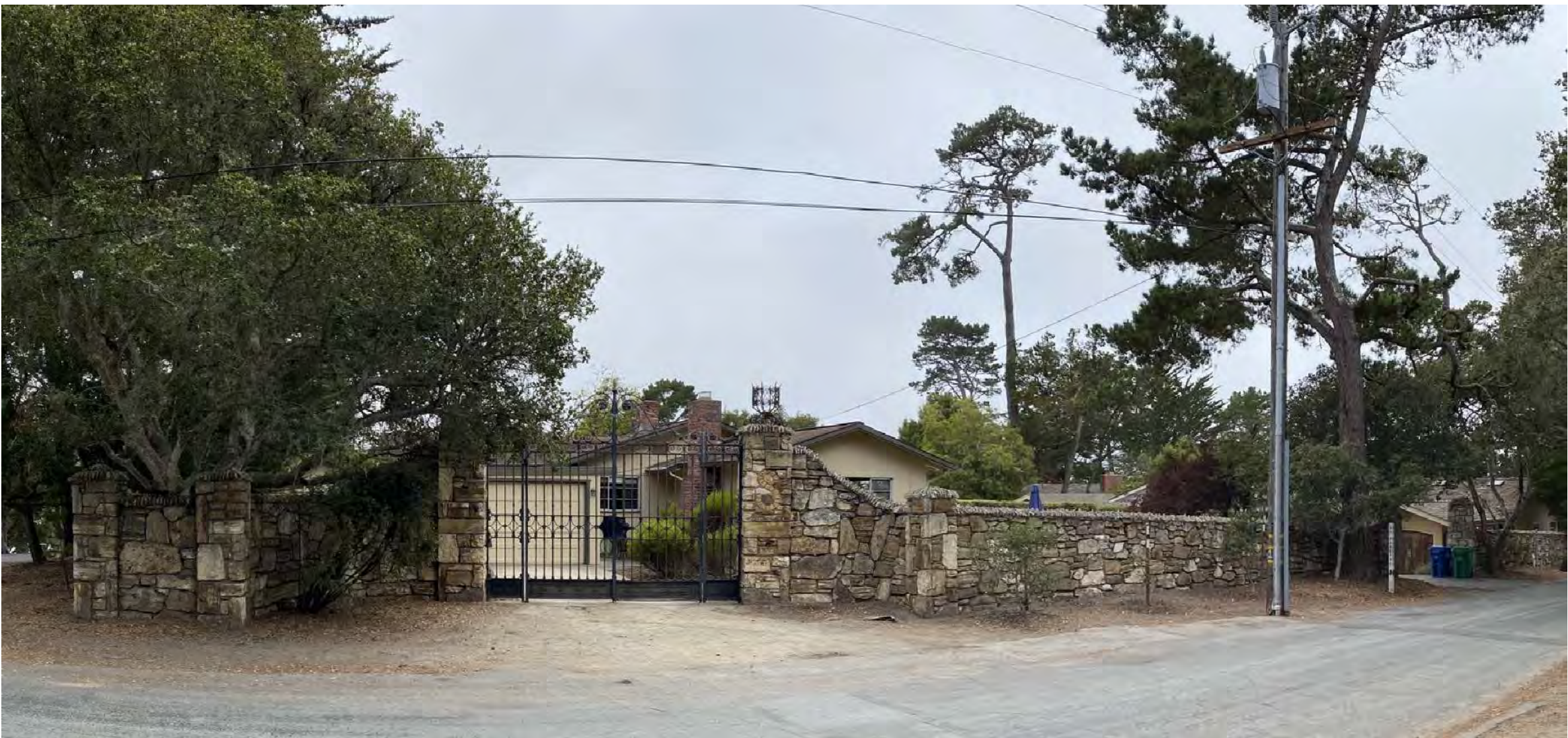
FRONT VIEW BEFORE
