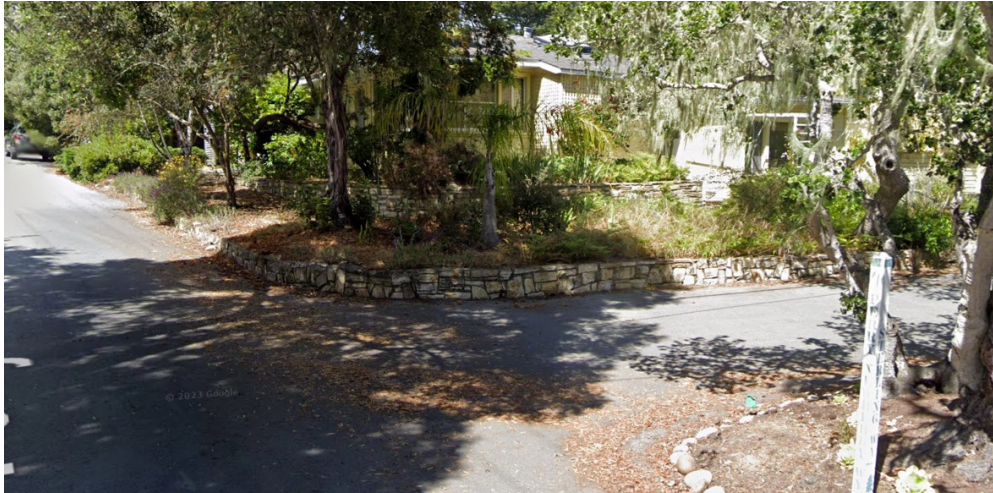
Figure 6. Existing right-of-way. Subject encroachment is lower wall. Property line is located at upper wall terrace (refer to Figure 5). As such, staff has included Condition of Approval for concept acceptance #4 stating that prior to scheduling for final details review, the applicant shall revise the proposed plans so the existing right-of-way encroachments are proposed for removal as part of the project, as well as a right-of-way improvement plan (ex. landscaping) be included in the submittal to be reviewed at the Final Details Hearing.
