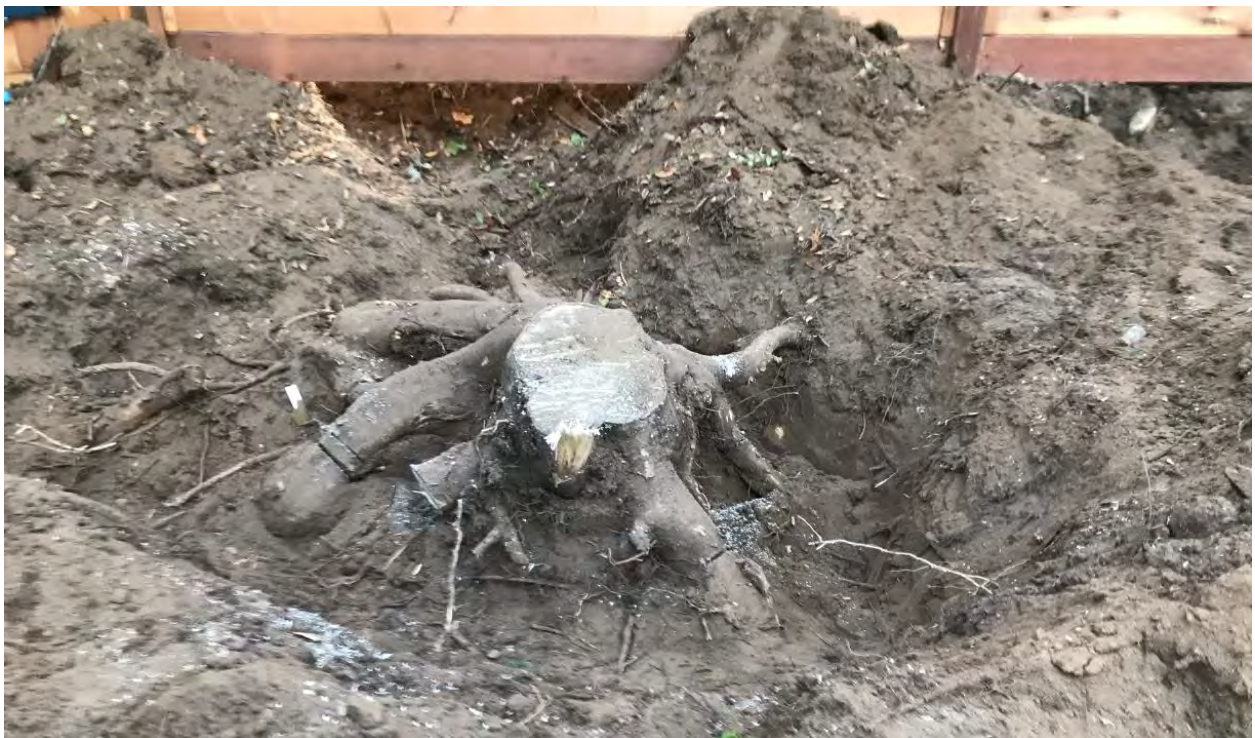
Figure 3 Stump excavation
