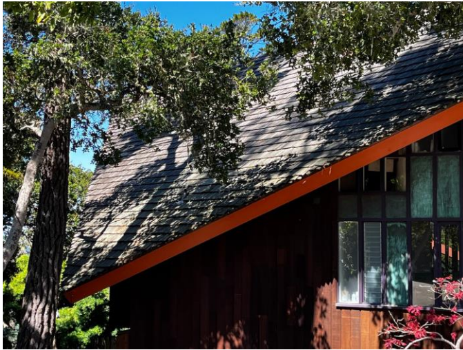
Replace Roof Shakes
