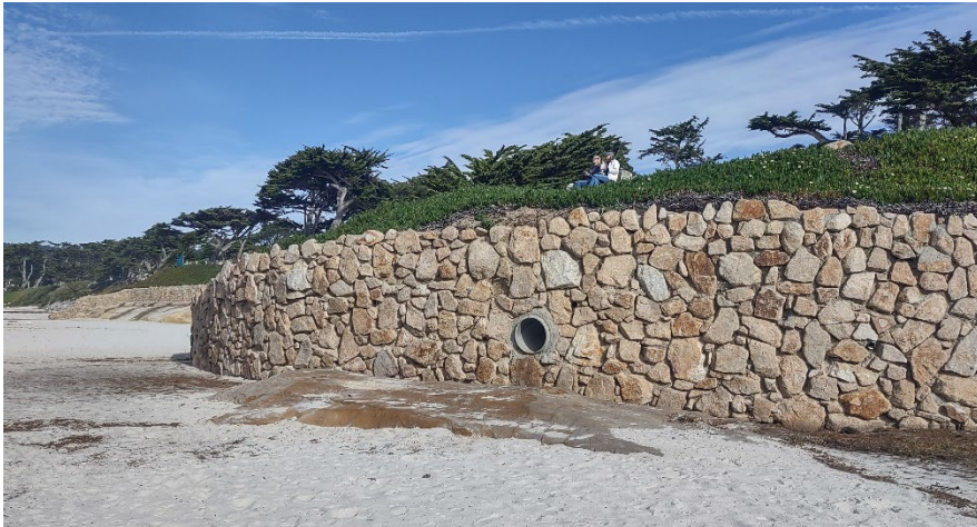
Figure 20. Stormwater drainage near 13th Avenue.
