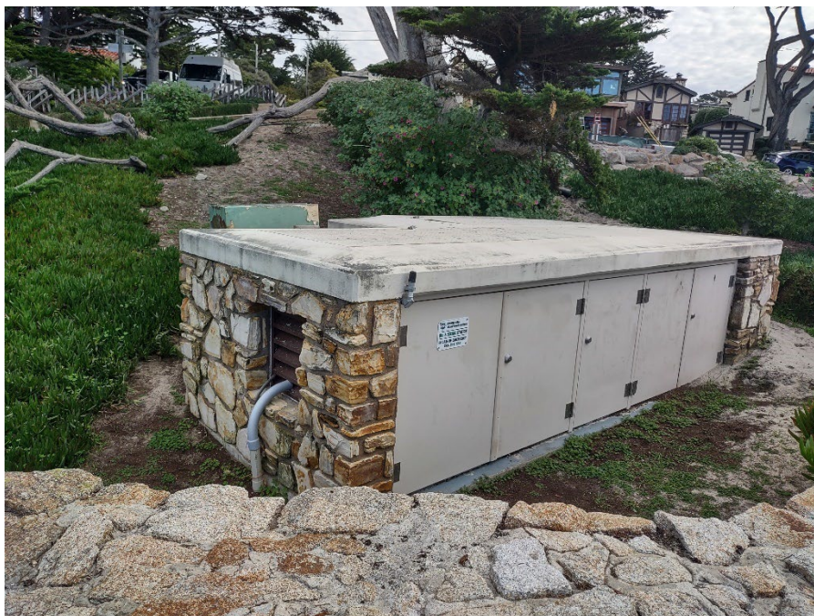
Figure 24. Wastewater lift station near 8 th Avenue.
