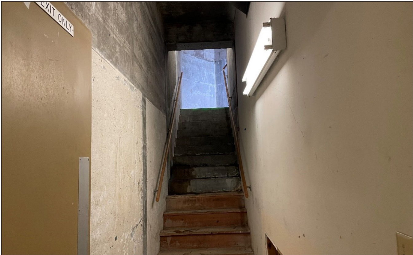
Structural Figure 8: Basement Entrance
