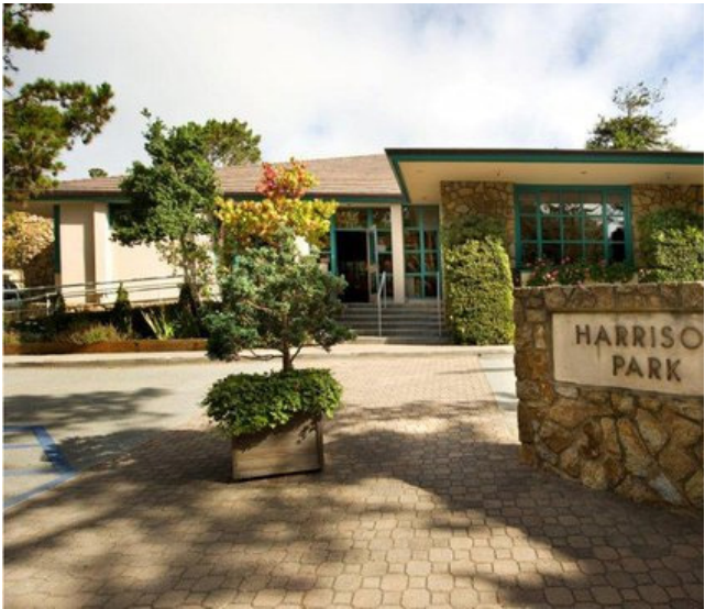
Architectural Figure 3: Existing Library - Exterior
