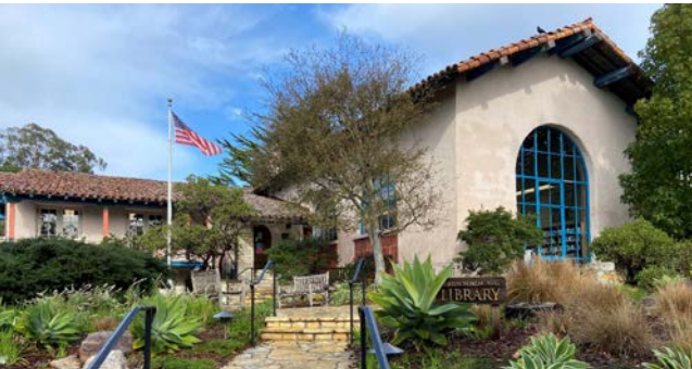
Architectural Figure 1: Existing Library - Exterior
