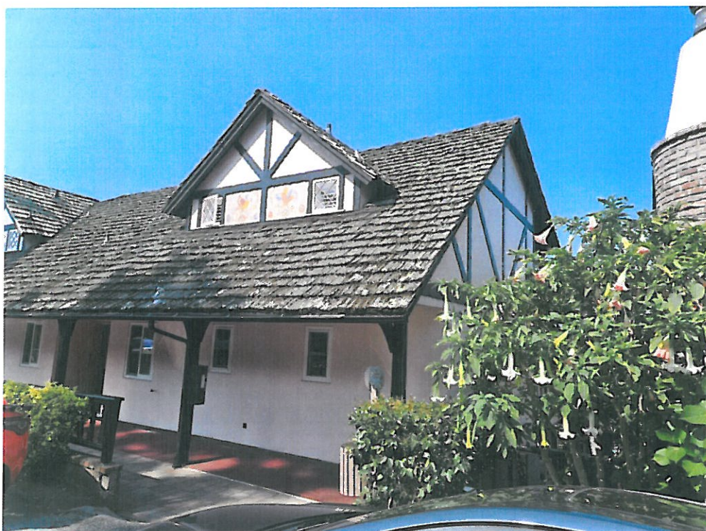
Figure 3: North wing looking southwest from San Carlos Street.
