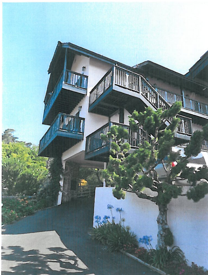
Figure 8: Rear elevation of North Wing, built in 1968.
