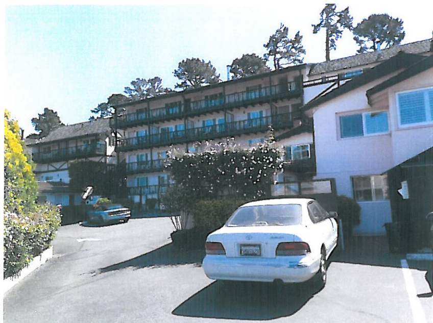
Figure 7: Rear elevation of 1957 hotel looking northeast.
