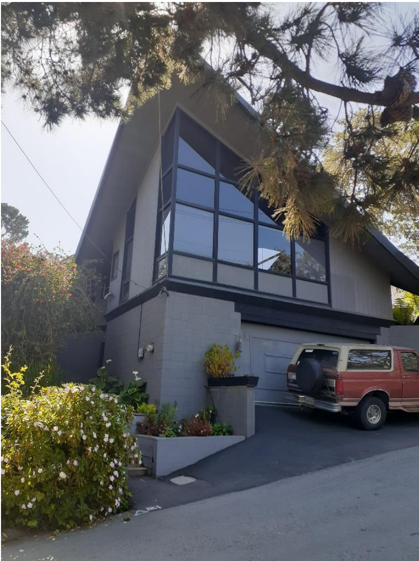
Figure 1: Front elevation looking southeast
