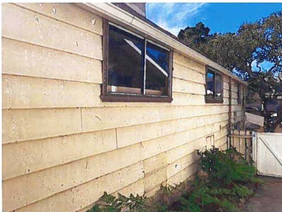
North elevation, looking west.
