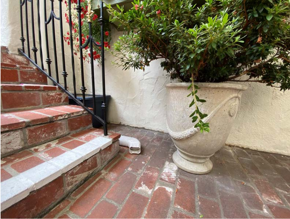
Photo 16, temporary surfact drainage at courtyard
