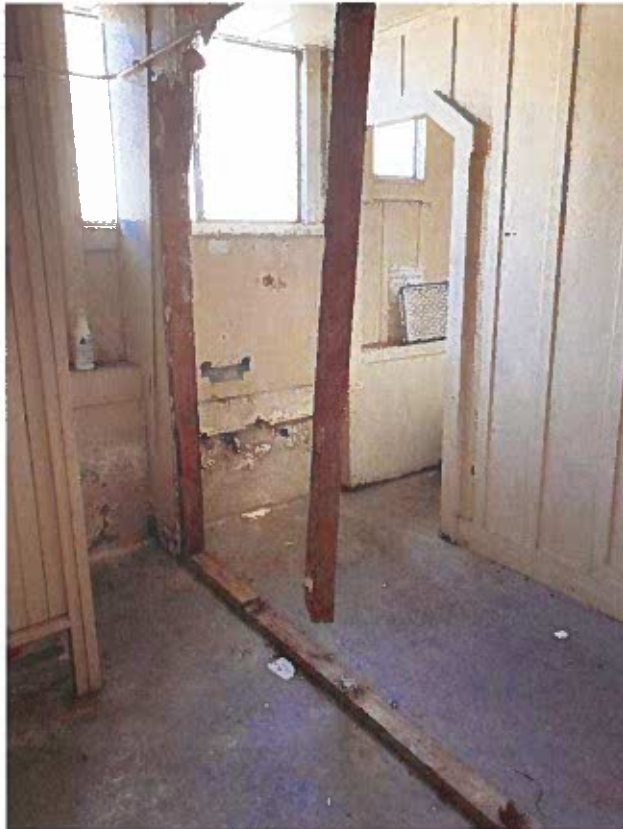
Downstairs restrooms, envisioned to be completely reconstructed
