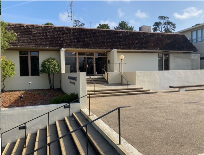
Police Building Renovation
