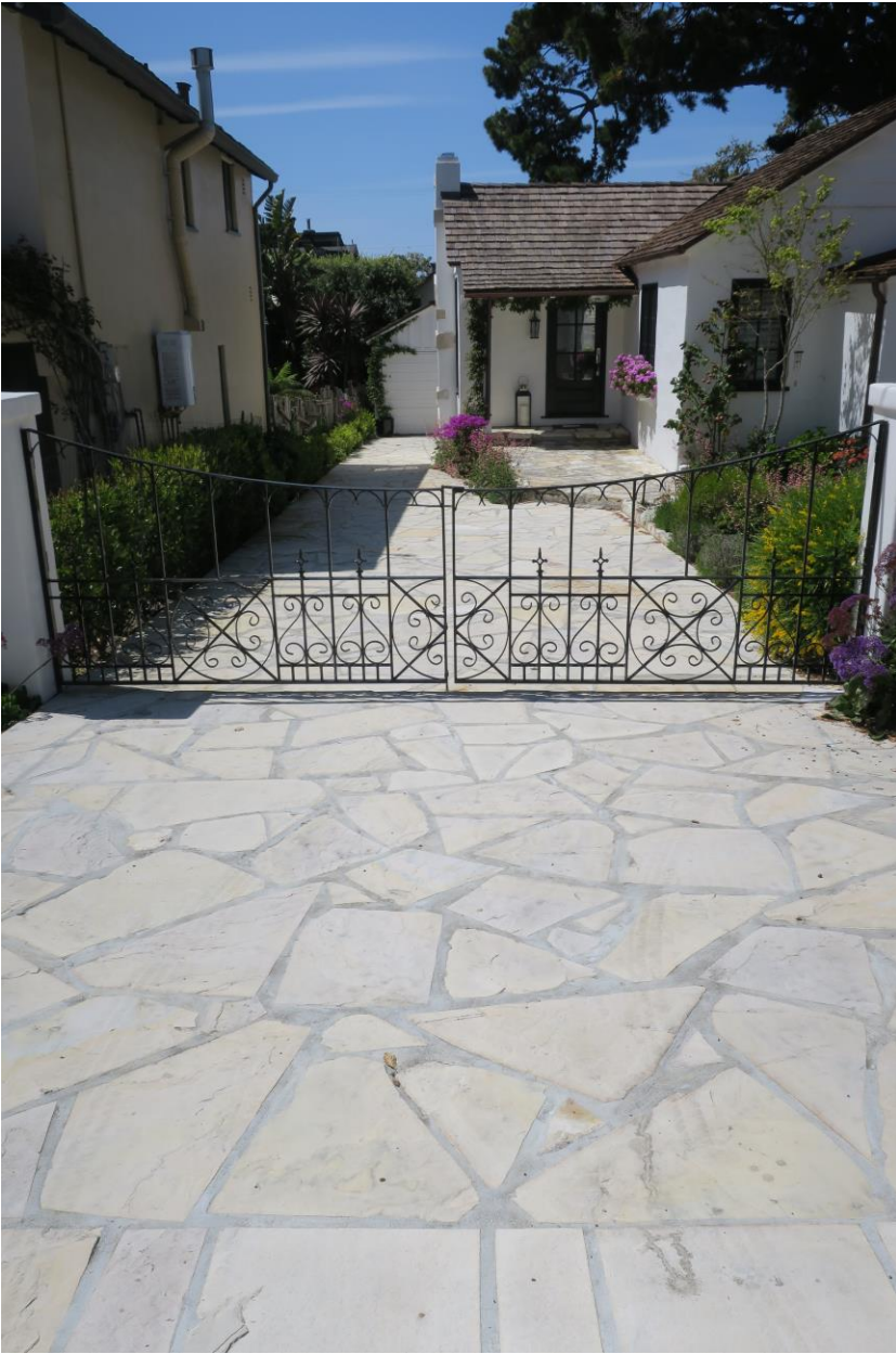
Unpermitted mortared stone driveway and driveway gate.
