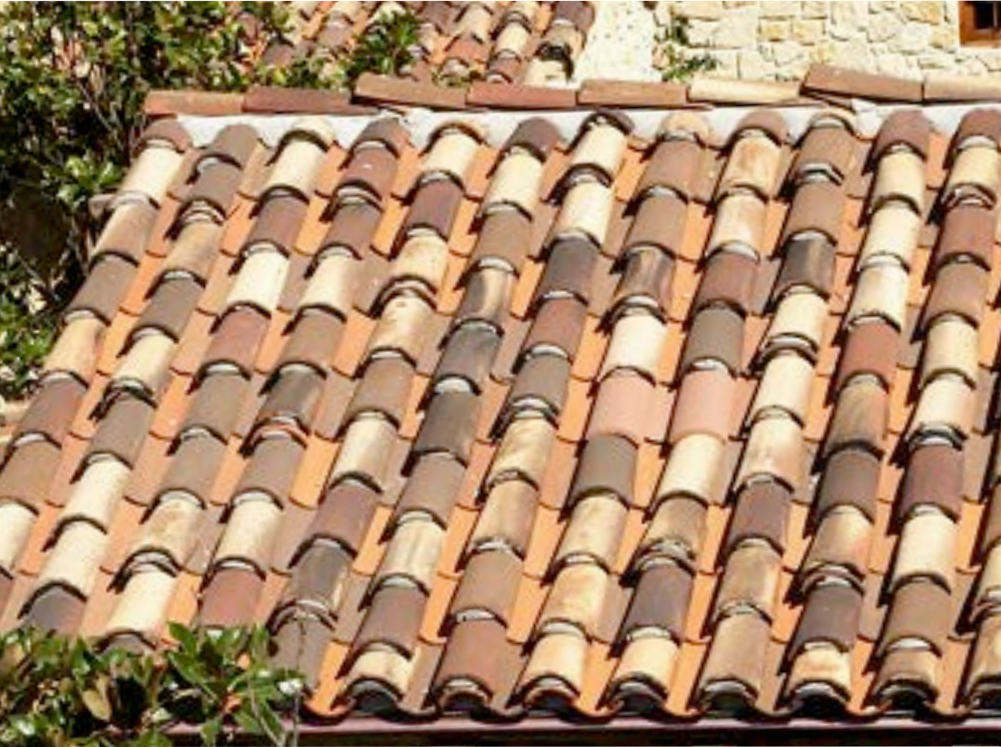
Roofing Two-Piece Mission Clay Tile Redland Clay Tile
