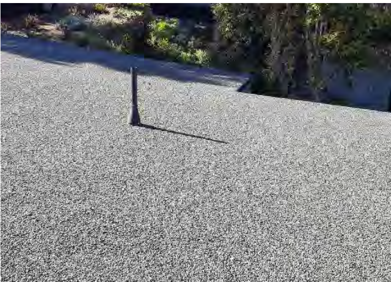
7.20 - PVC LOW SLOPE ROOF - COVERED WITH GREY PEBBLES (EPOXY ADHERED)
