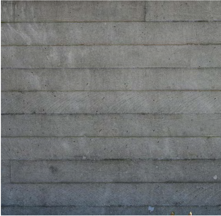
3.10 BOARD FORMED CONCRETE WALLS
