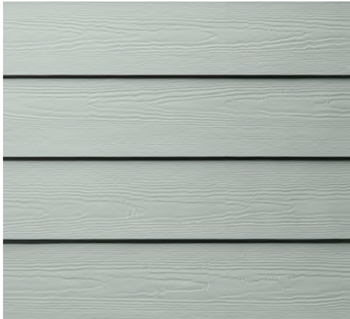
PLANK SIDING HARDIPLANK COMPOSITE HORIZONTAL SIDING PAINTED PEDIMENT 1ST FLOOR OF HOUSE
