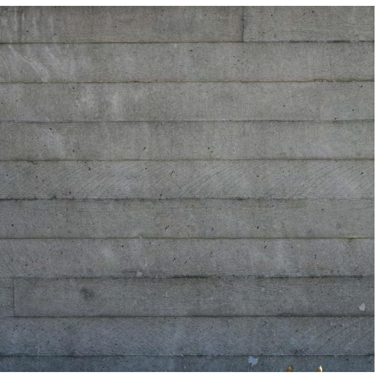
3.10 BOARD FORMED CONCRETE WALLS
