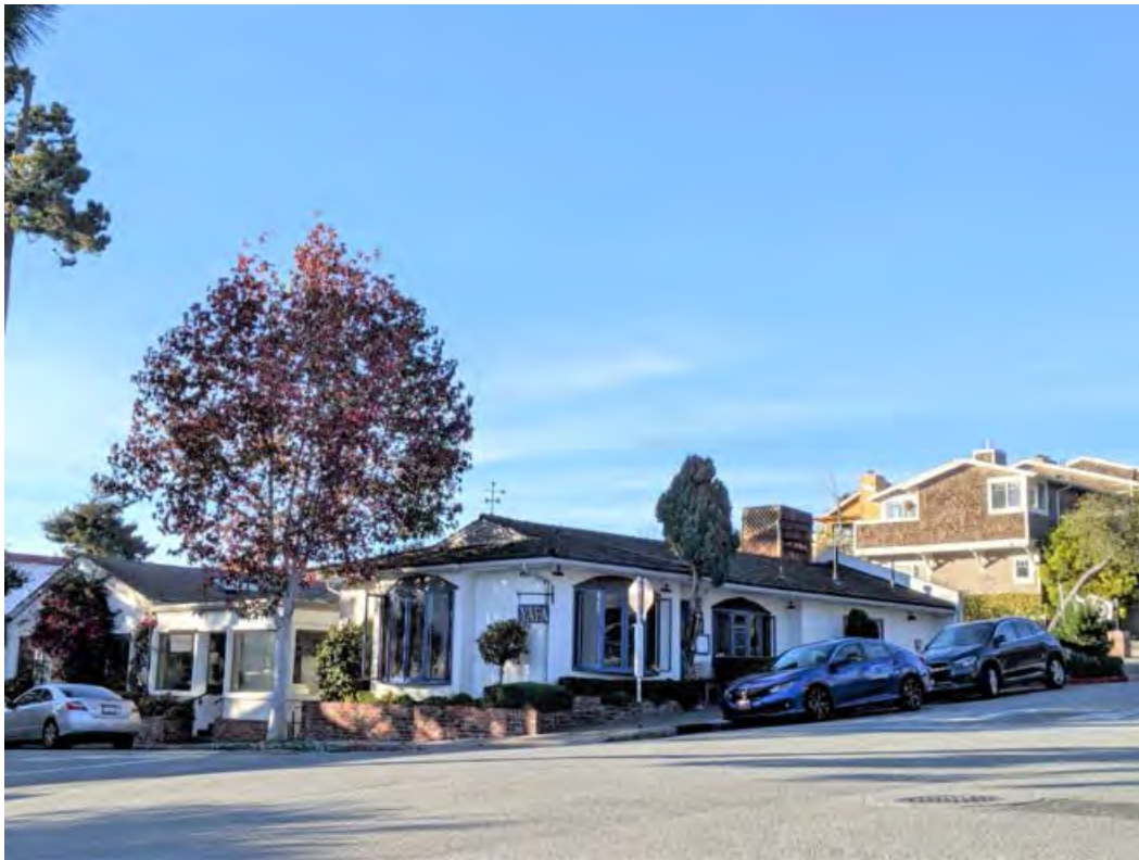
Figure C-17 5 th and Juniper Site (Site #16)
