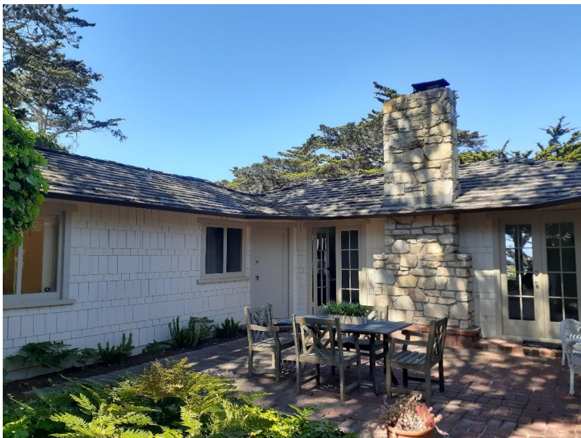
Figure 1: View of back patio, looking SW
