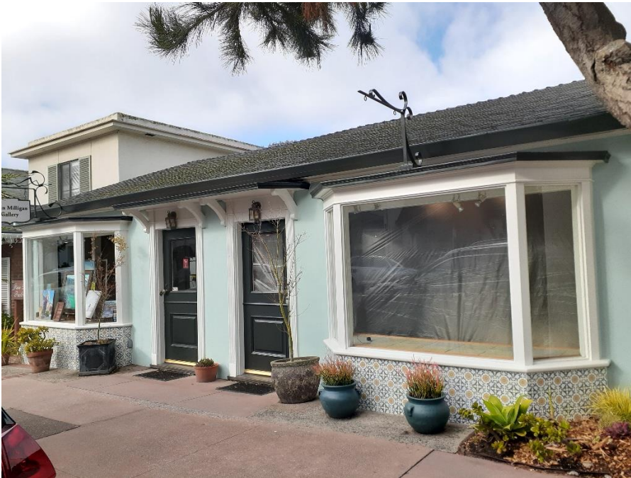
Figure 1: View of 1937 building (Building #1) looking southwest
