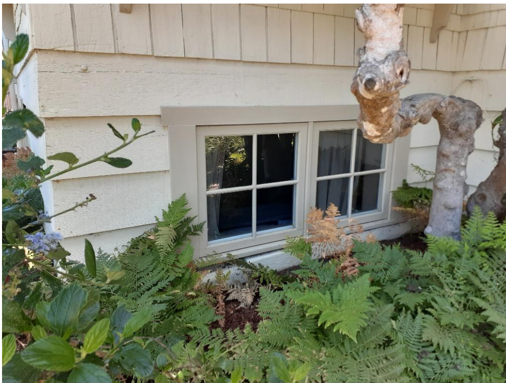
Figure 4: Basement windows on south elevation
