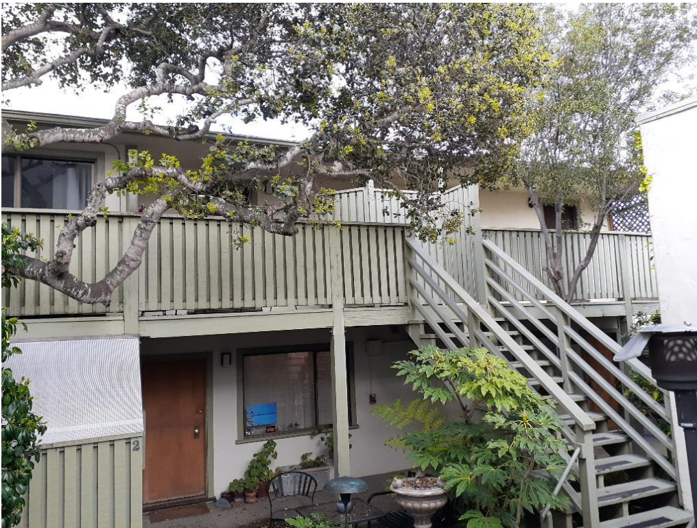
Figure 4: Northwest view of apartment building (Building #4) behind commercial block
