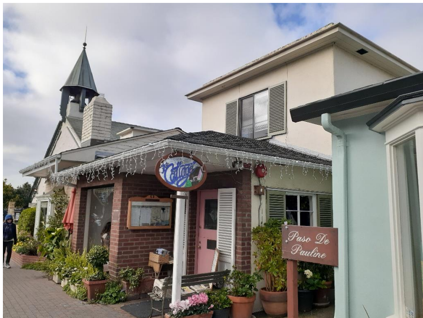
Figure 2: View of 1938 building (Building #2) looking southwest
