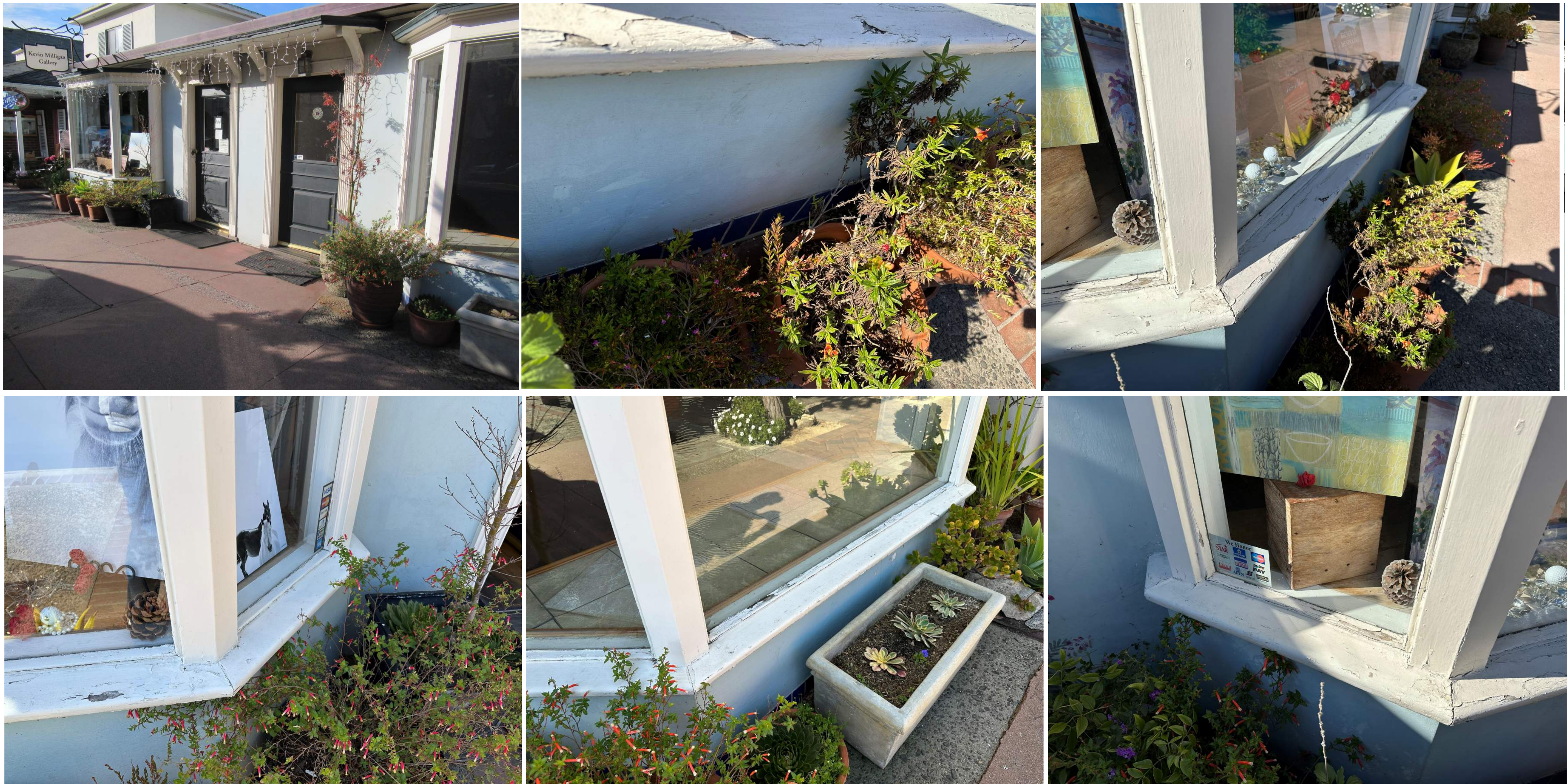
PHOTOS OF EXISTING CONDITIONS
