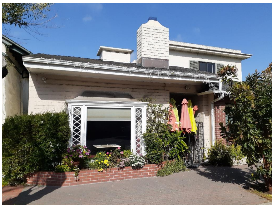
Figure 3: View of 1941 building (Building #3) looking west
