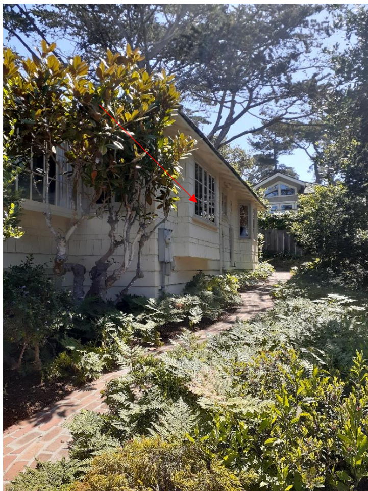
Figure 3: Arrow indicates location of new entrance.
