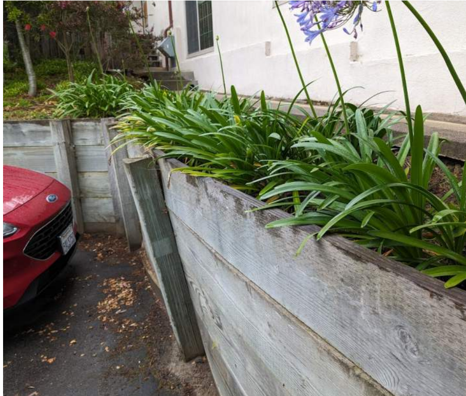
Figure 25 – Wood Retaining Help
