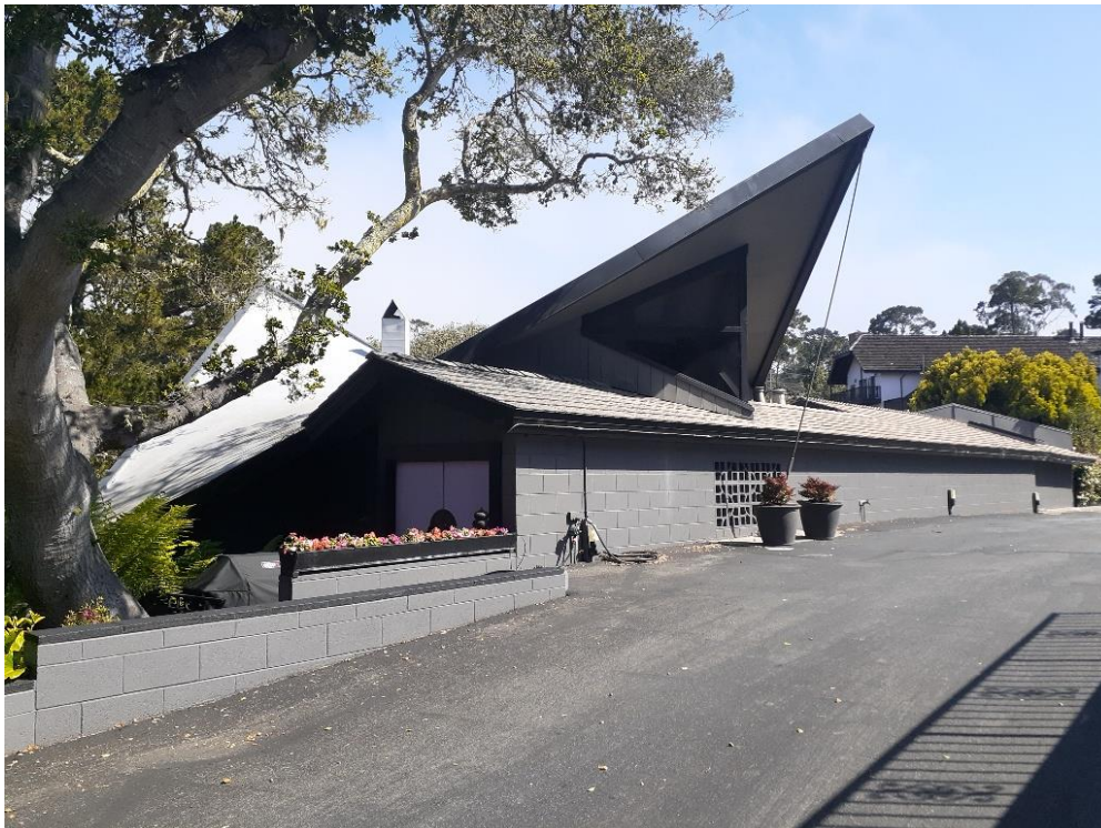
Figure 2: View looking northwest
