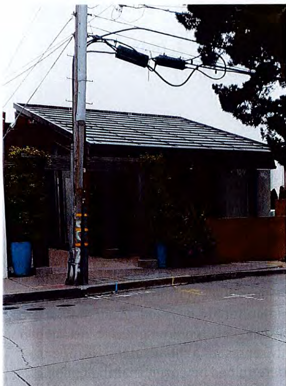
Front Elevation Facing Dolores Street, 2020
