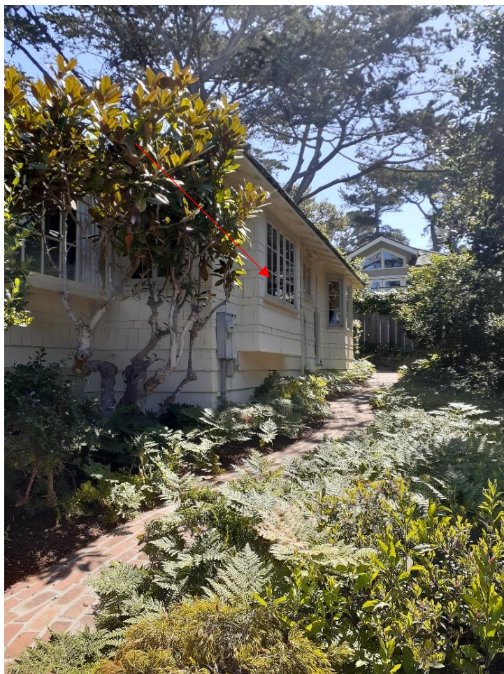
Figure 3: Arrow indicates location of new entrance.
