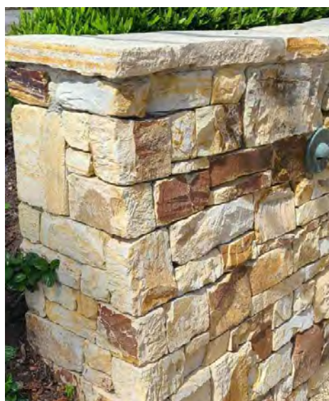
NEW STONE AT ENTRY COLUMN / GARAGE
