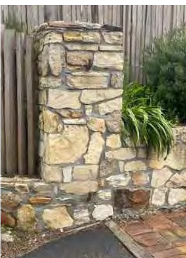
EXISTING CARMEL STONE AT RETAINING WALL DRIVEWAY
