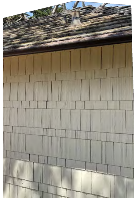
EXISTING WOOD SHINGLES / ROOF SHAKES
