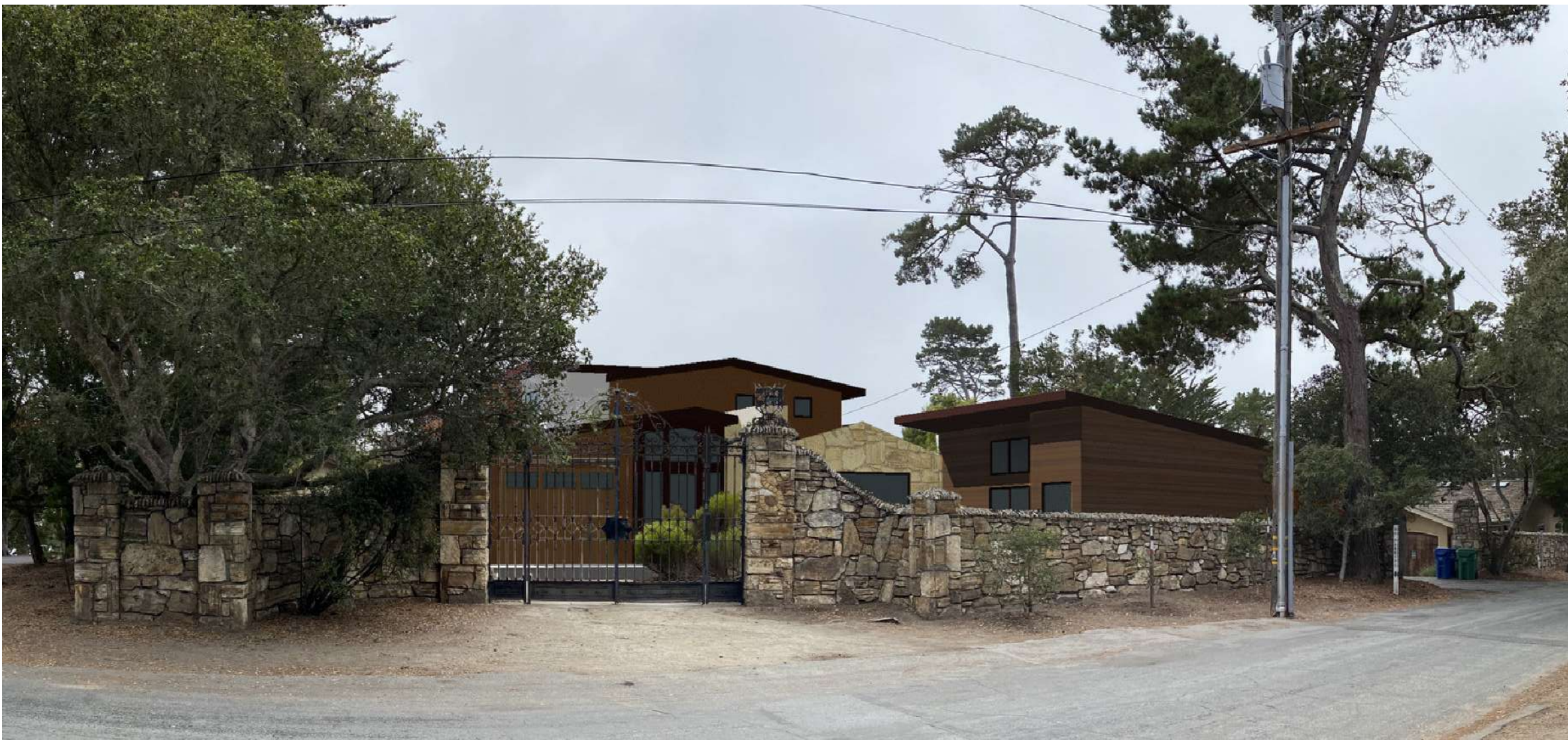
FRONT VIEW AFTER
