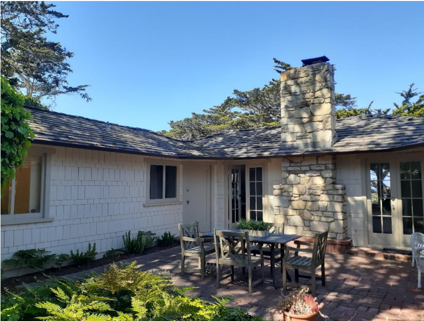
Figure 1: View of back patio, looking SW
