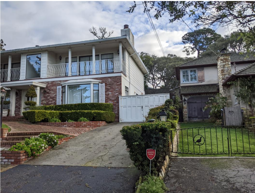
Figure 5: Neighboring property to the north (image left) and subject property (image right).
