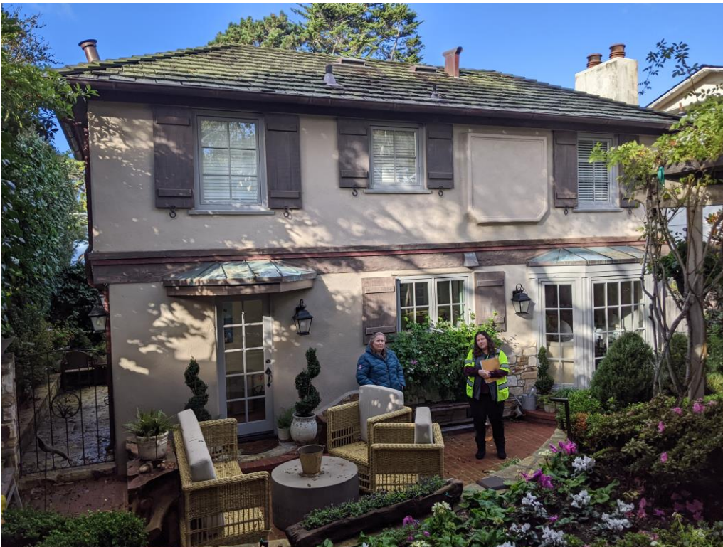
Figure 11: Rear elevation, looking west.
