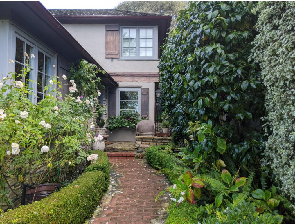
Figure 10: Detail of south portion of existing residence, looking east.
