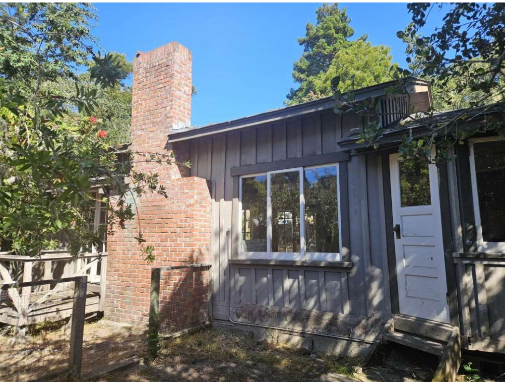
Figure 4: View of rear elevation looking northeast.
