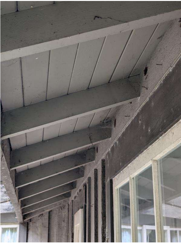
Detail photo of exposed rafters typical of the north and south wings.
