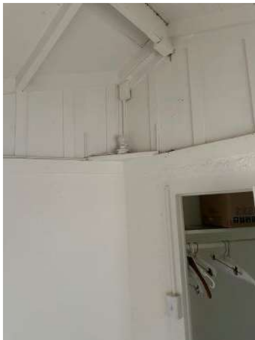
Figure 16 Stucco on interior walls and exposed wiring
