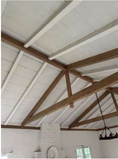
Figure 5 Roof framing in main room
