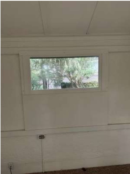
Figure 18 Stucco interior walls at modified window
