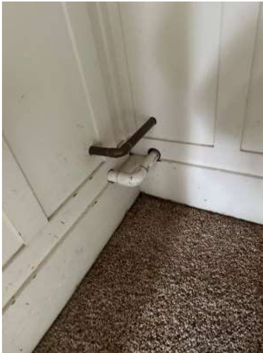
Figure 14 Surface run plumbing in bedroom
