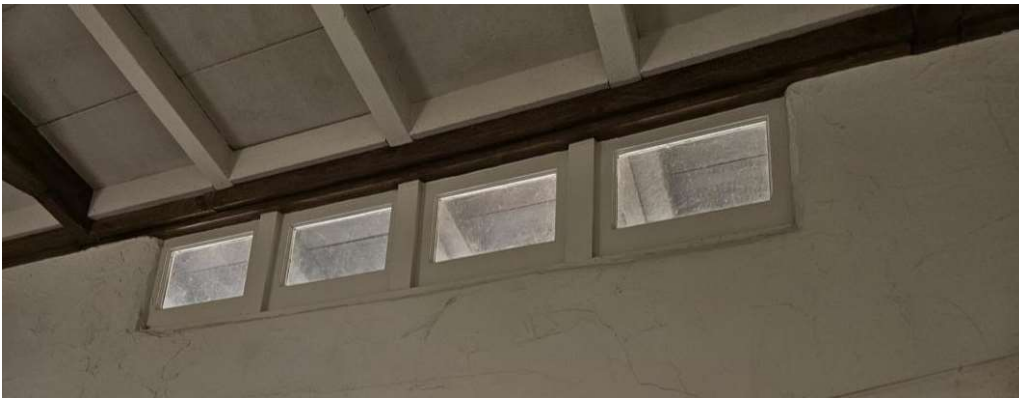
Figure 3: Interior view of fixed clerestory windows.
