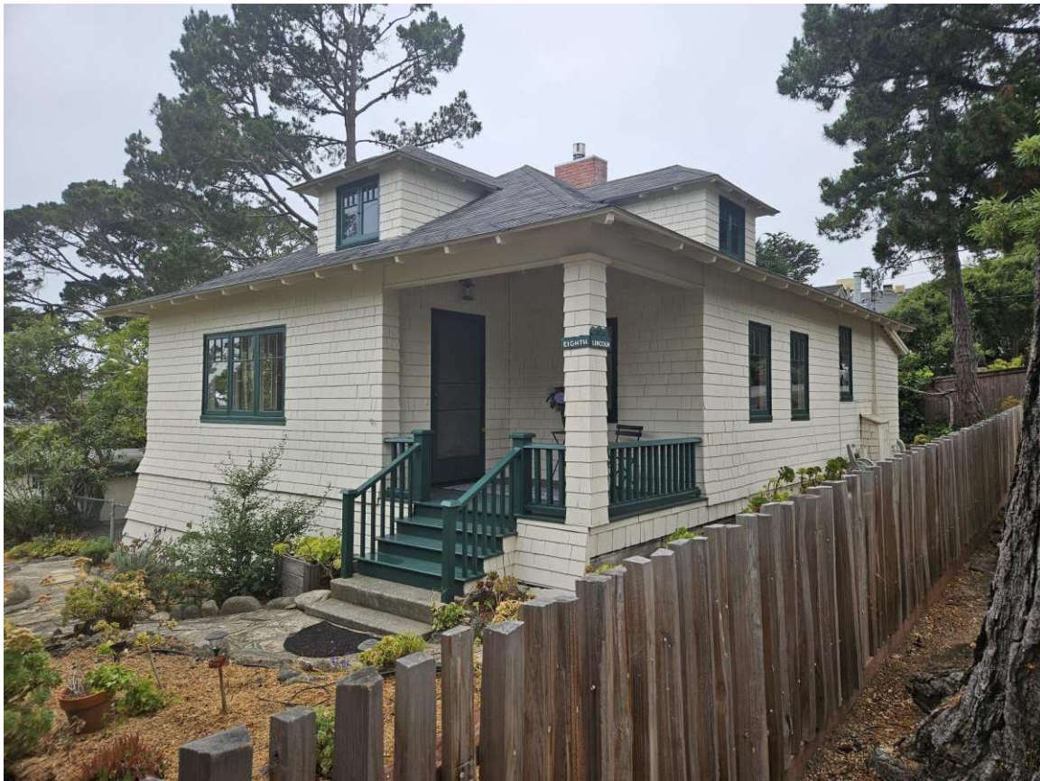
Front elevation looking northwest.
