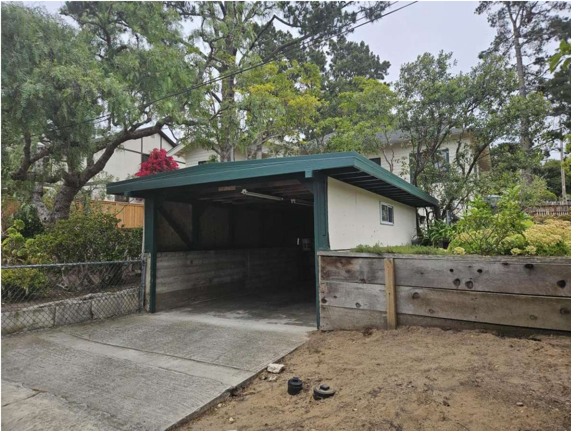
Figure 7: View of carport looking northeast.
