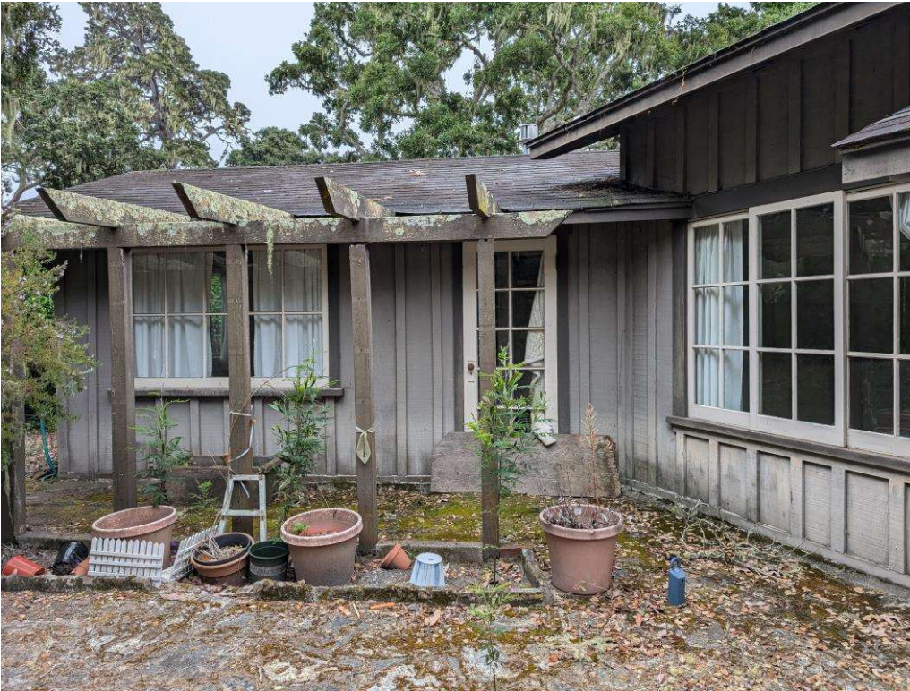
South wing, looking south. Window at image left are fixed, whereas window at image right is a tripartite sliders.
