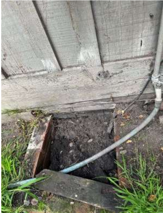
Figure 3 Top of foundation below grade
