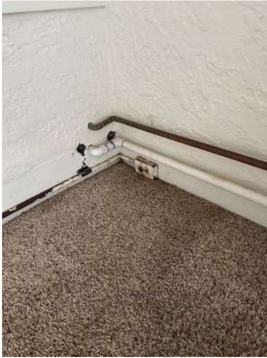
Figure 13 Surface run plumbing and electrical in bedroom
