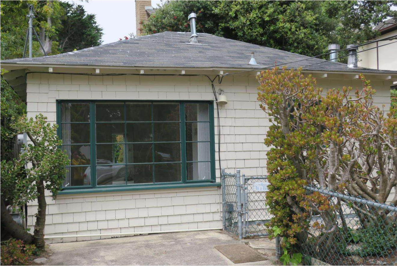
Detached guesthouse (former garage).
