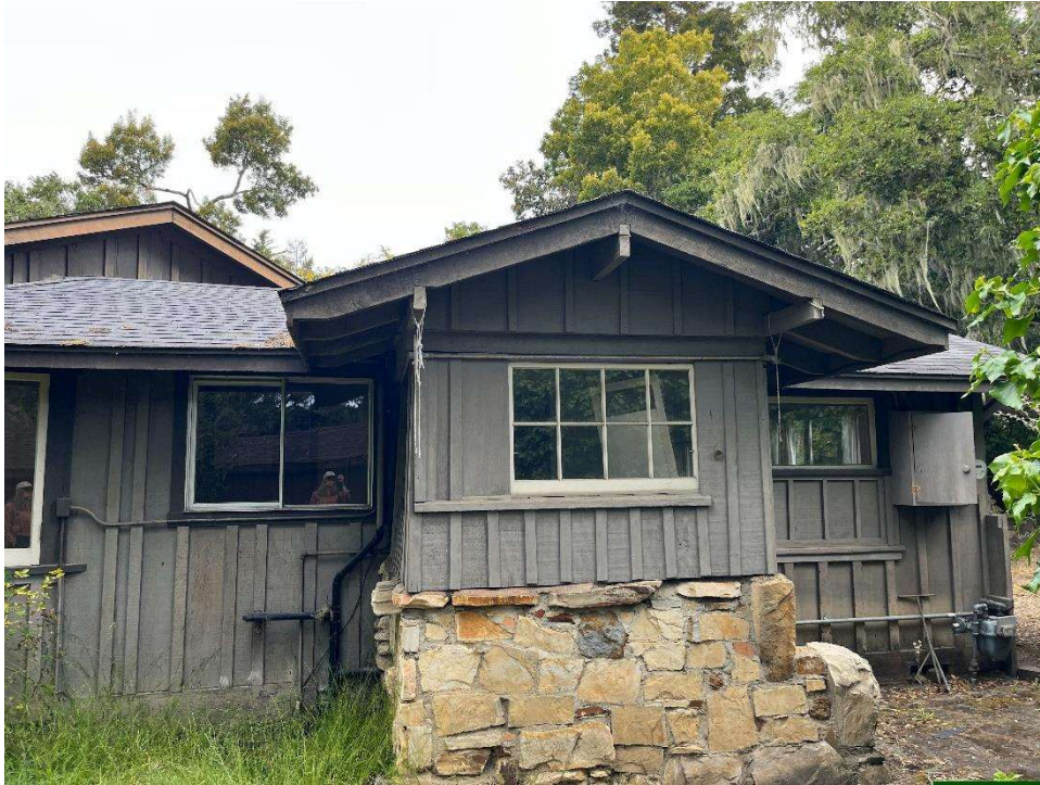
Photograph 5: Southeast elevation, showing small projecting volume with raised stone foundation. camera facing northwest.
