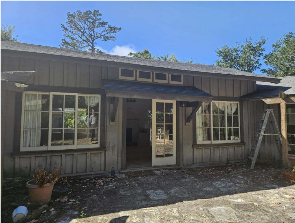
Figure 2: Front entrance with clerestory windows, French doors, and multi-paned wood sliding windows
