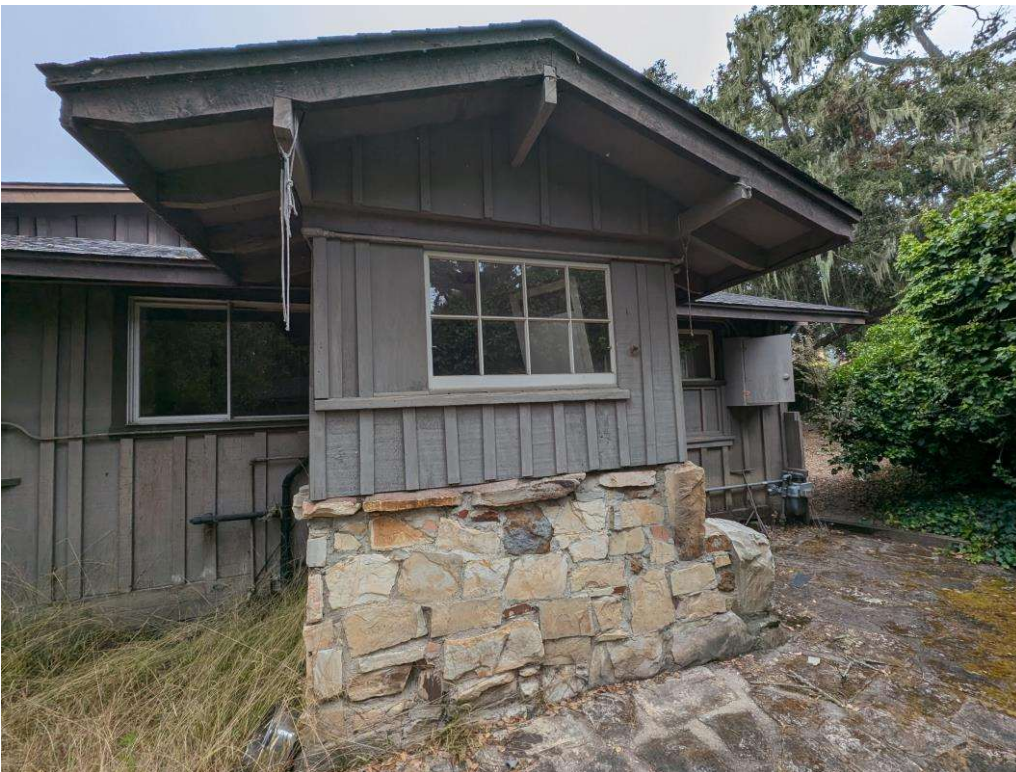
South wing service porch, looking northeast. Aluminum window at image left, and what appears to be a non-original or altered window opening in the foreground.
