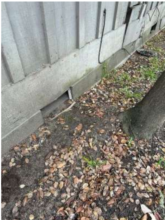
Figure 4 Foundation below grade
