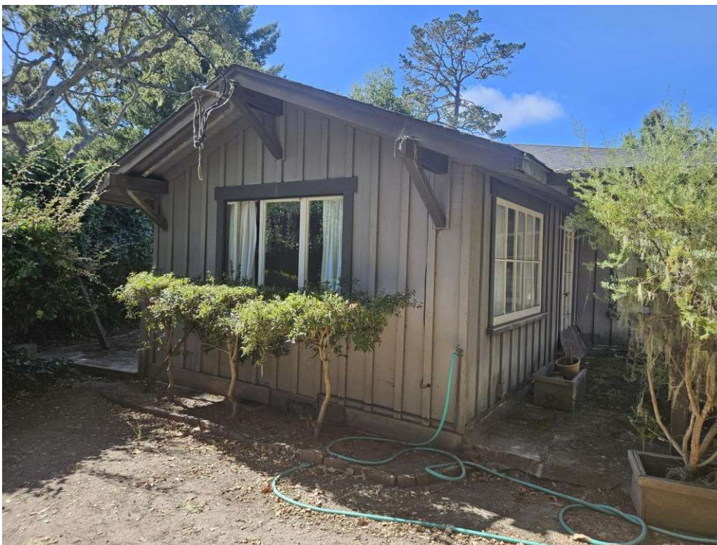
Figure 5: Knee brace brackets in south wing gable.
