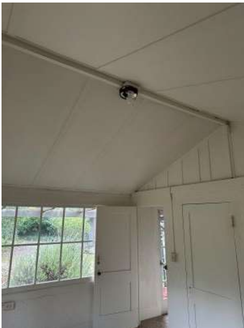
Figure 8 Bedroom ceiling with 2x6 ridge board and wood fiber insulation finish material
