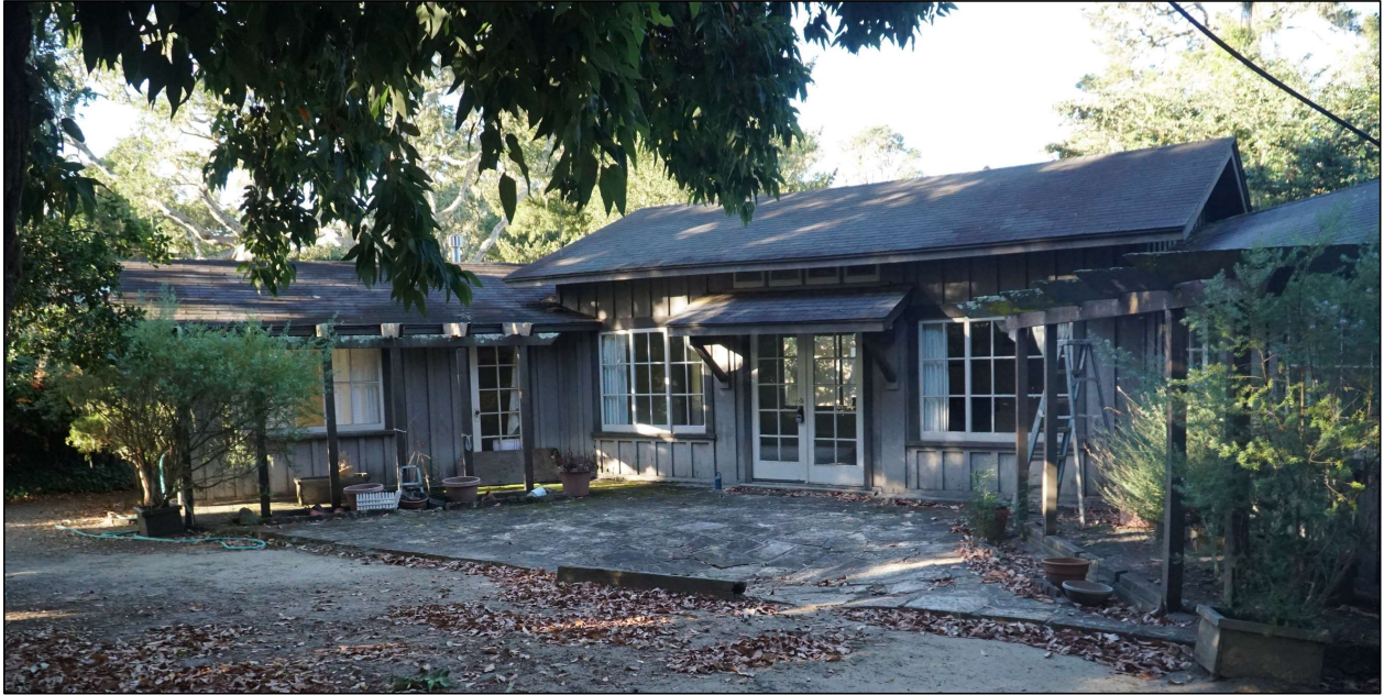
Figure 1. Looking west at east side and adjoining wings. The presence of subsurface water carrying soil away is evident at the front of the patio, directly below the two French doors.
