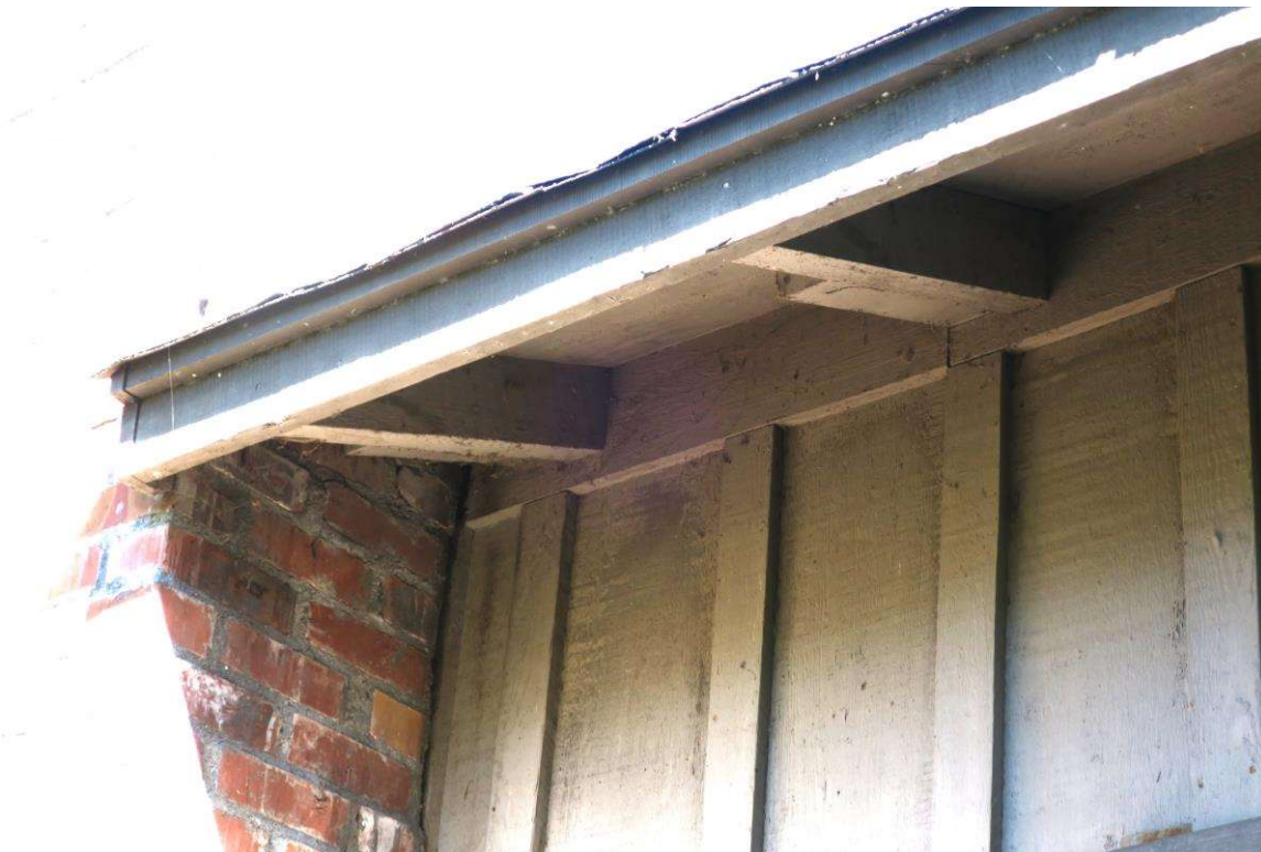
Detail of exposed rafters in the central volume. Note that the exposed rafter tails are truncated and have sistered extensions; this may reflect a construction error where the rafters used were simply not long enough to reach the fascia.
