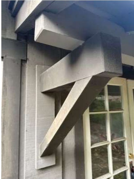
Figure 19 Knee brace at front entry
