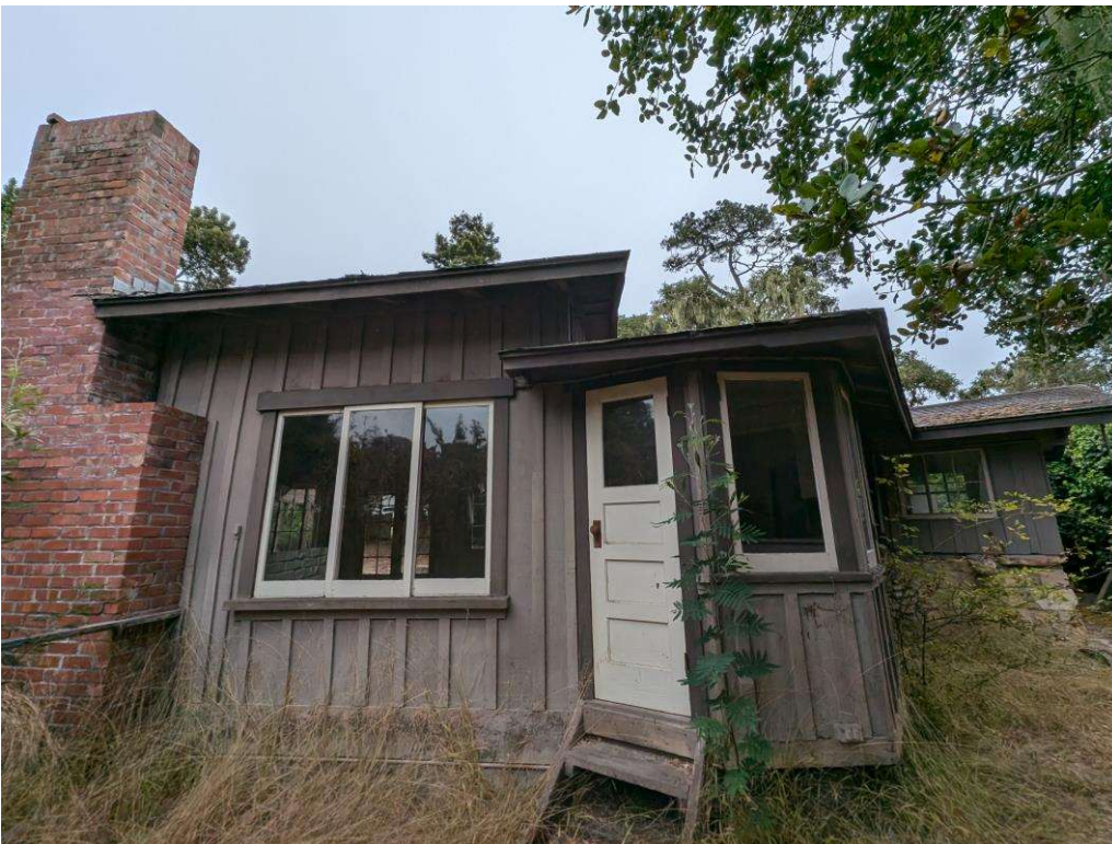
Rear (west) elevation, with exterior brick chimney at image left, pentagonal bay with casements at image center, and service porch image right.
