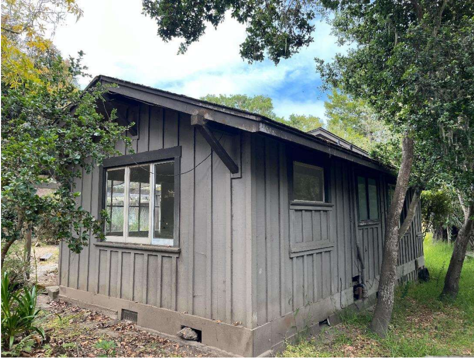
Photograph 3: Northeast (end) and northwest (rear) elevations showing single-light sliding wood windows, partially enclosed window openings, and aluminum sliding-sash, camera facing southwest.
