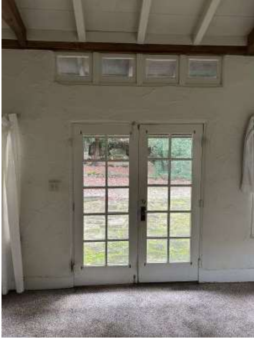
Figure 17 Heavily textured stucco walls in living room
