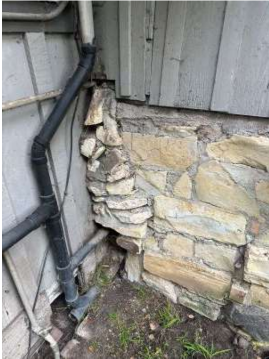
Figure 15 Surface run plumbing waste and gas lines
