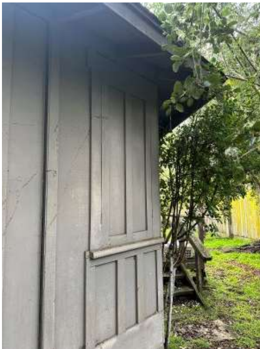
Figure 10 Former window filled in
