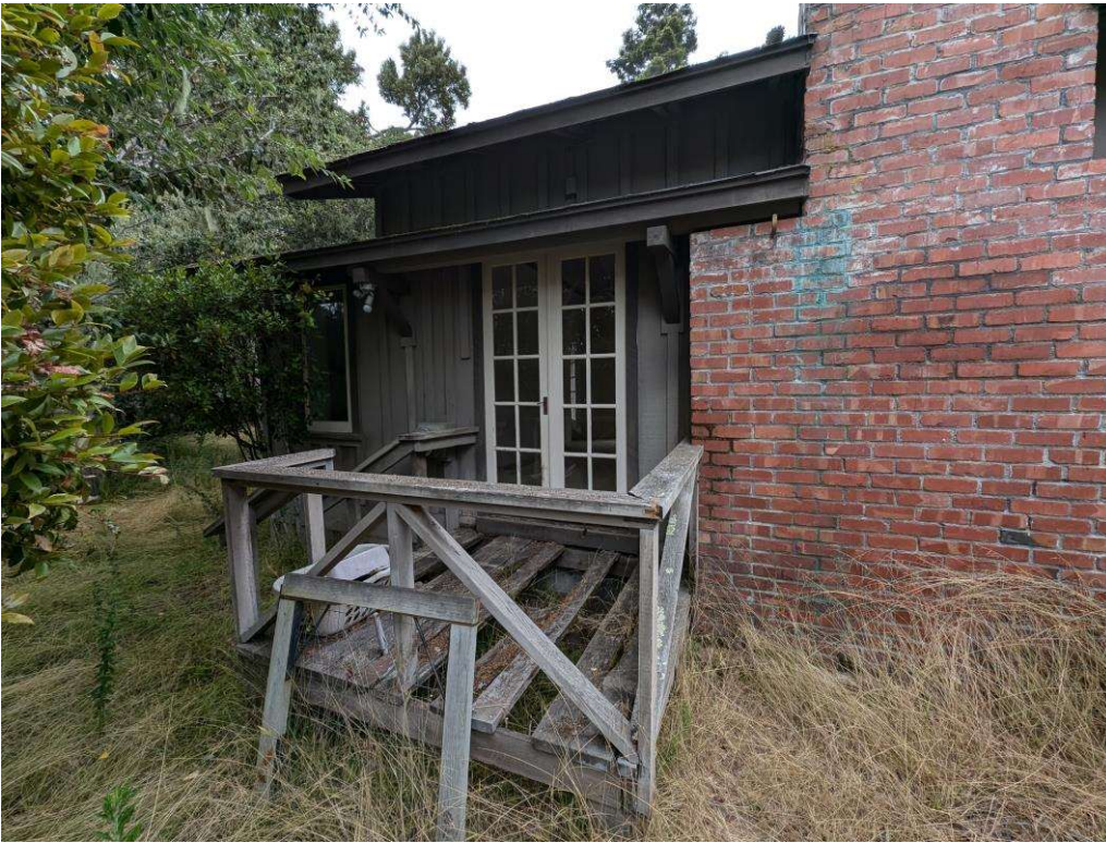
Rear (west) elevation with French doors and exterior brick chimney. Note the narrow shed roof supported by brackets, matching the design of the front entry doors.
