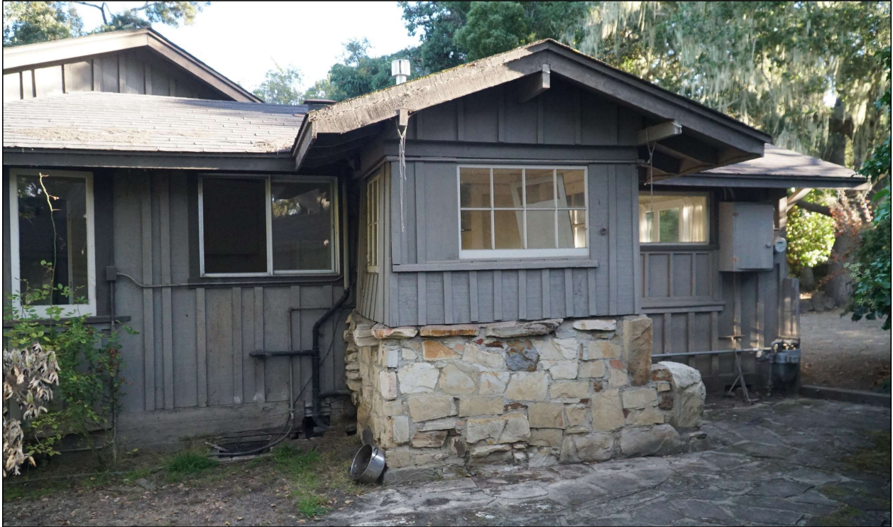
Figure 3. Looking north at a section of south side. The window above the rubblework is clearly not original, nor is the aluminum sliding-sash window is to the left of it.
