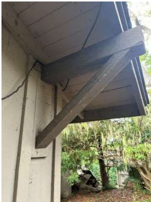
Figure 20 Knee brace at bedroom wing
