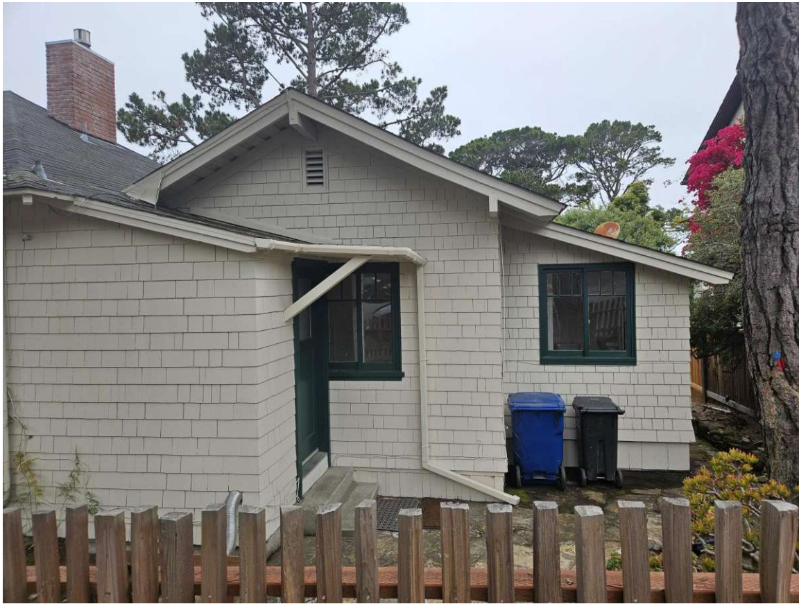
Additions at rear elevation, looking west.
