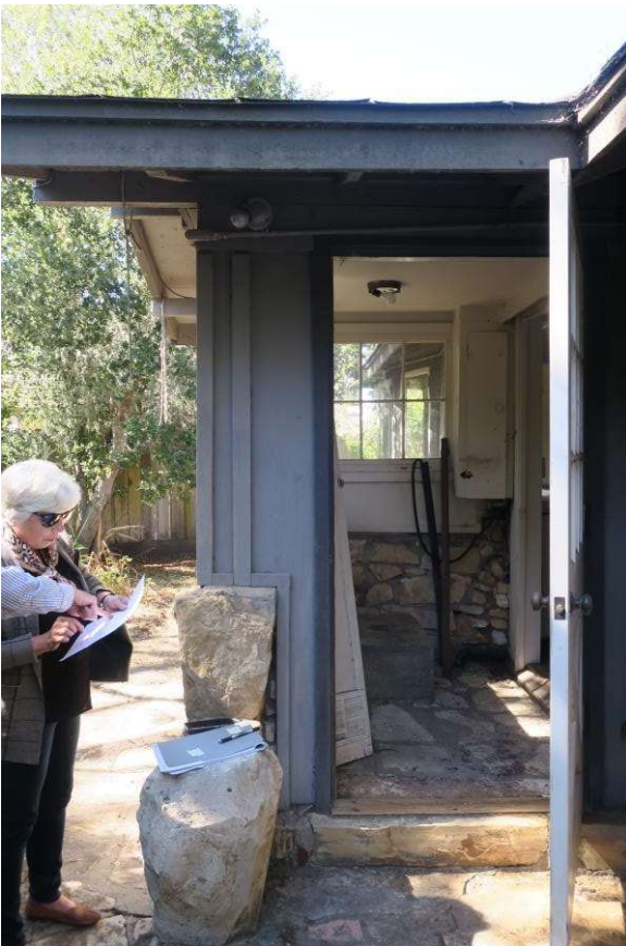
Service porch, with rubble stone base and what appear to be non-original window openings.
