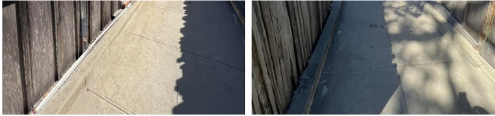
Figure 6. 12th Avenue Walkway - Existing Condition.
