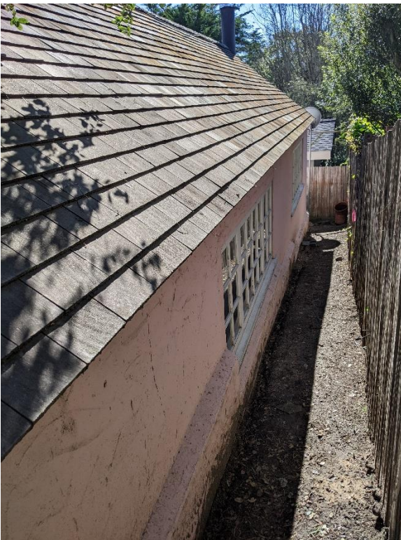
Figure 8: Rear (west) elevation, partially below-grade.
