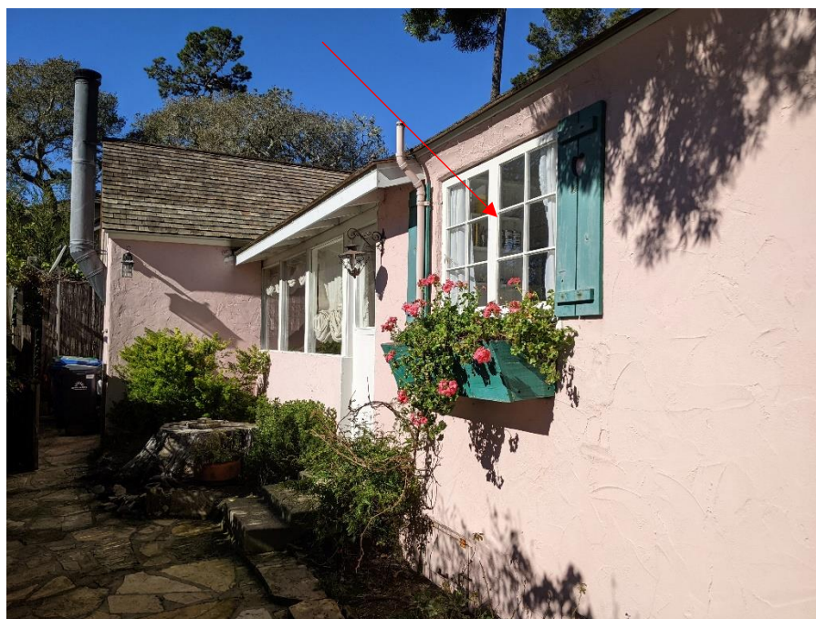
Figure 4: View of window on south elevation that will be shifted west.
