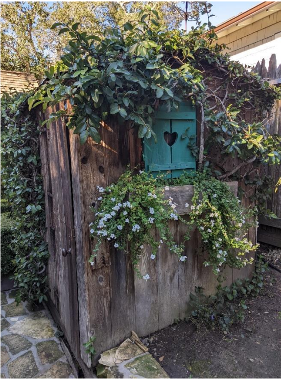
Figure 9: Non-historic shed to be demolished.
