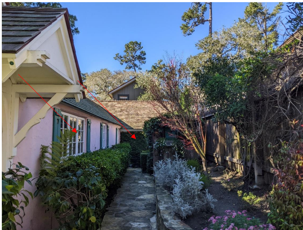
Figure 3: View of north elevation, location of bedroom addition and bank of windows that will be moved west.
