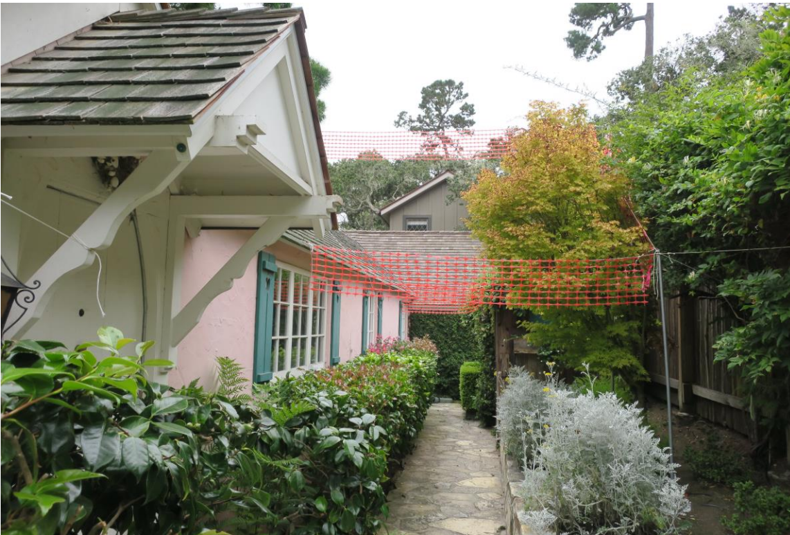
Figure 4: Storypoles for the proposed north bedroom addition, view looking west.
