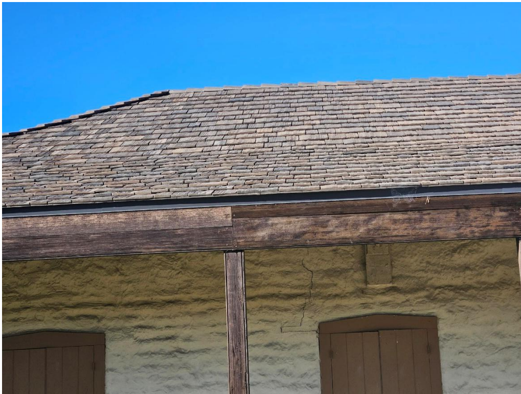
Figure 7: Simulated cedar shakes installed on the Boronda Adobe in Salinas.
