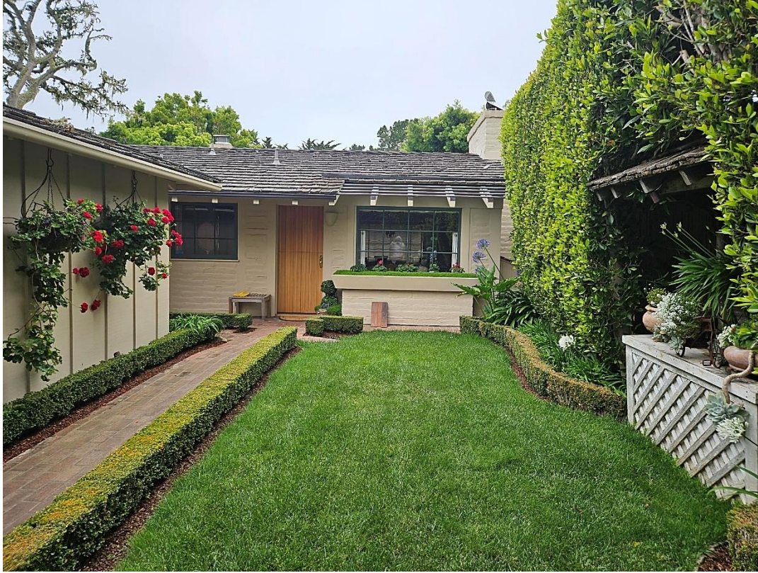
Figure 2: Front elevation, looking west from Carpenter Street.
