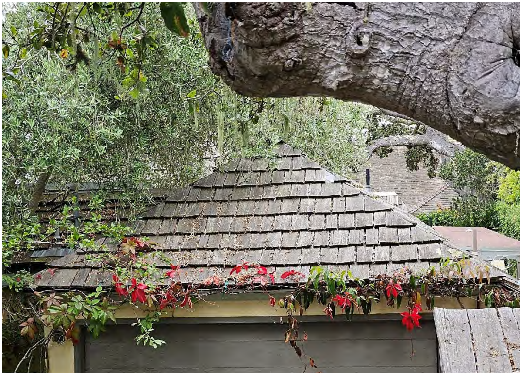
Figure 3: View of garage roof.
