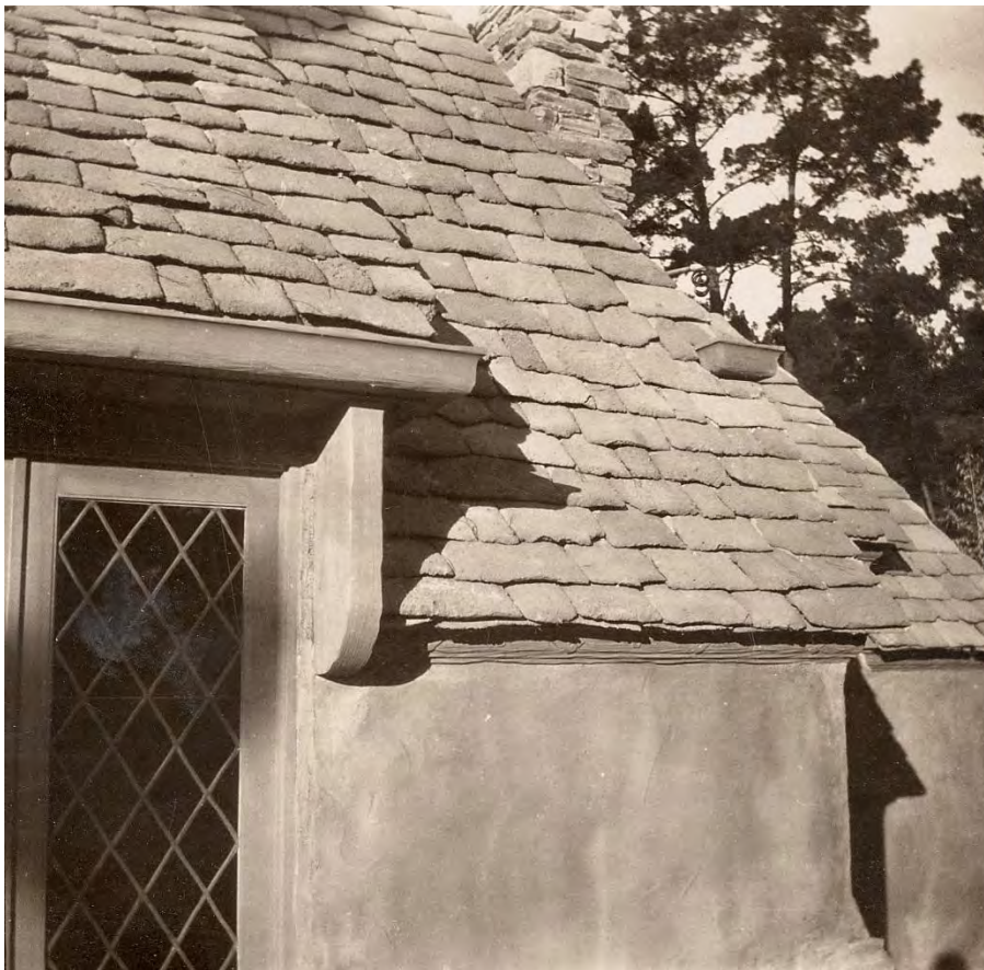
Figure 6: Original bubblestone roofing on the Comstock Studio. Courtesy of Roberta Voris, n.d.
