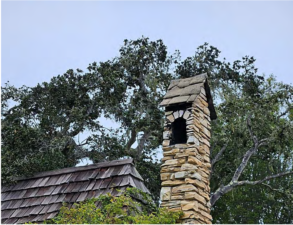
Figure 4: Bubblestone spark arrester.
