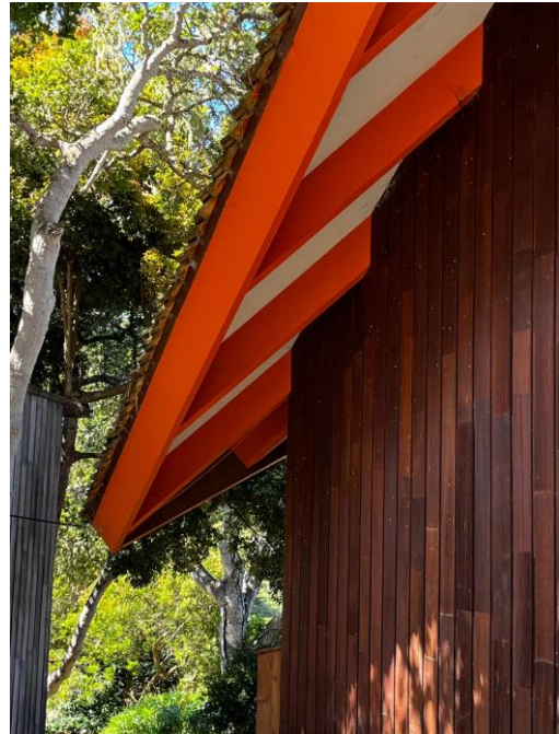
Paint Beams and Ceiling
