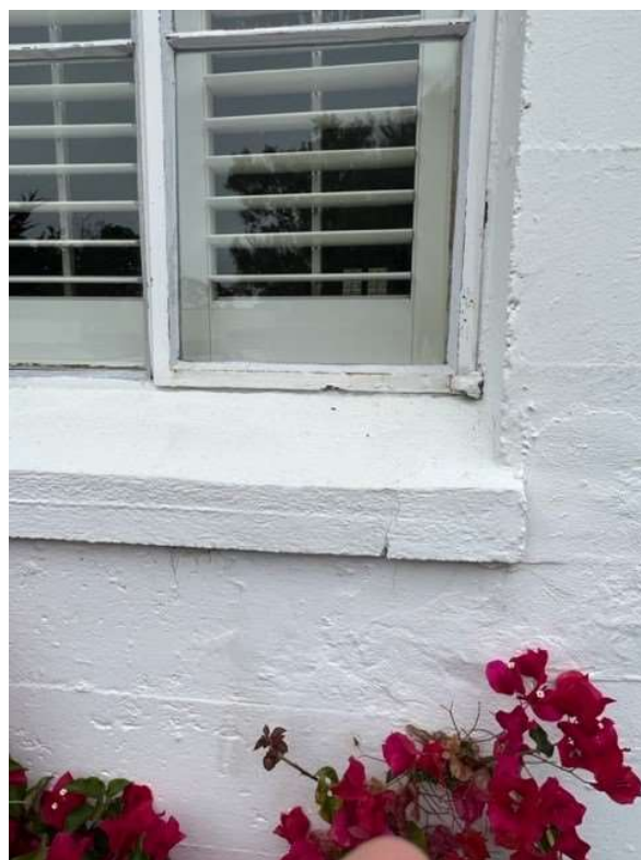
Photo #12, Typical deterioration of single pane metal window (View from 7 th Ave)
