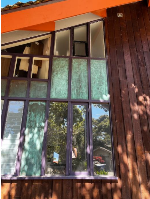
Paint Door and Window Trim
