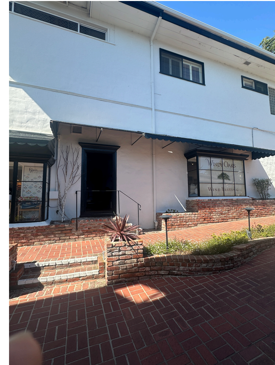
Existing Courtyard Entrance from Lincoln Street
