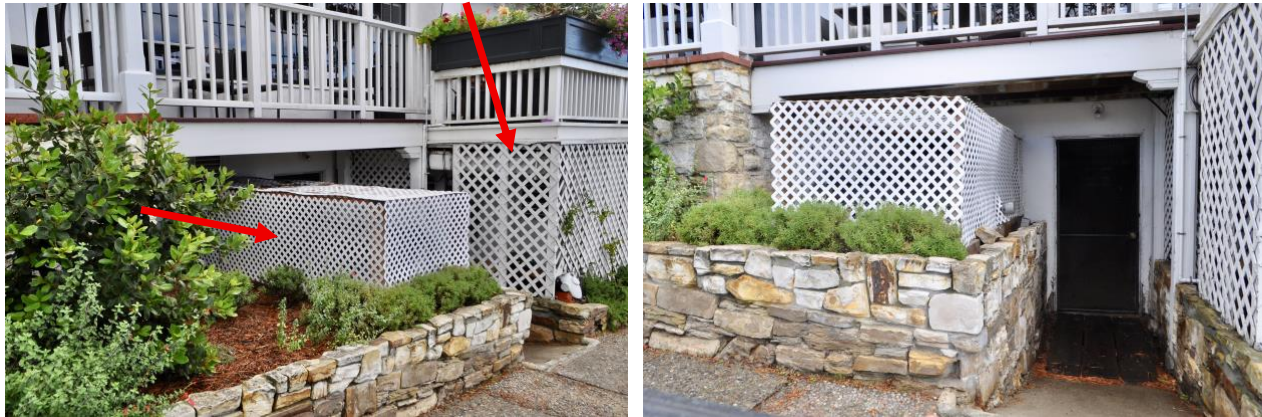
Figures 3 and 4. Left image looks south down the Monte Verde St. sidewalk at the existing locations of the fire sprinkler infrastructure. Left arrow shows a plastic lattice screen added after 2002 in an effort to match the wood lattice screen installed during the 2002 Thodos remodeling campaign (right arrow). Right image views the lower utility room entrance and the two areas impacted.
