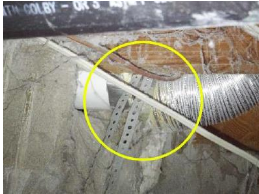
Crawlspace to be rehabilitated: install sill plate anchors and repair raised piers.
