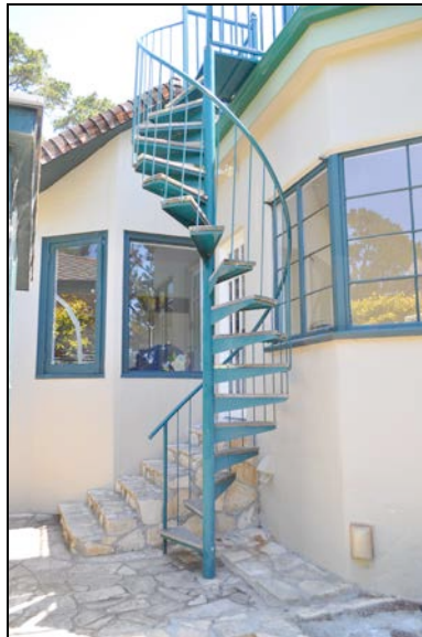
Figure 4. Metal spiral staircase.
