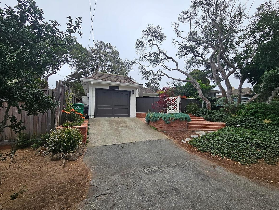
Figure 1: View of Helen Leslie House from Carmelo Street.
