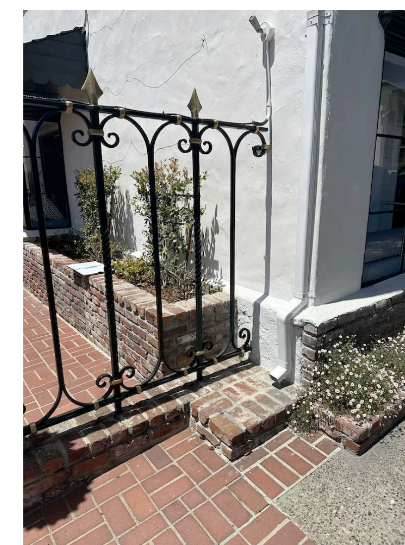
Proposed Location of New Free Standing Fire Department Connection in Front of Existing Wrought Iron Fencing
