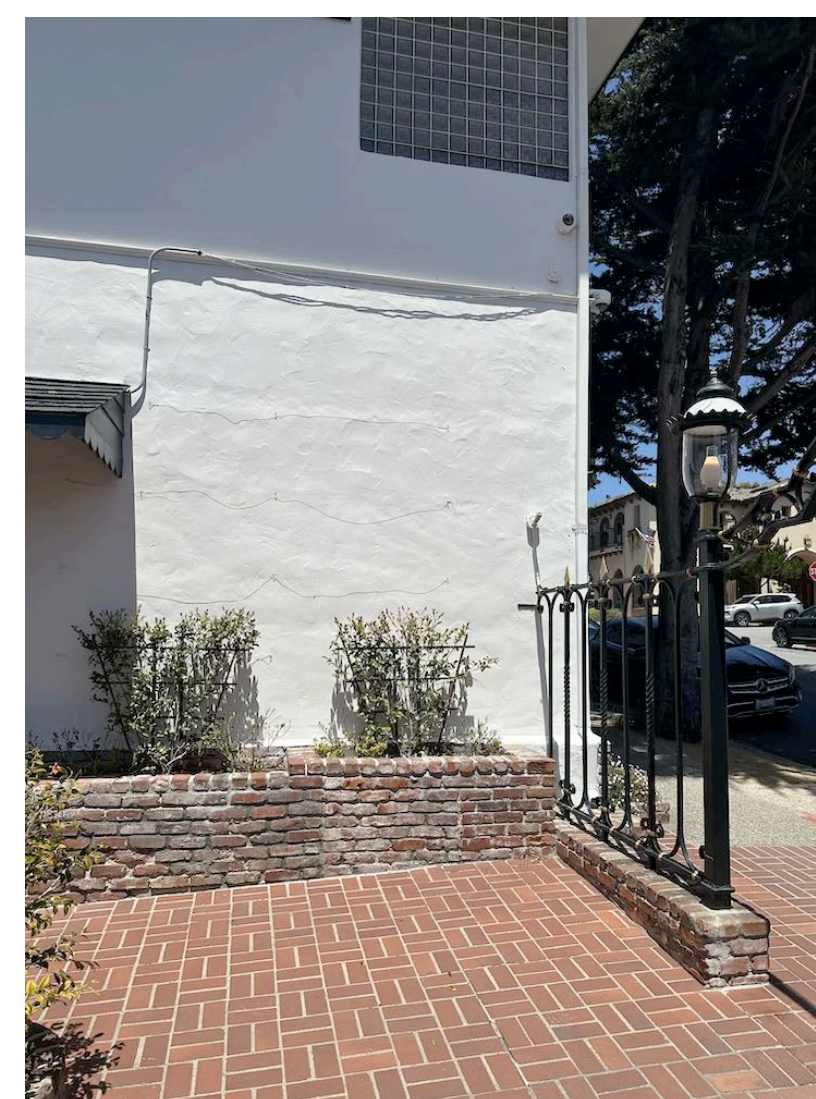
Proposed Location for New Planting Bed for New Reduced Pressure Backflow Device
