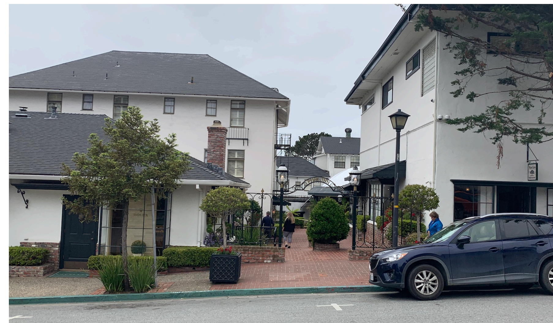
Existing Courtyard Entrance on Lincoln Street
