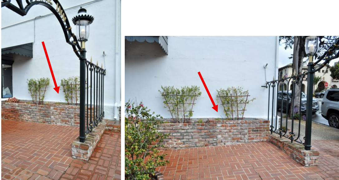
Figures 5 and 6. Left image shows the Lincoln St. entrance and the location of the proposed utility box to house the fire sprinkler risers (arrow). Right image shows the brick planter and proposed location.
