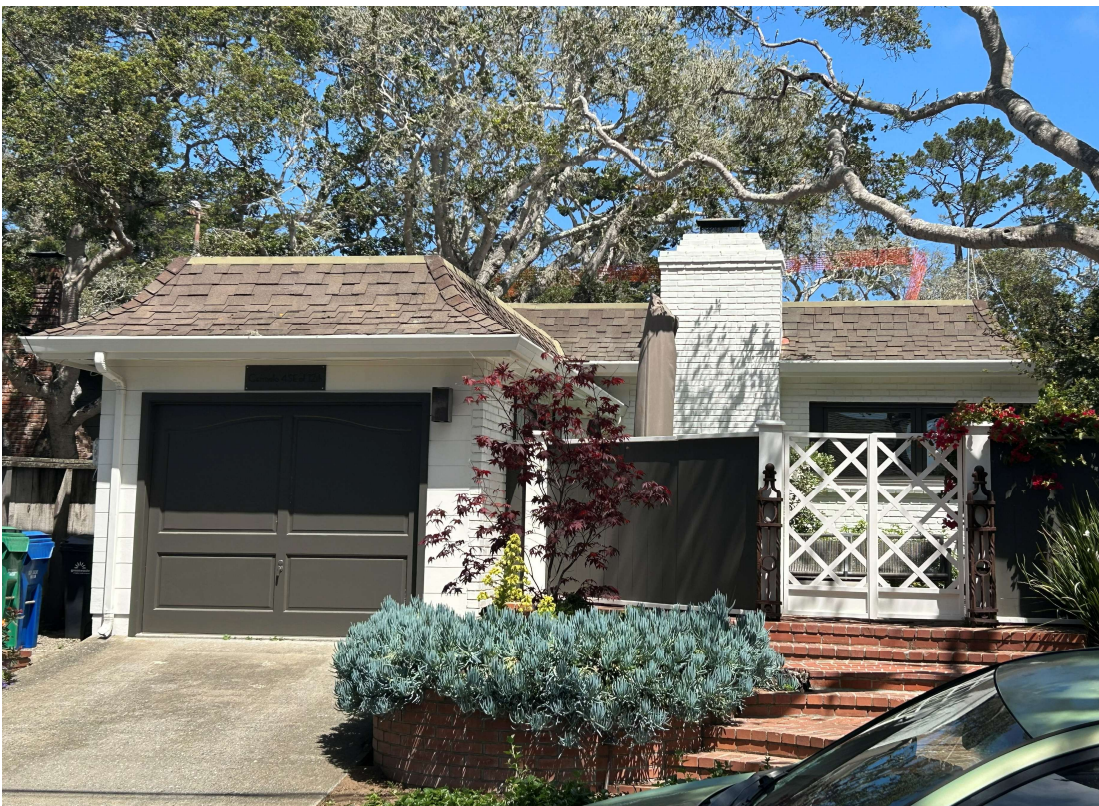
View of west elevation from Carmelo Street, view looking east.
