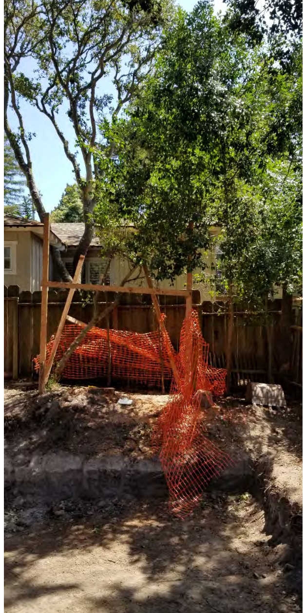
Figure 6: Small Privet trees seen looking east.
