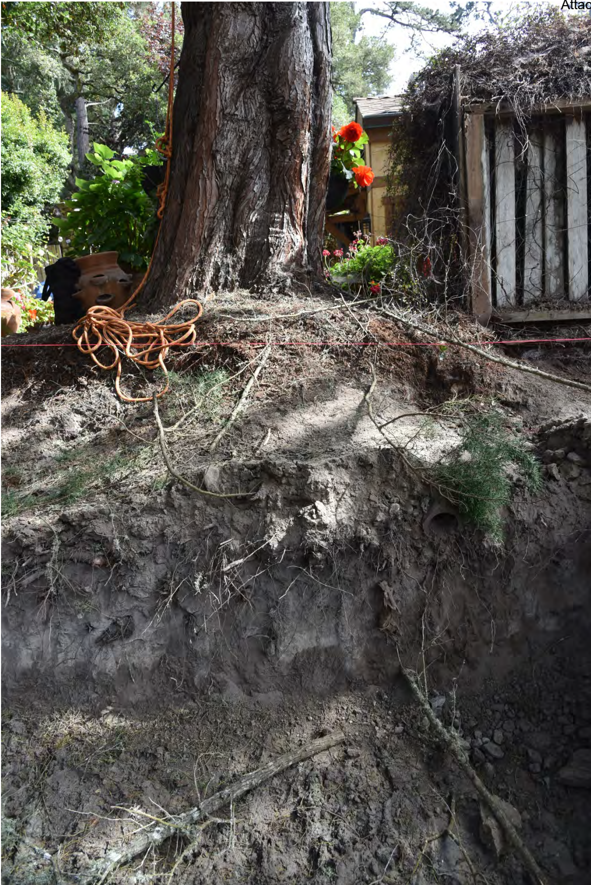
Grading around “Cypress tree #1”
