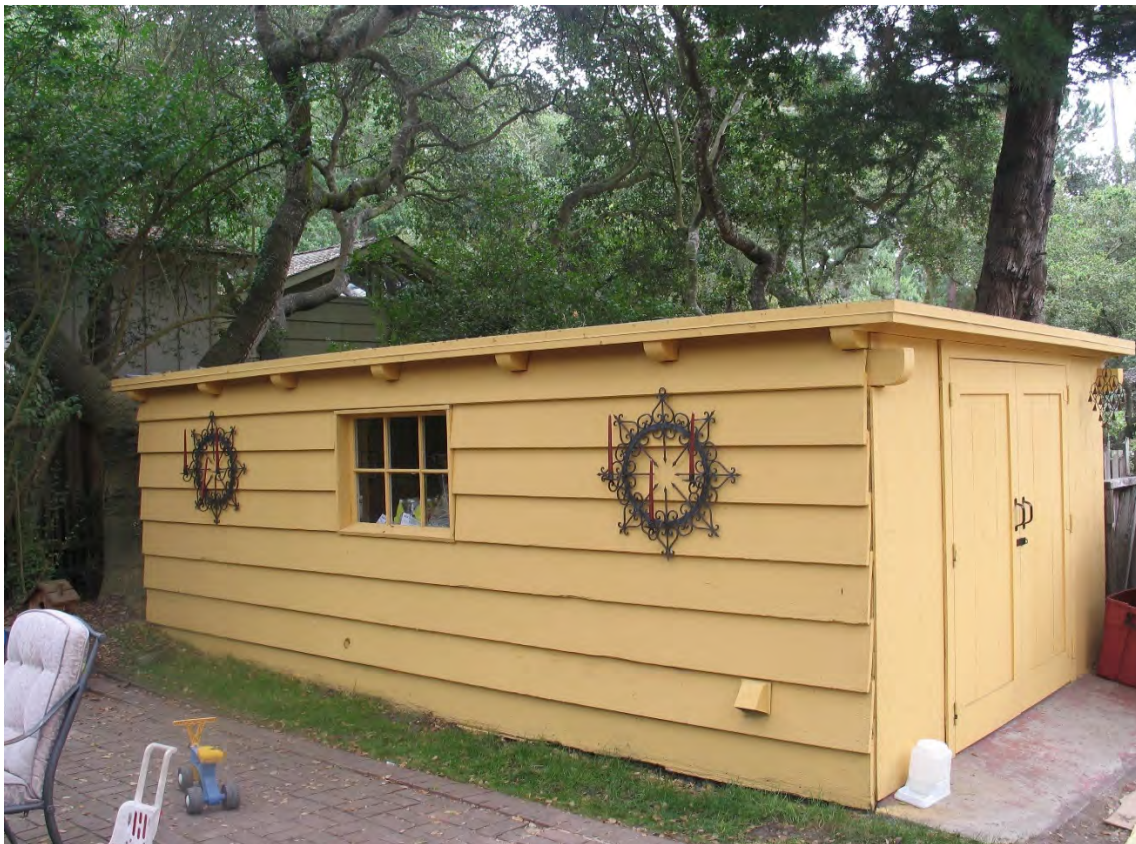
Pre-existing structure adjacent tree
