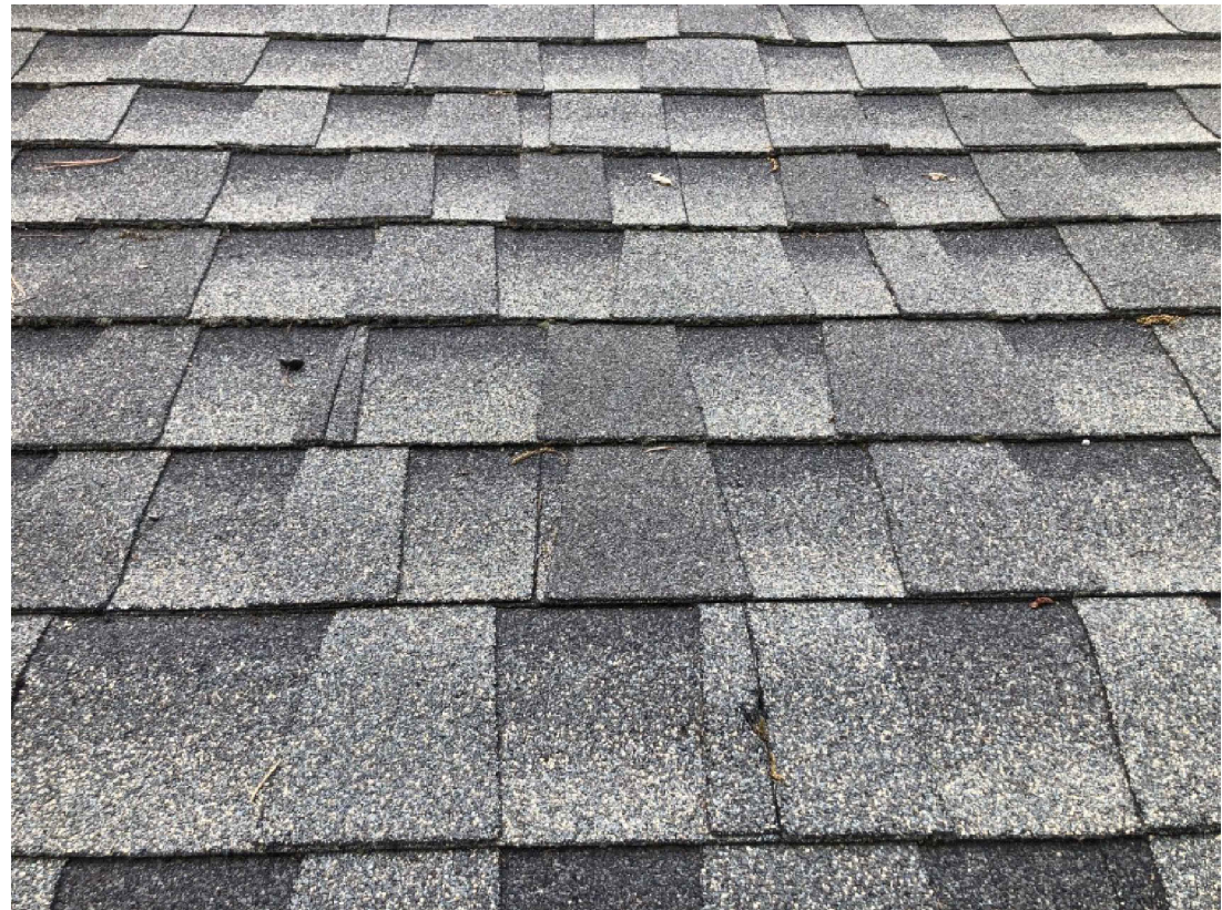
Existing and New Roofing Asphalt Composition Shingle
