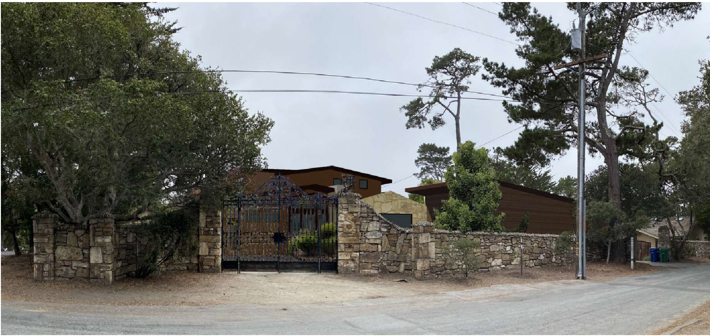
FRONT VIEW AFTER
