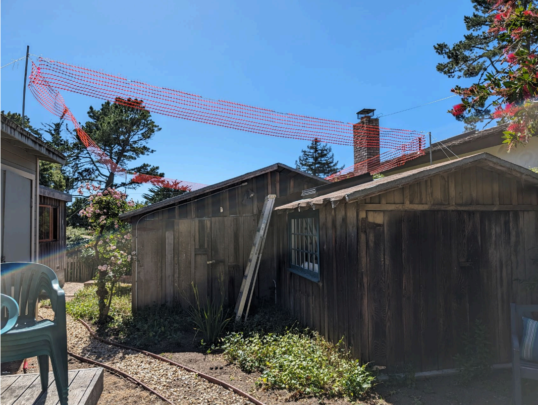
Art studio demolished in 2025, view looking west. Storypole flags are outdated.
