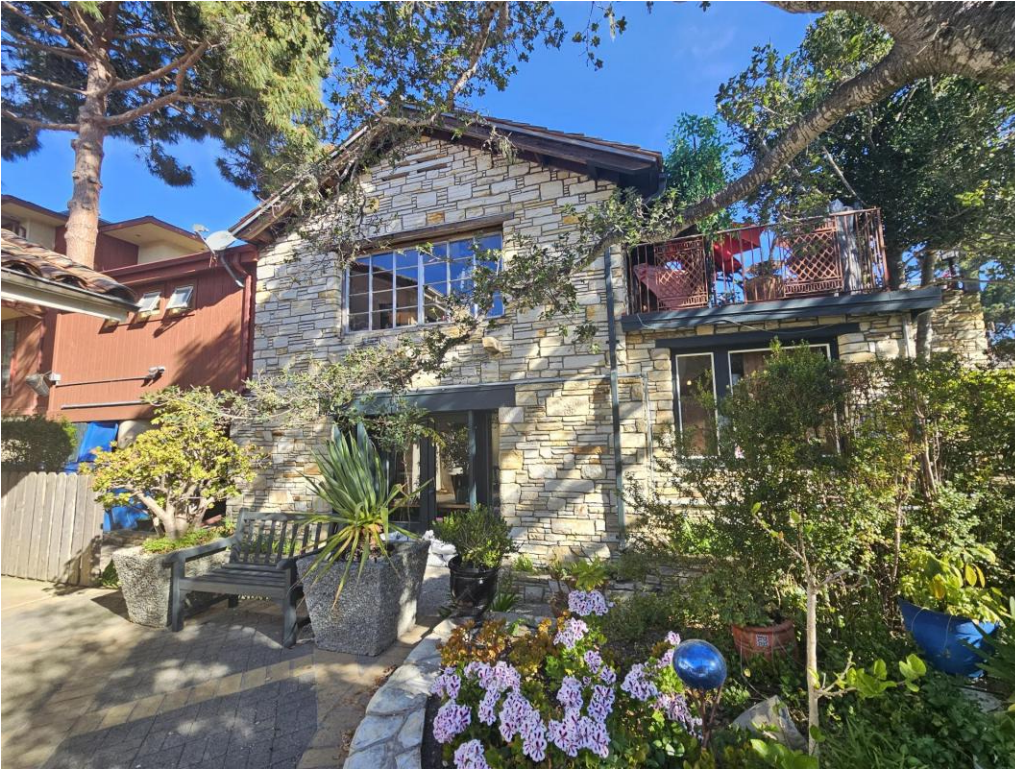
Figure 12: View of cottage south elevation, looking north from neighboring property.
