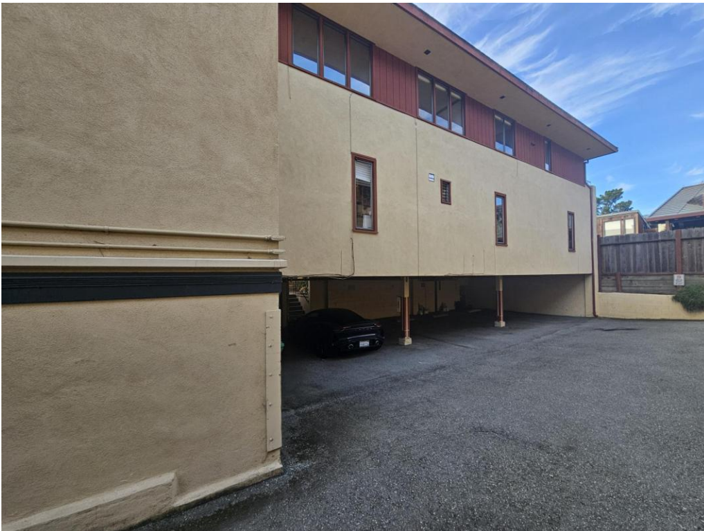
Figure 3: View of the parking garage on the north elevation, looking southwest.
