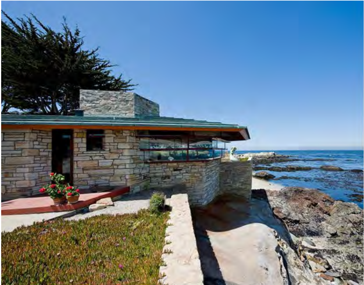
Figure 9 Circa 2010 photograph of east elevation and kitchen door and window
