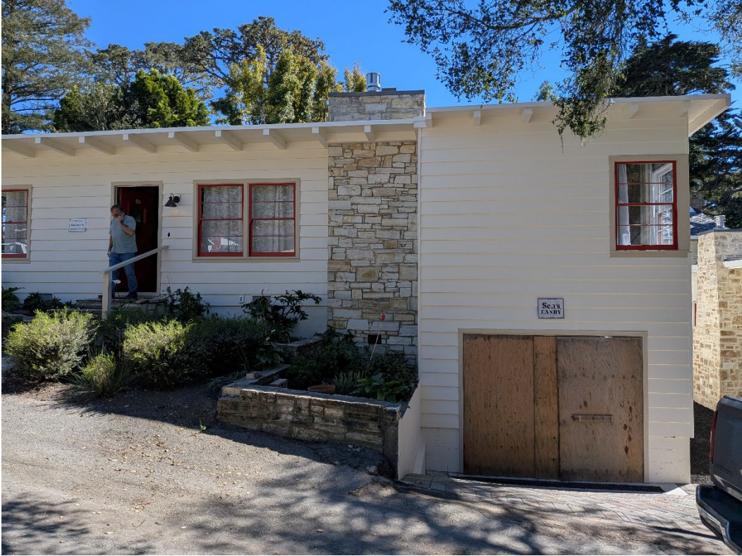
Current condition, with re-graded driveway, dropped garage floor grade, and increased garage door opening dimensions completed.
