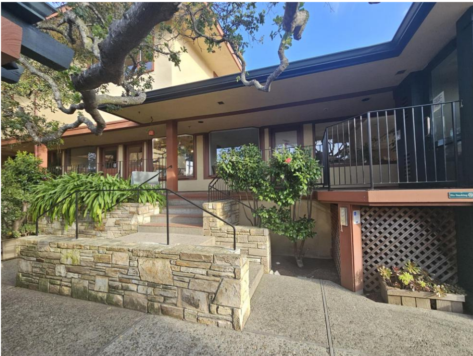
Figure 1: View of the mid-level retail space, looking north. The chalk rock hardscape in the foreground and walkway railings were installed in 2012. The bump-out at image right accommodates access to the 2012 ADA lift.
