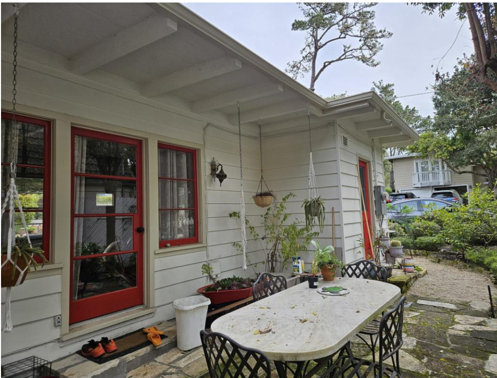
Figure 4: View of patio, south elevation.
