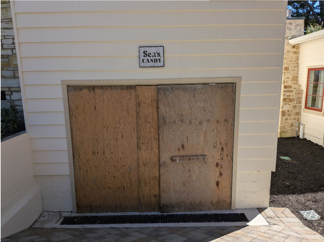
Current condition, with re-graded driveway, dropped garage floor grade, and increased garage door opening dimensions completed.
