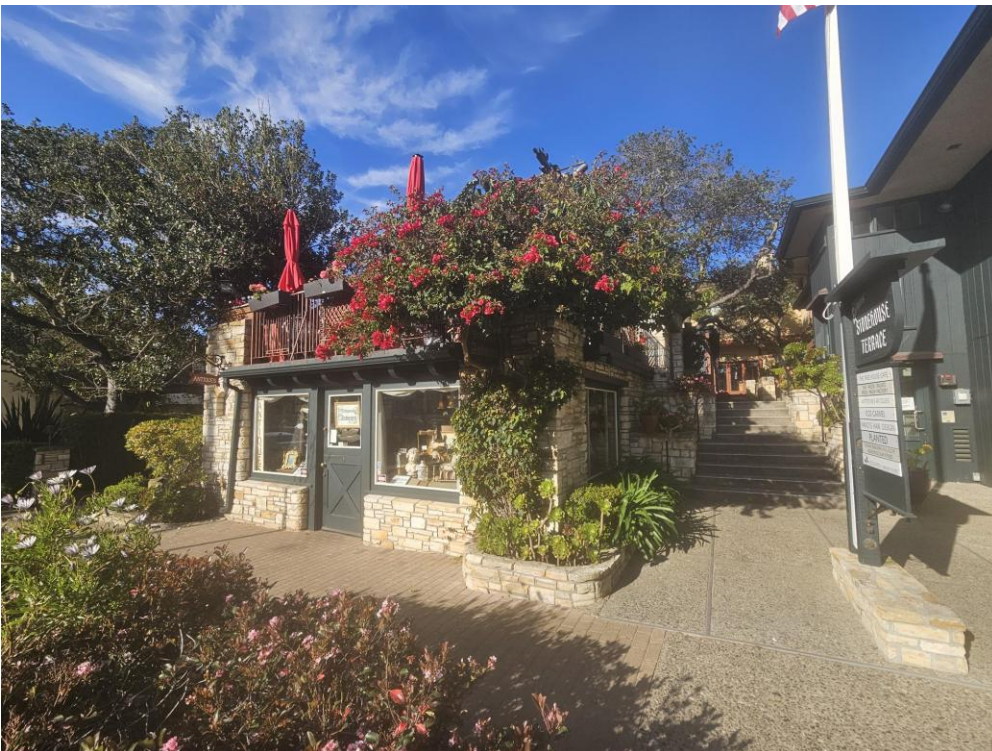
Figure 9: View of cottage east façade and north elevation, looking southwest.
