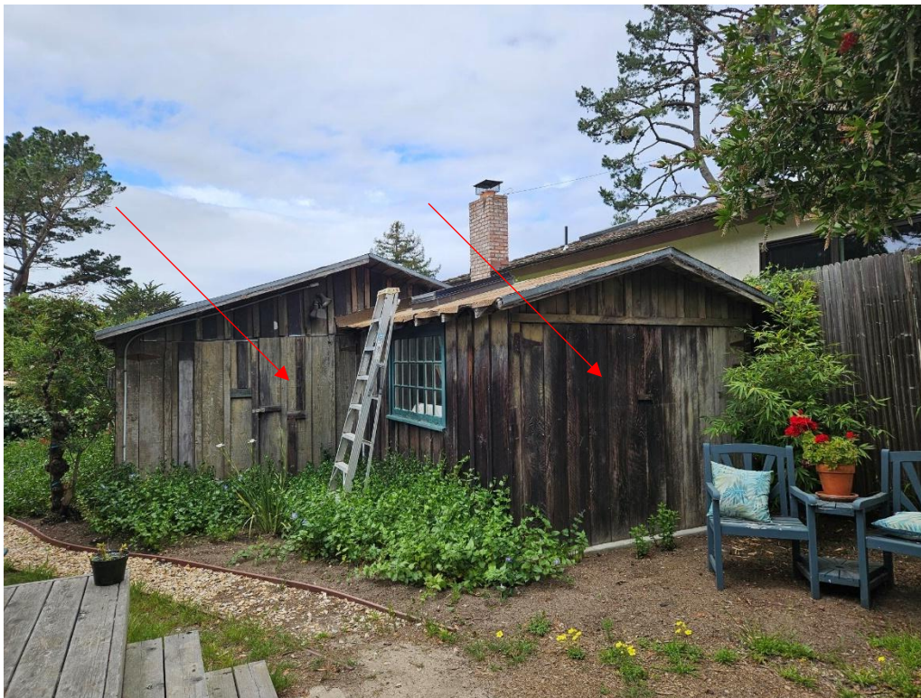
Figure 5: View of art studio looking west. Garage doors indicated by arrows.
