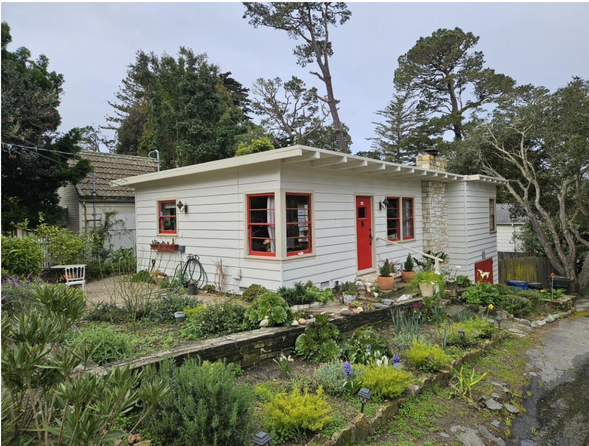
Figure 1: View of Mary Haven House looking southwest.
