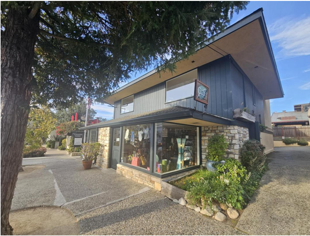
Figure 2: View of façade & partial north elevation (image right) looking southwest.
