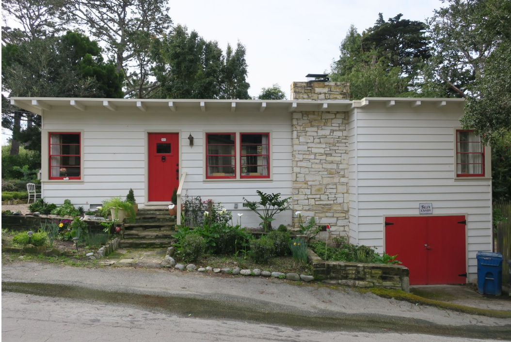
North elevation, view south. Original garage door pictured.
