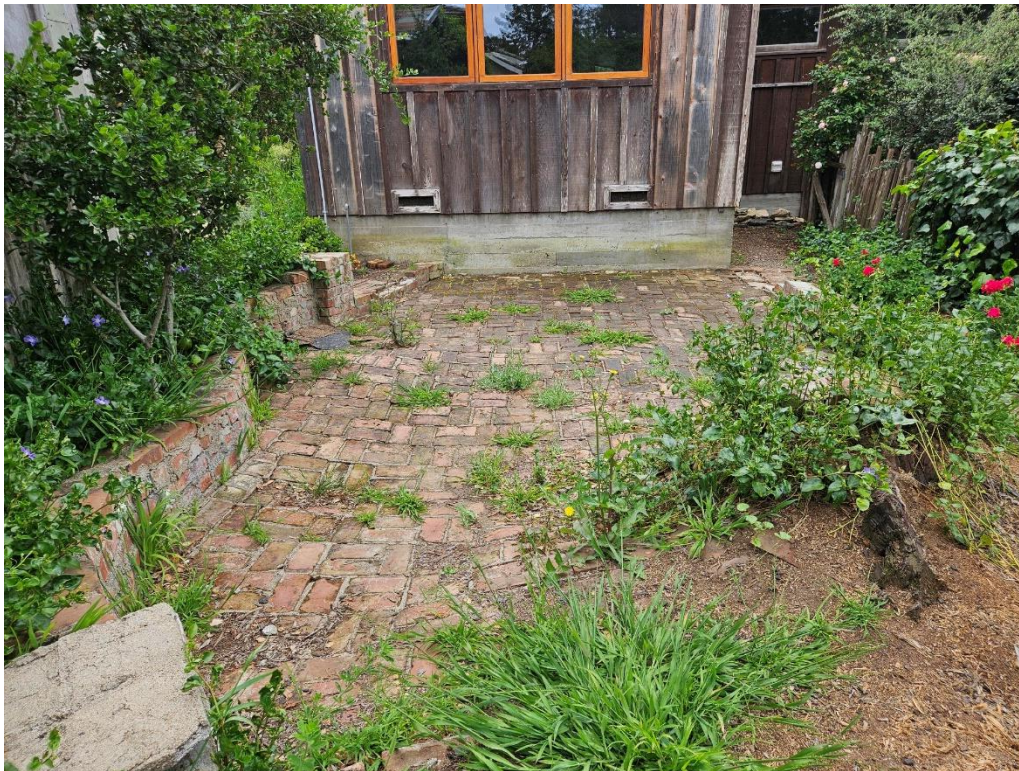
Figure 4: View of brick patio to be removed.
