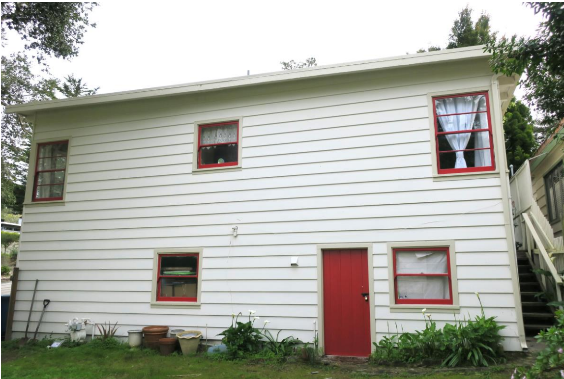
Figure 3: View of west elevation.
