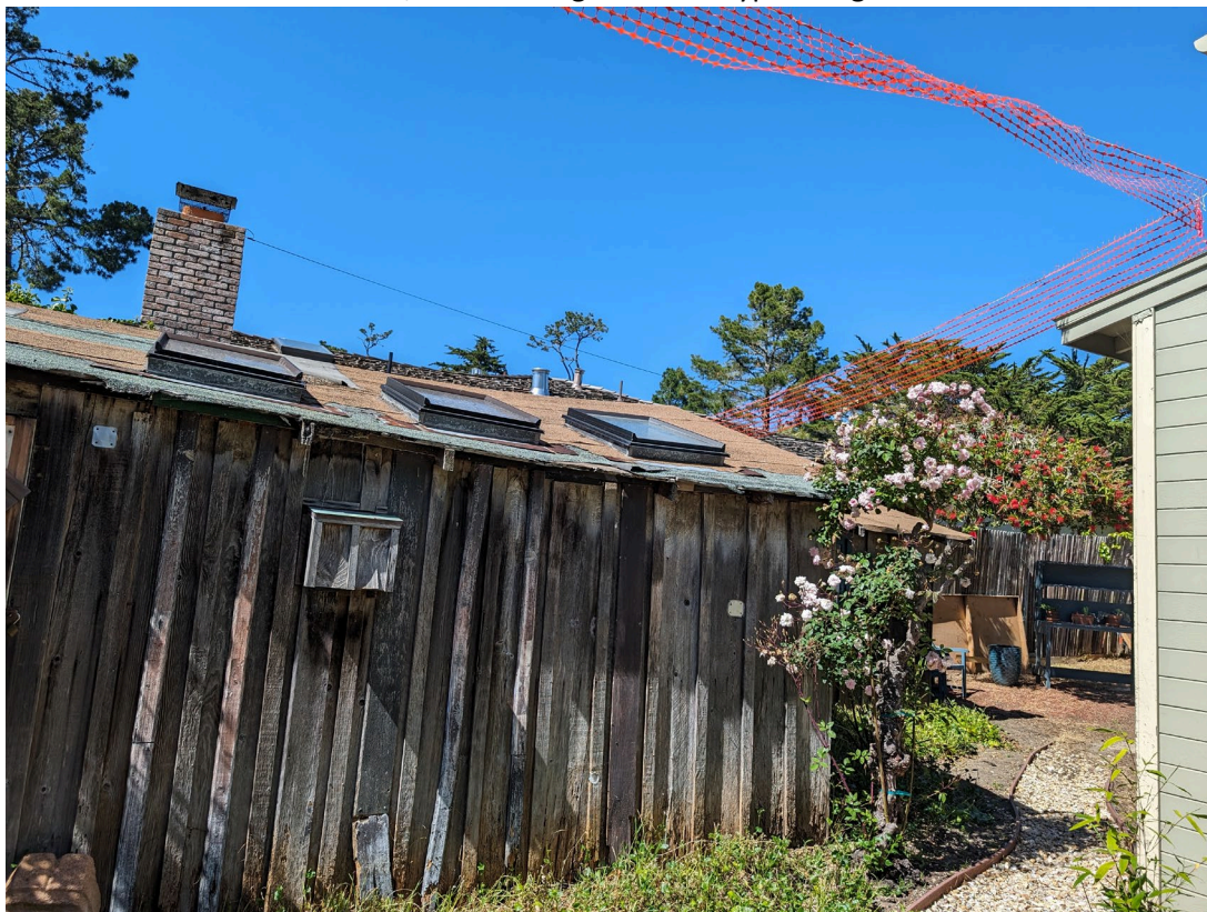
Art studio demolished in 2025, view looking northeast. Storypole flags are outdated.
