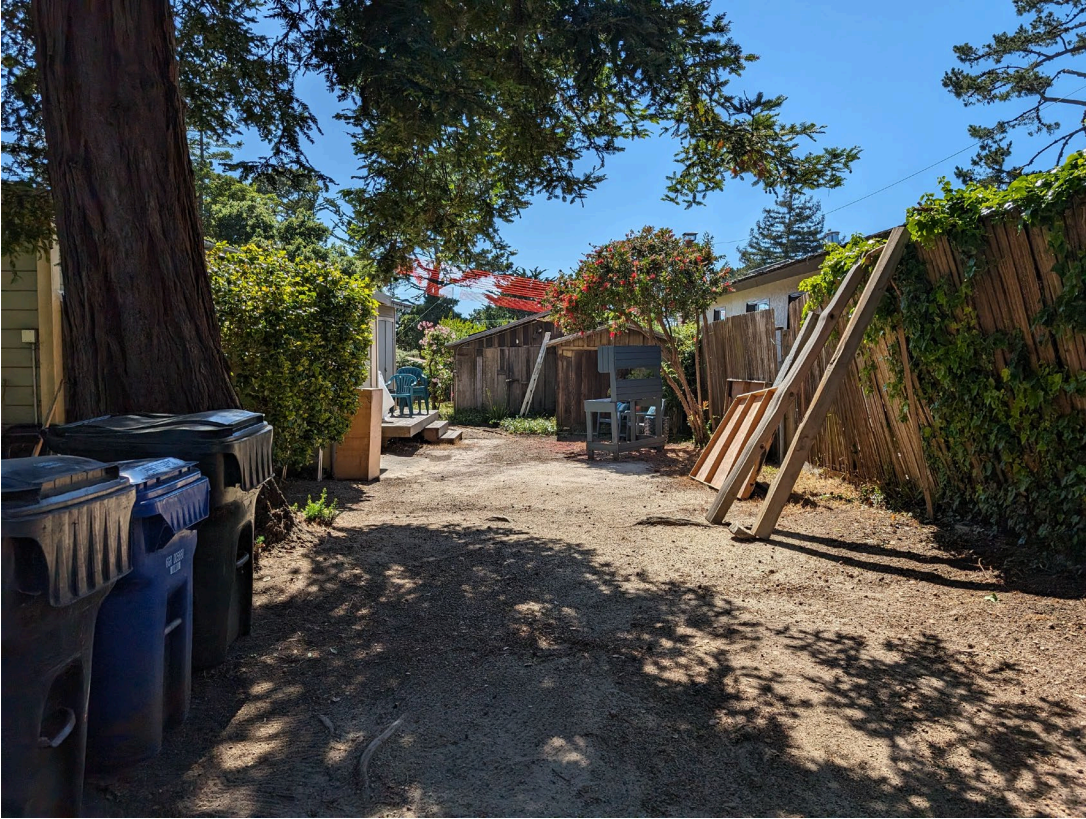
Art studio shed demolished in 2025, view looking west from Guadalupe Street. Storypole flags are outdated.
