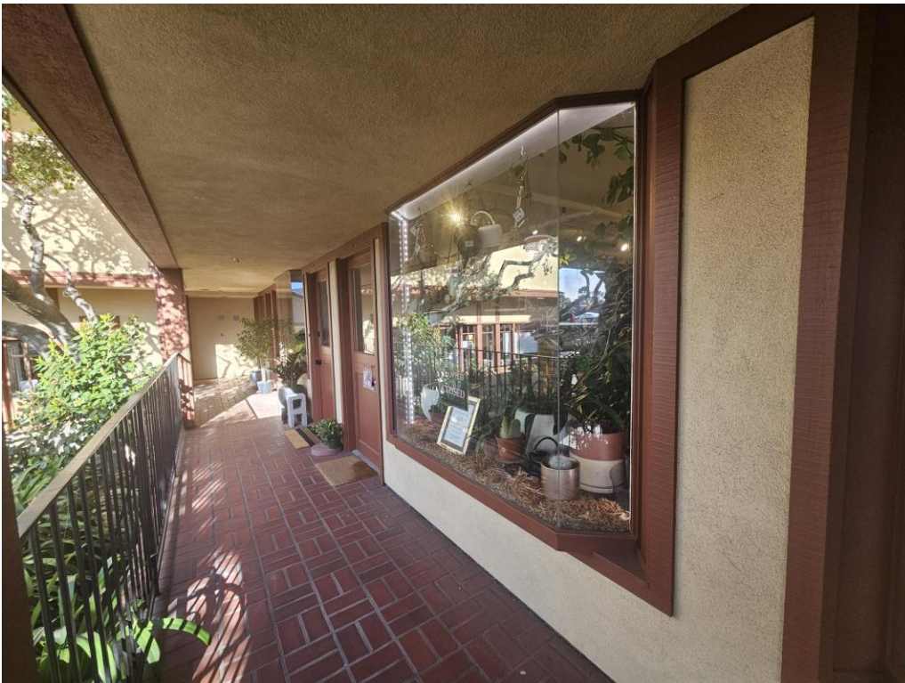
Figure 5: Looking west down mid-level retail/office walkway with bay windows.
