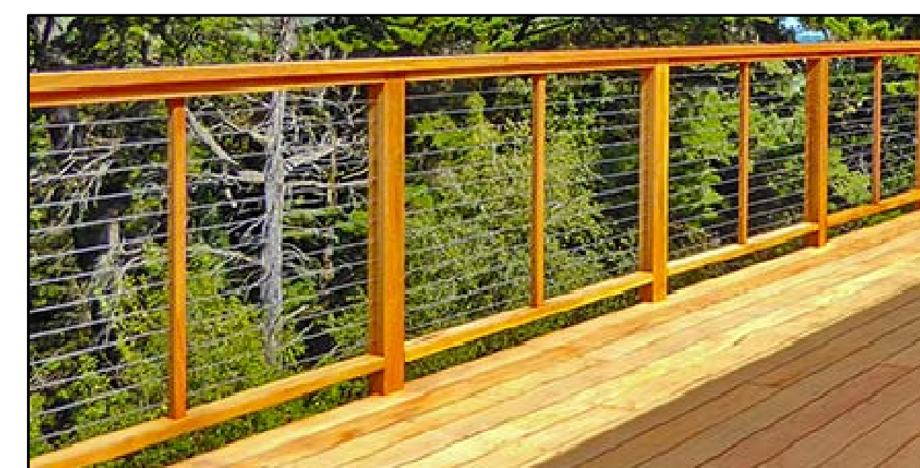
A - WOOD POSTS WITH CABLE RAILING
