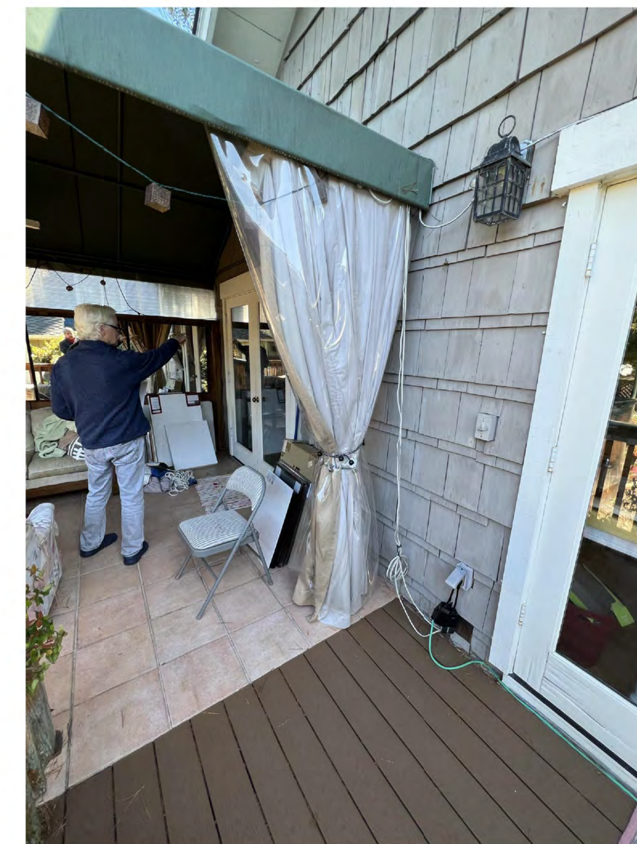
REAR FACING (WEST) VIEW OF HOME & BACK DOORS FROM DECK
