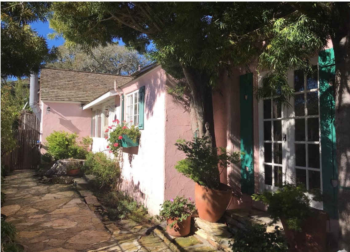
Figure 6: French doors on south elevation to remain in place. Kitchen window with shutters also to remain in place.
