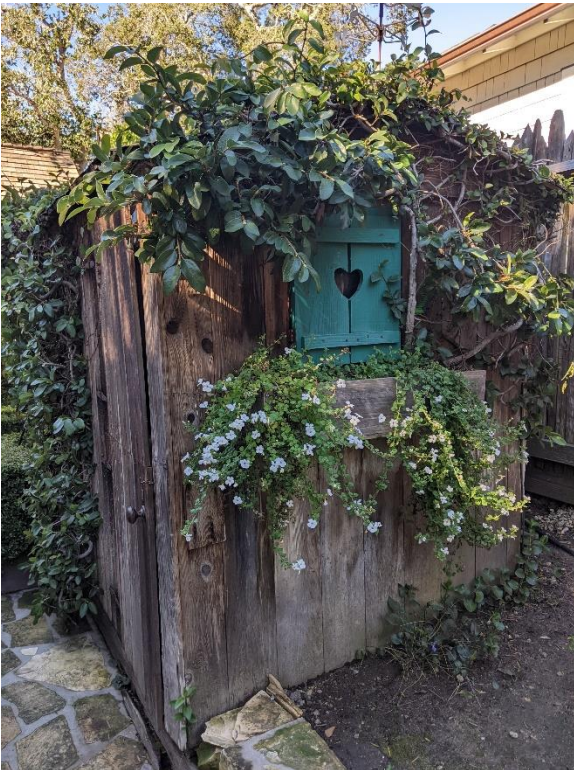
Figure 9: Non-historic shed to be demolished.
