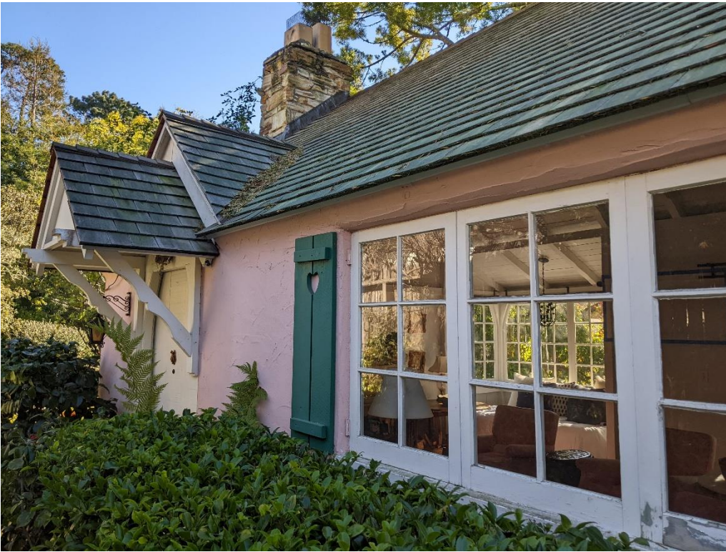
Figure 7: Entry door and bank of three windows to remain in place.
