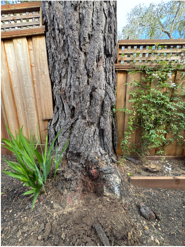
Inspection of the root collar south side revealed areas of compressed wood development, indicating long-term mechanical stress at the base of the trunk.
