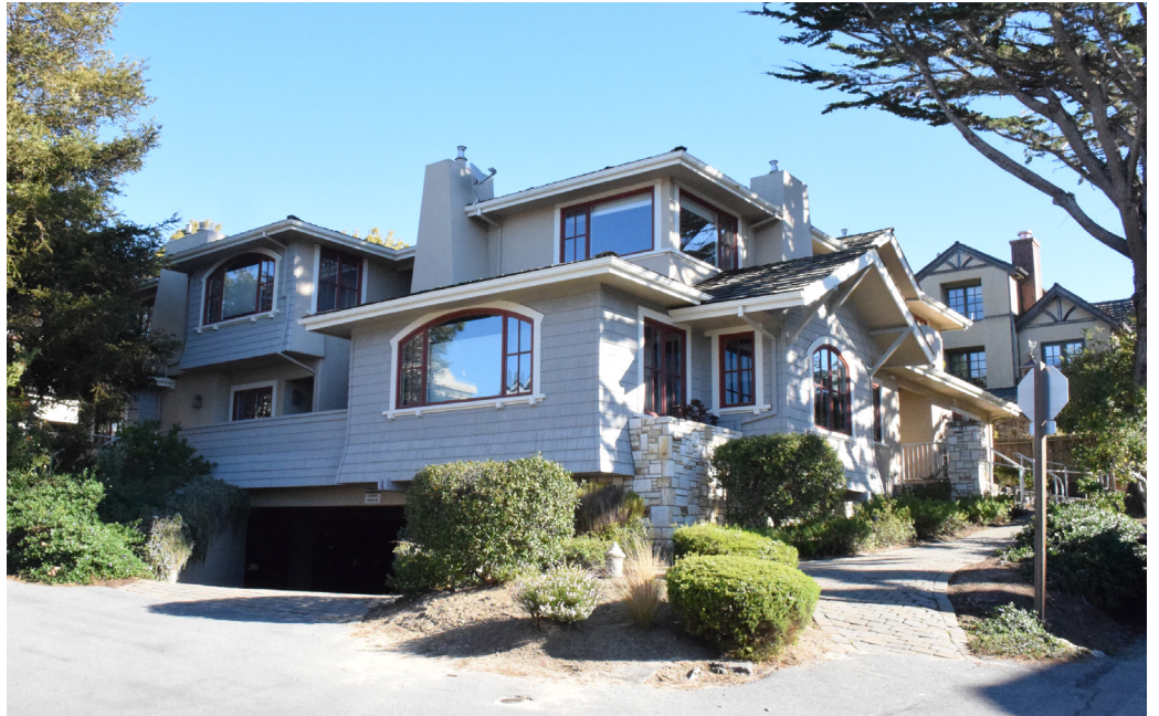
NE Corner of Mission St and 4th Ave
