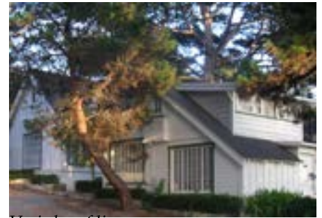
Varied roof lines
