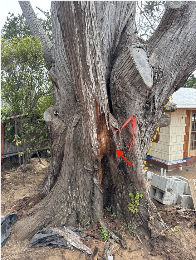
Advanced decay is present in multiple areas of the trunk, as confirmed through probing, sounding, and removal of loose bark, further reducing structural integrity.
