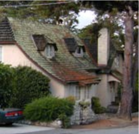
Low eave lines and dormers that are subordinate to the roof plane are typical features.
