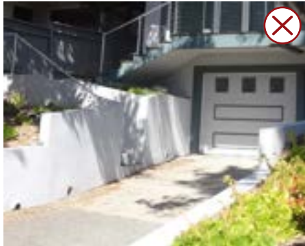
Large exposed retaining wall
