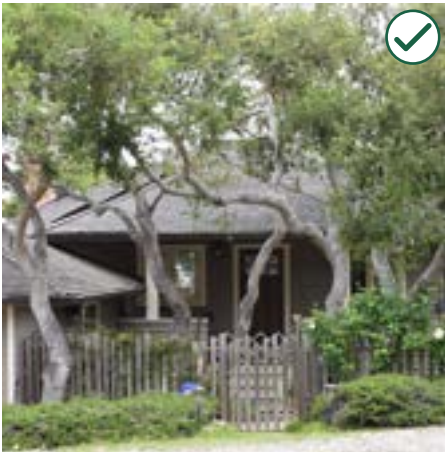
A building shall be designed to be subordinate to the forest character.
