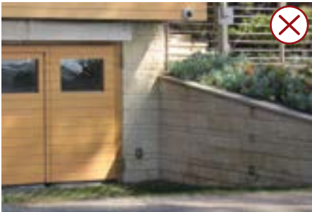
Large exposed retaining wall
