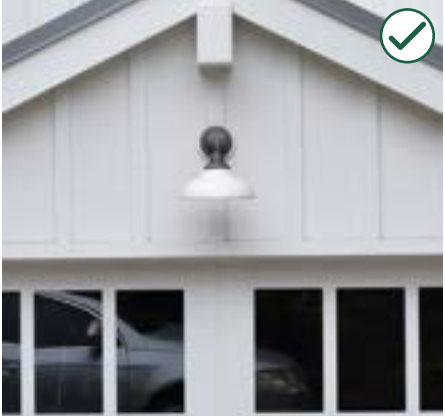
Locate and shield fixtures to avoid glare.
