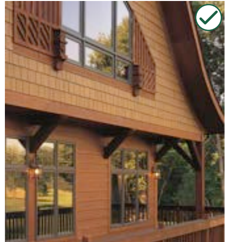
Fiber cement siding that appears similar to traditional wood may be used.
