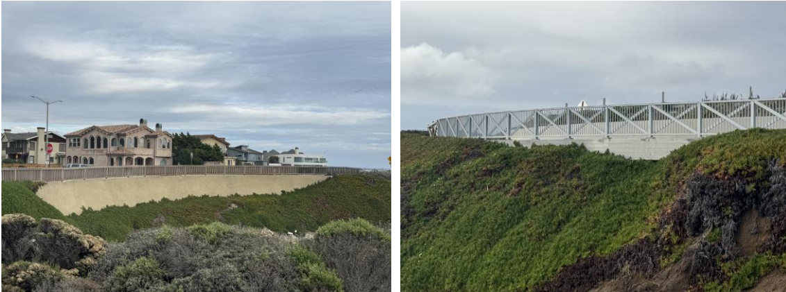
Figure 26. Armored Pathway Along West Cliff Drive in Santa Cruz, California.
