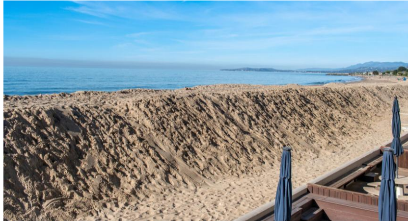
Figure 6. Winter Storm Berm at Carpinteria City Beach Protecting a Low-Lying Neighborhood
