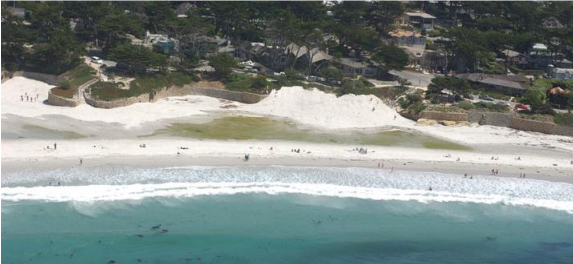
Figure 13. Sand Management with Sand Bulldozed over Riprap Revetments near 13th Avenue (Kenneth & Gabrielle Adelman, Coastal Records Project 2003)
