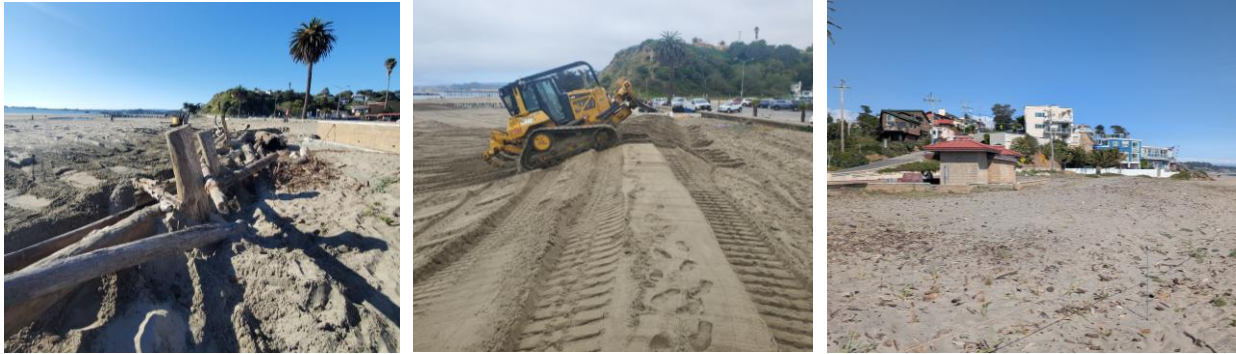
Figure 8. Rio del Mar State Beach in Aptos, California: Driftwood Logs Pinned Vertically and Cross-Braced to Form the Core of a New Dune Site (left); Sand Placed over the Logs (center); Post-Construction with Dune Vegetation Establishment (right)
